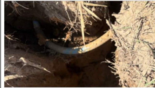
TEST HOLE PHOTO OF UTILITY DATE: 9/4/2025
