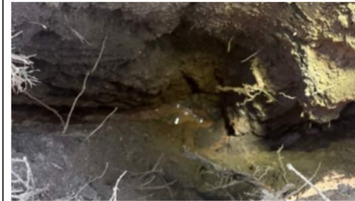
TEST HOLE PHOTO OF UTILITY DATE: 9/9/2025
