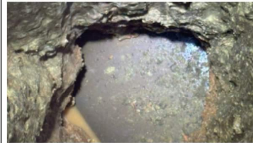
TEST HOLE PHOTO OF UTILITY DATE: 9/5/2025
