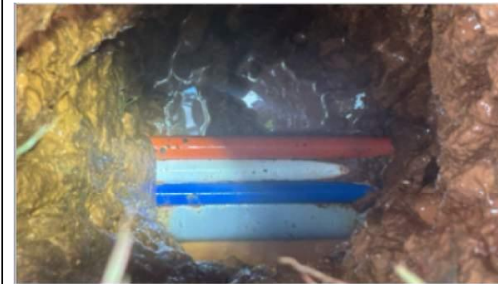
TEST HOLE PHOTO OF UTILITY DATE: 9/3/2025
