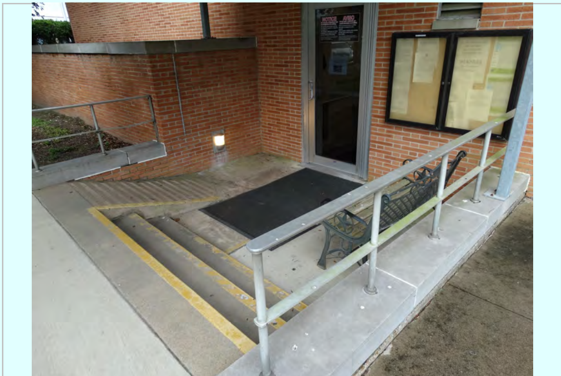
Photo: Non-compliant entry ramp, no handrails, non-compliant door, only existing ramp entry
