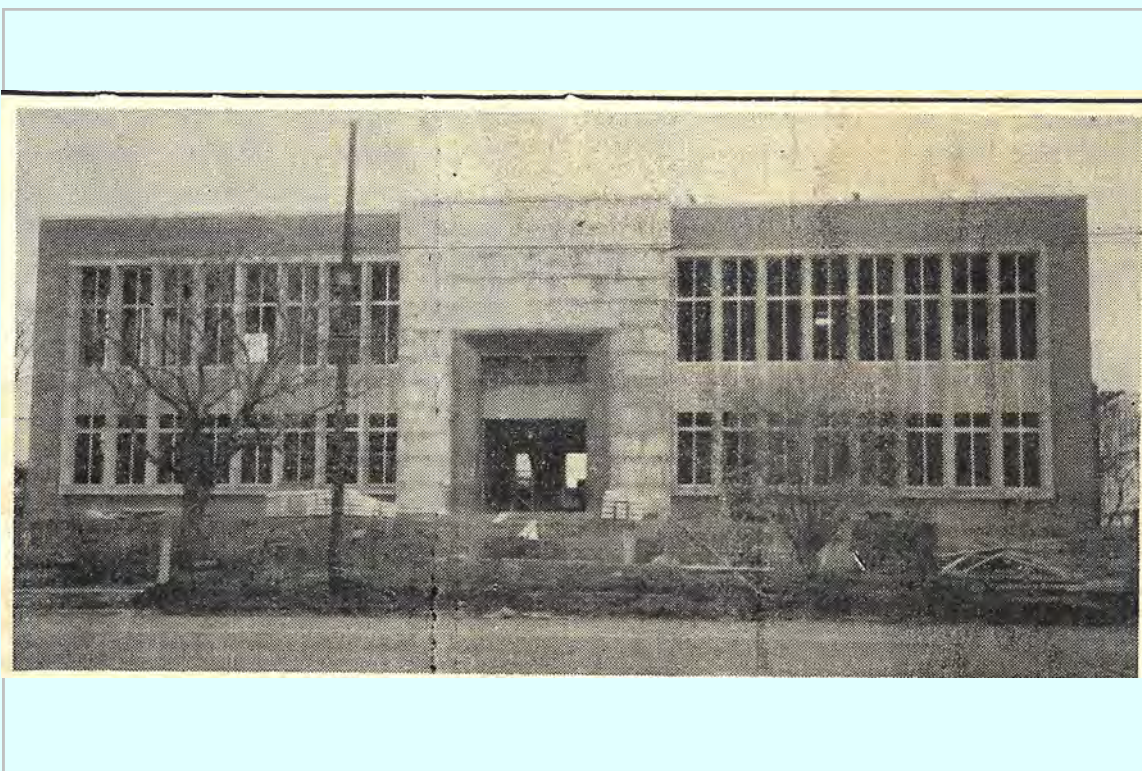
Photo: Photo of 1955 courthouse in construction, circa March 1955
