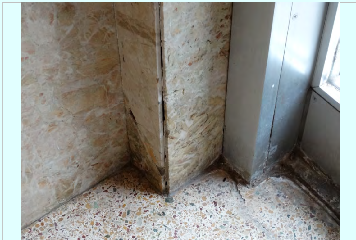
Photo: Typical stone condition at outside corner at north curtain wall
