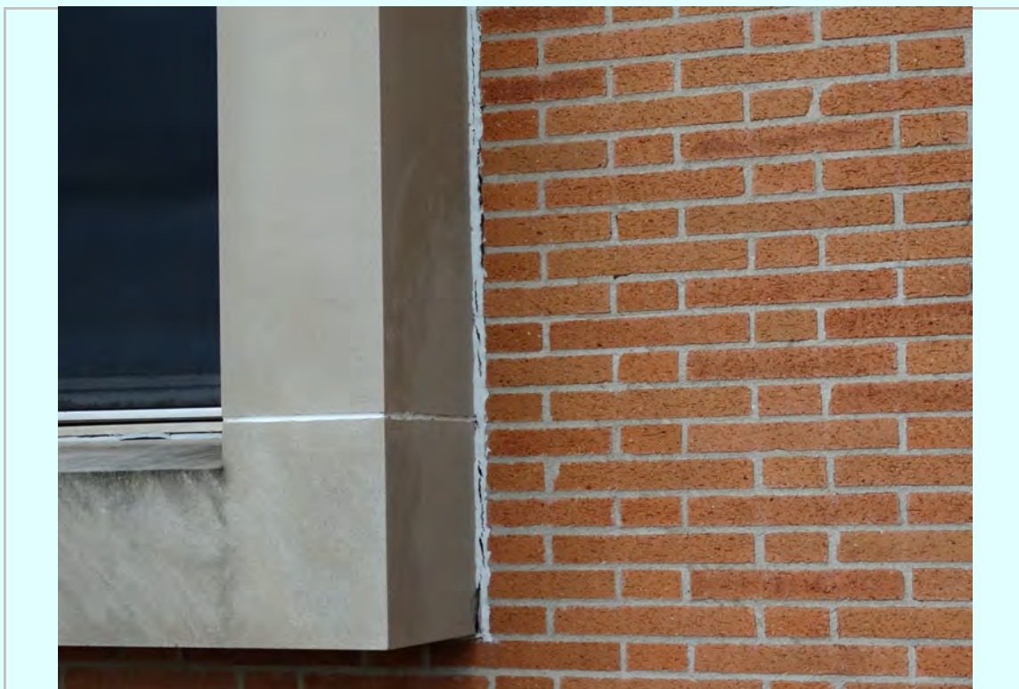
Photo: South Elevation, masonry juncture failing, replacement sealant failing
