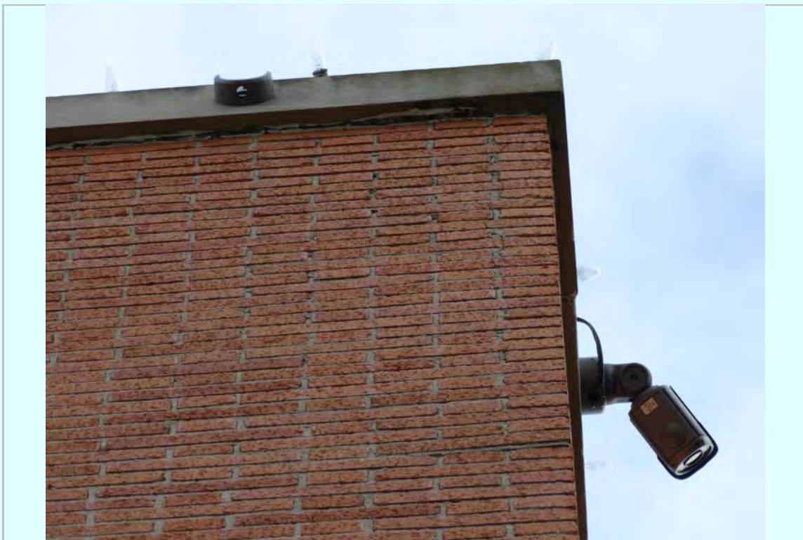
Photo: South Elevation, masonry mortar failing
