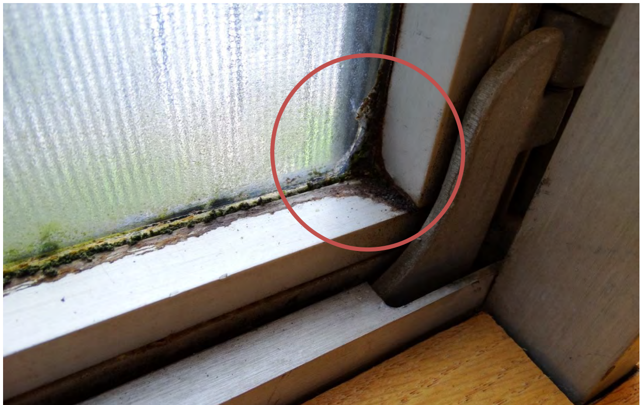
Figure 31. Biological growth occurring at window lower sash, typical.
