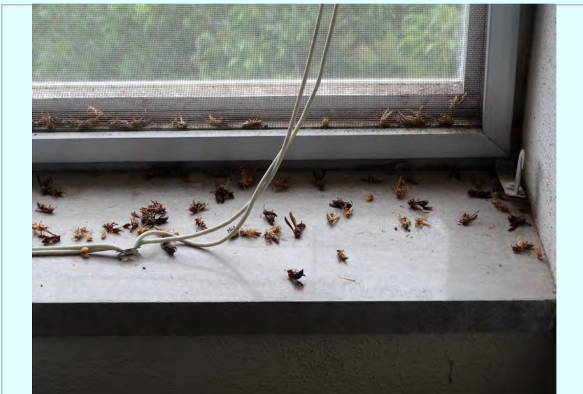
Photo: 4th floor existing window failure and insect infestation
