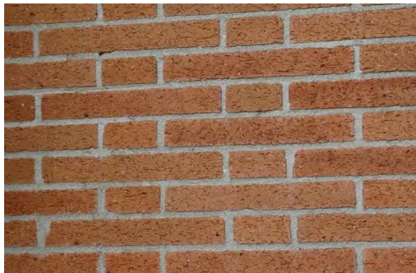
Figure 21. Typical face brick masonry
