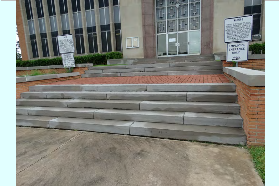
Photo: South entry limestone steps
