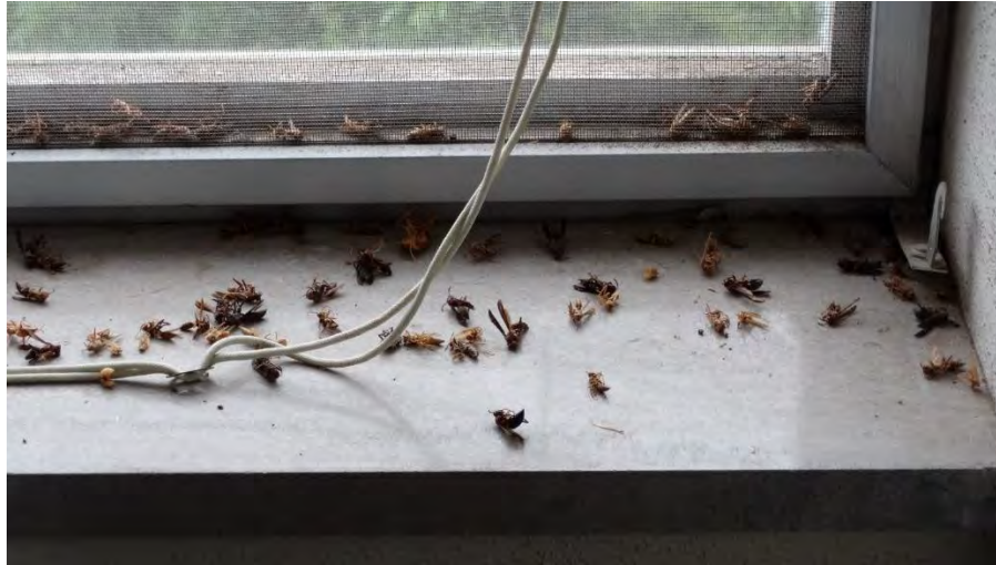
Figure 32. Wasp infestation at fourth floor windows, not active
