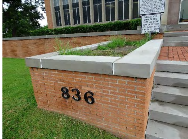
Figure 4. (Left) South walkway entrance with limestone steps and clay pavers. Figure 5. (Right) South walkway entrance masonry cheek wall with planter
