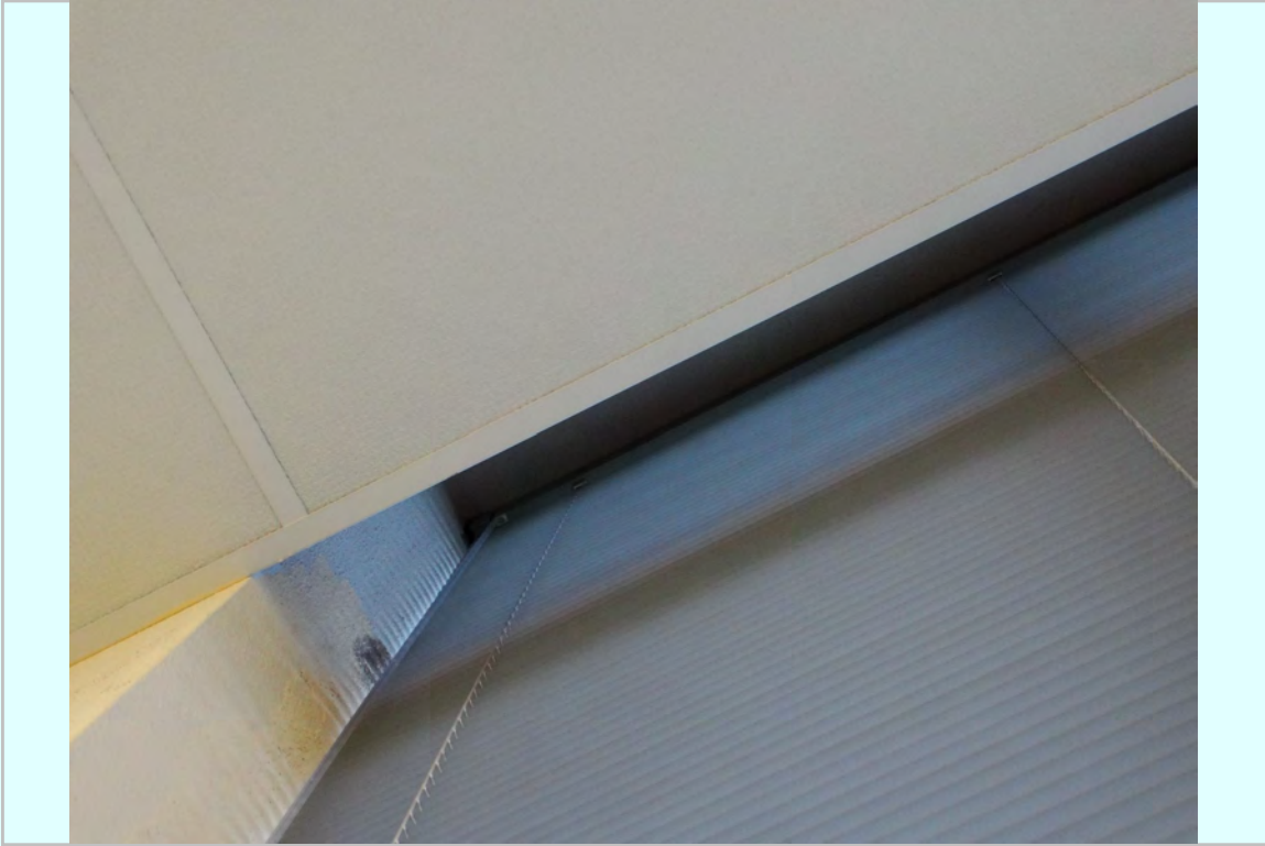
Photo: 2nd floor existing window pocket
