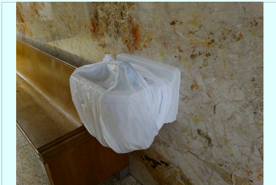
Photo: Non-compliant water fountain in public corridors.
