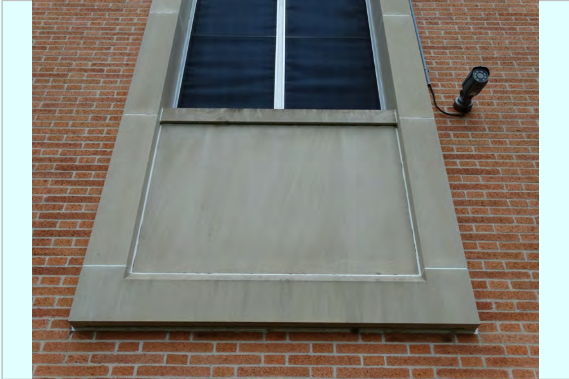
Photo: West Elevation, spandrel panel joint mortar replacement
