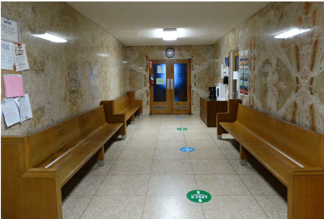
Figure 40. Existing first floor corridor
