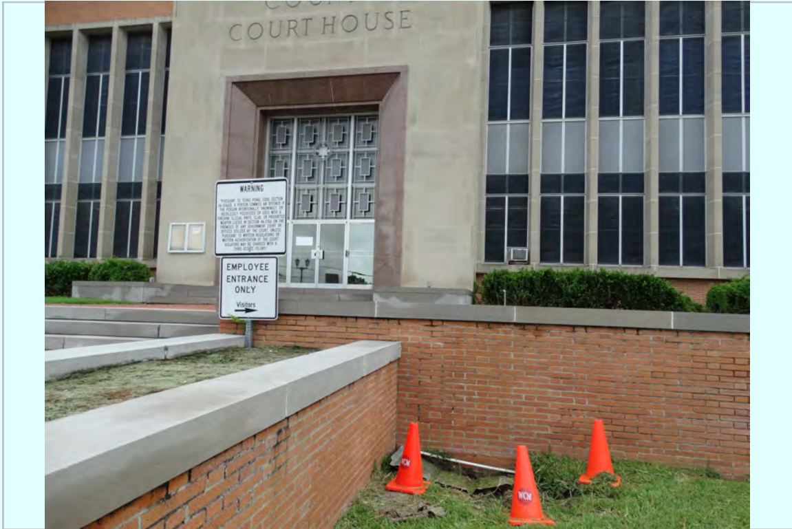
Photo: South entry East retaining wall and erosion
