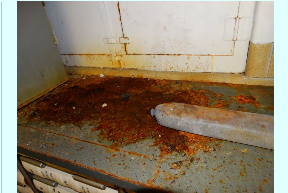
Photo: Storage space below County Clerk, rust from moisture damage
