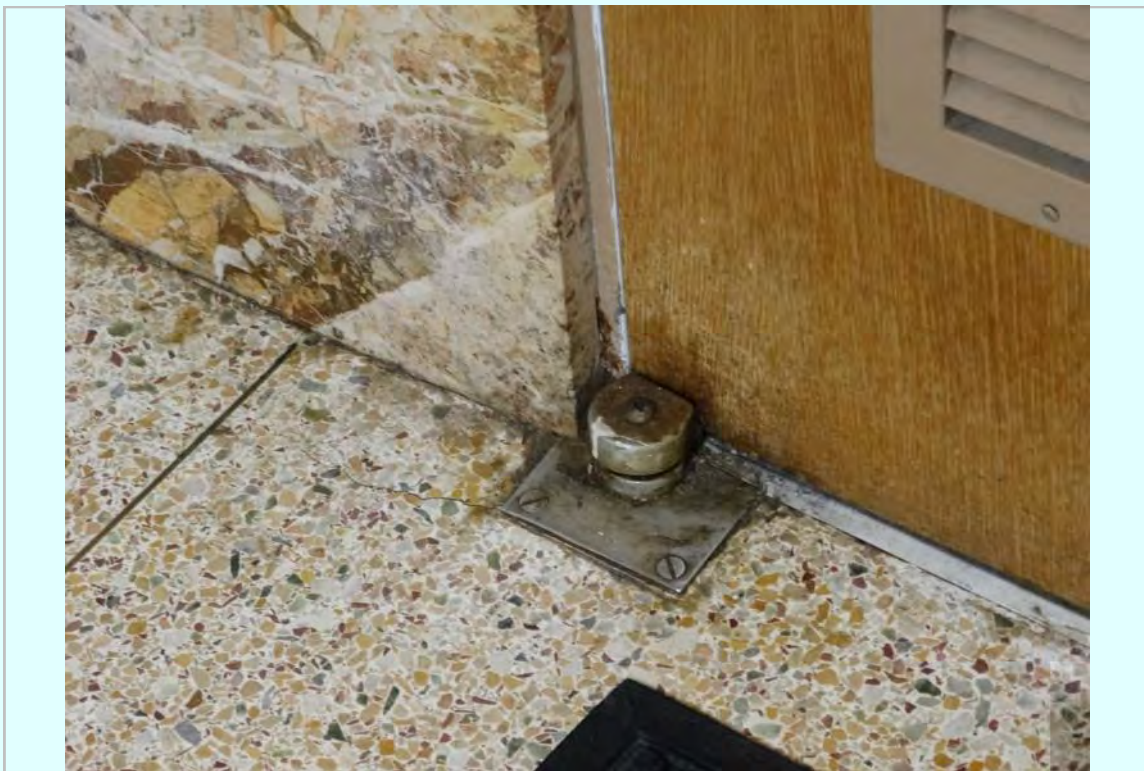
Photo: Second floor corridor door pivot hinges
