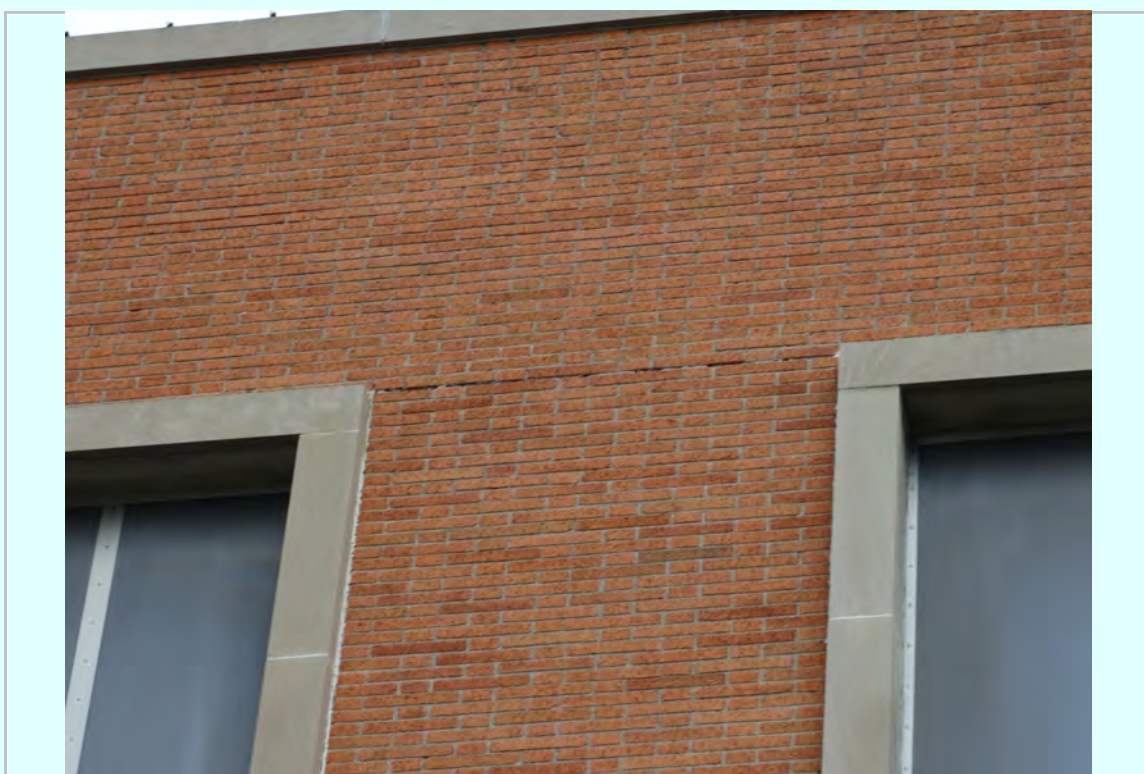
Photo: East Elevation, shelf angle joint deterioration
