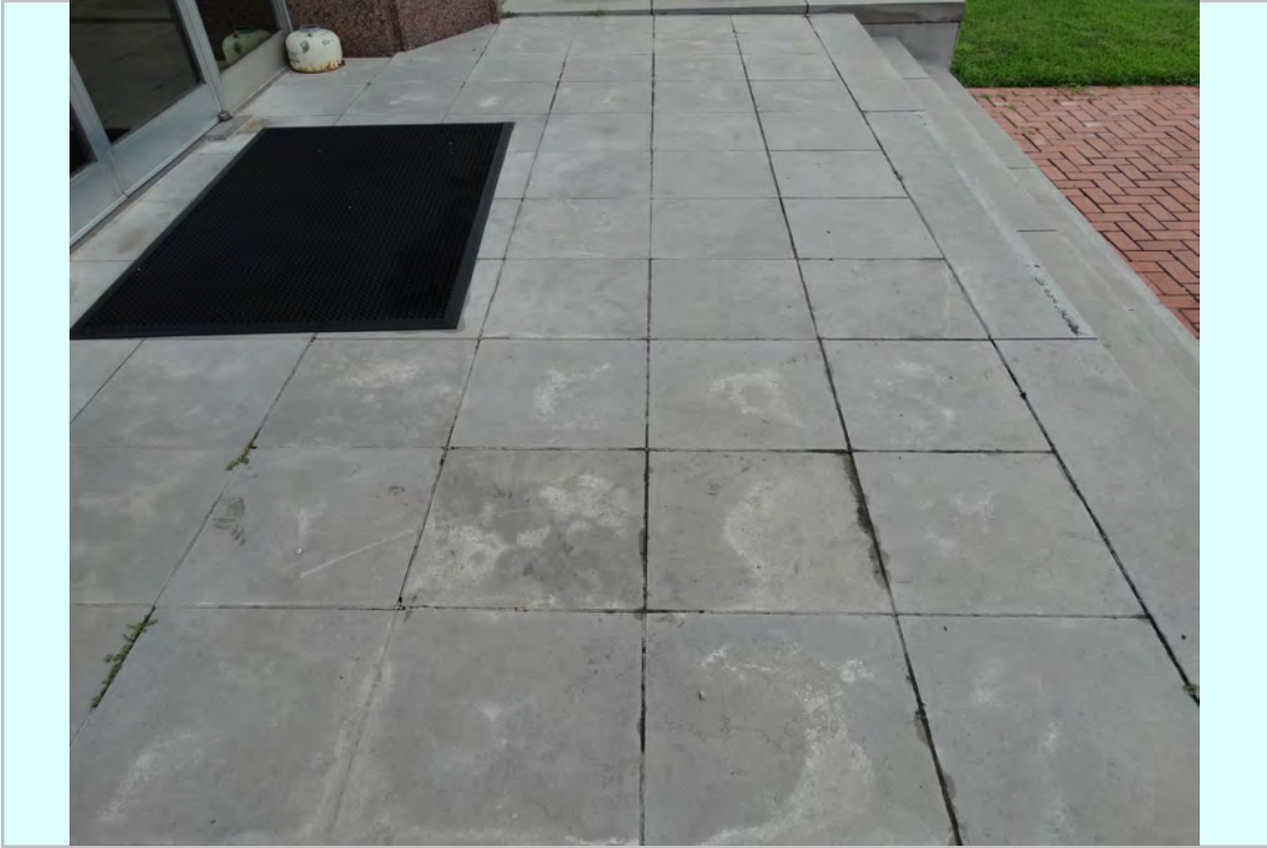
Photo: South entry patio stone paver condition
