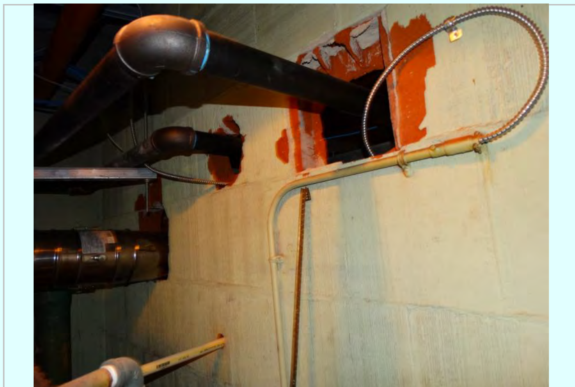
Photo: Fourth floor, mechanical space
