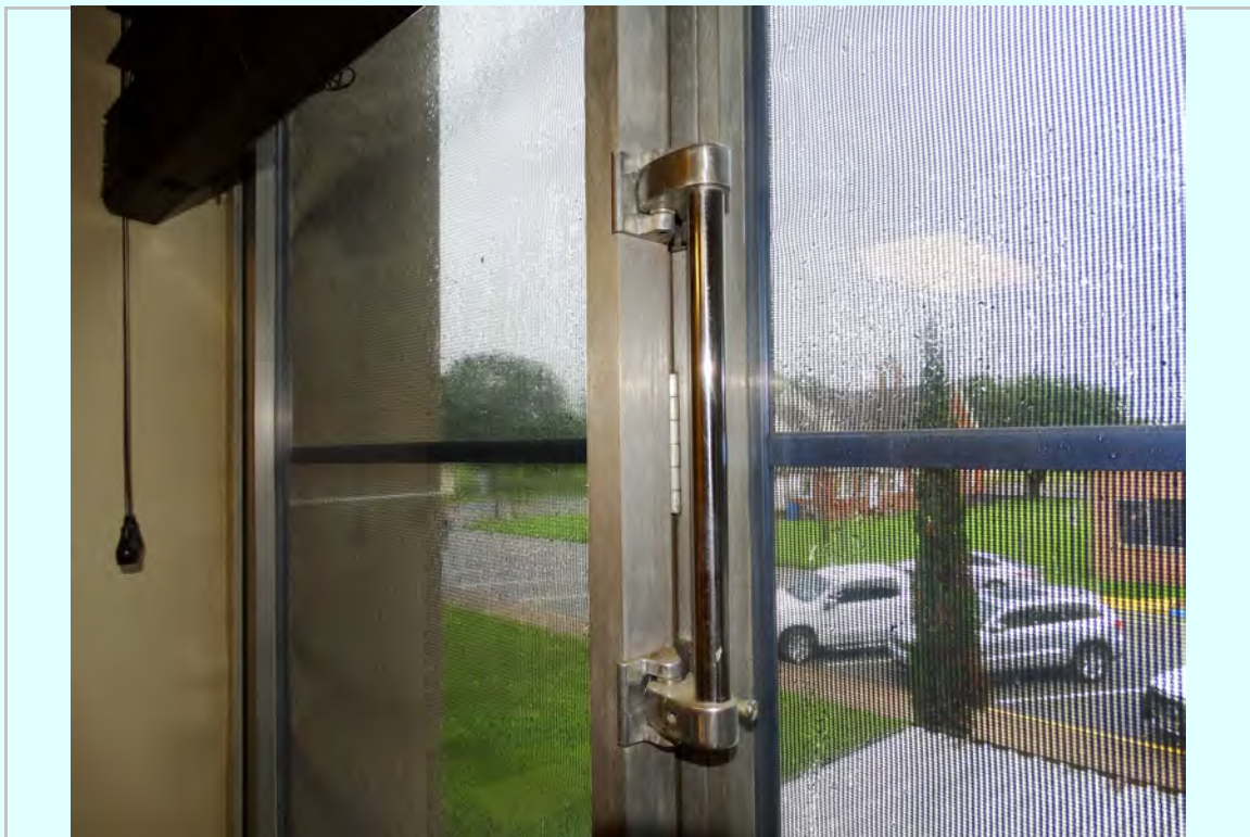
Photo: 2nd floor window existing condition at operator hardware
