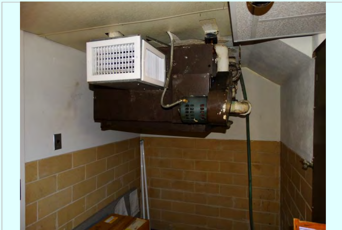
Photo: County Clerk storage below and mechanical equipment
