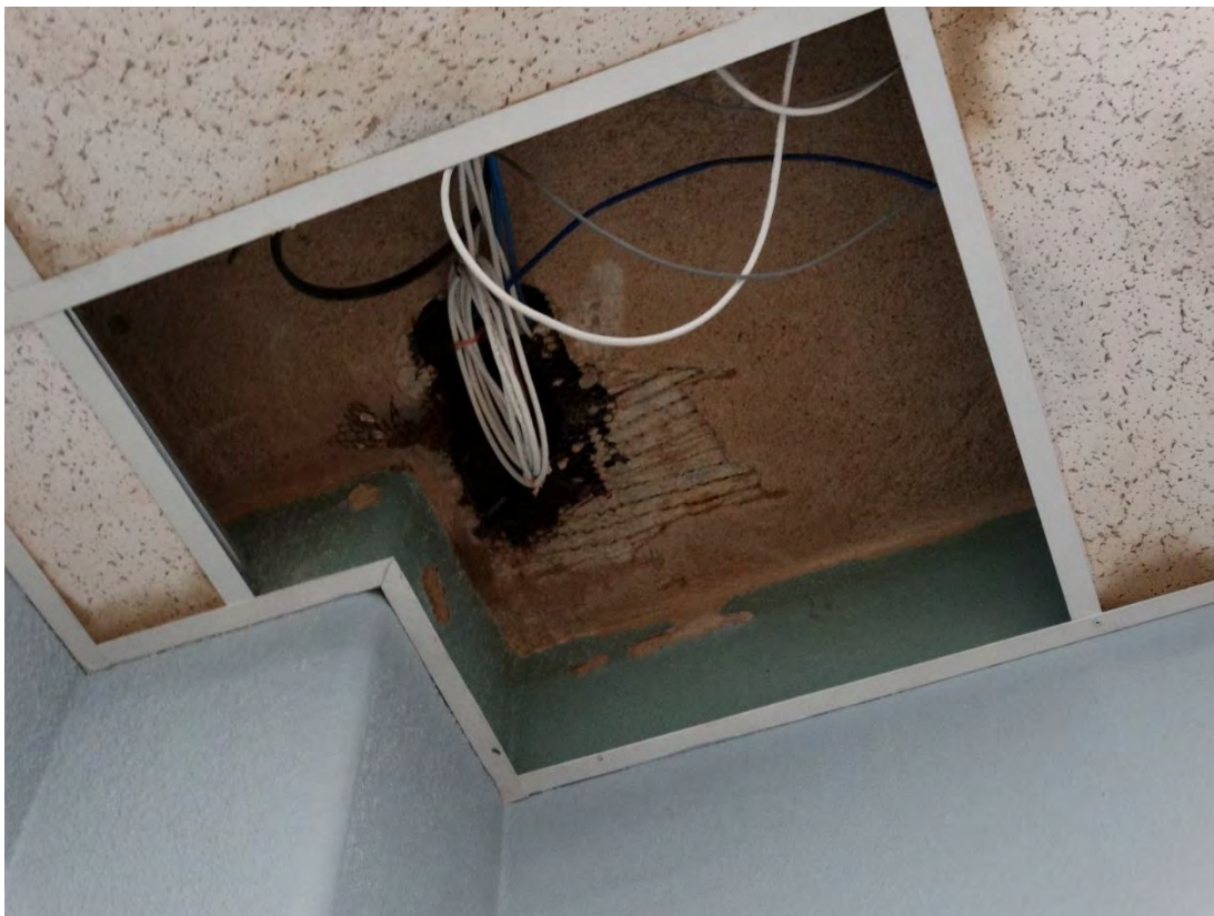
Figure 35. Original acoustical plaster ceiling and possible color
