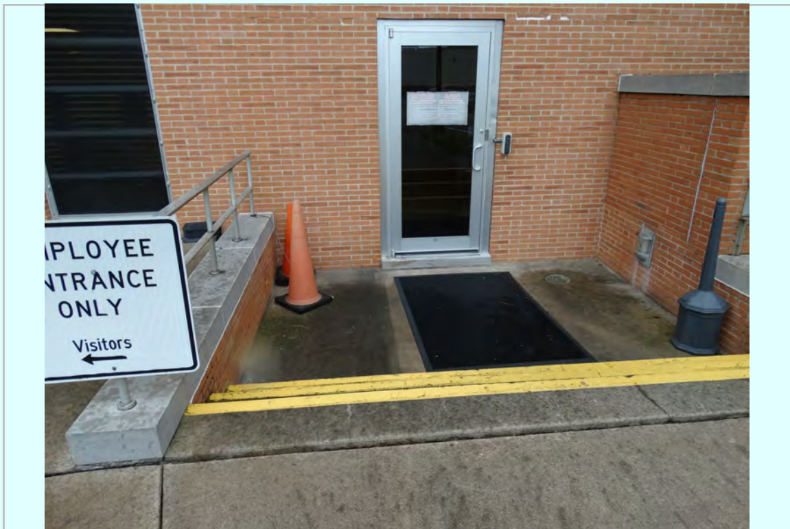
Photo: Non-accessible west entry, no handrails, non-compliant door
