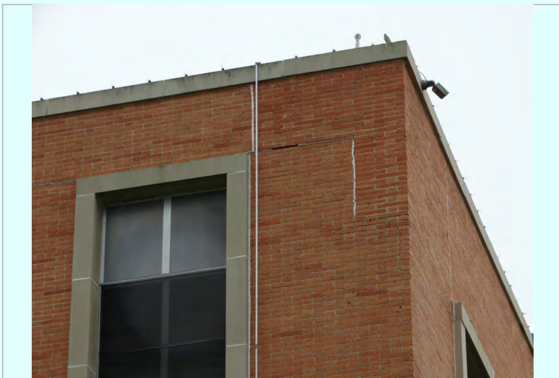
Photo: North Elevation, masonry cracking, mortar joints failing
