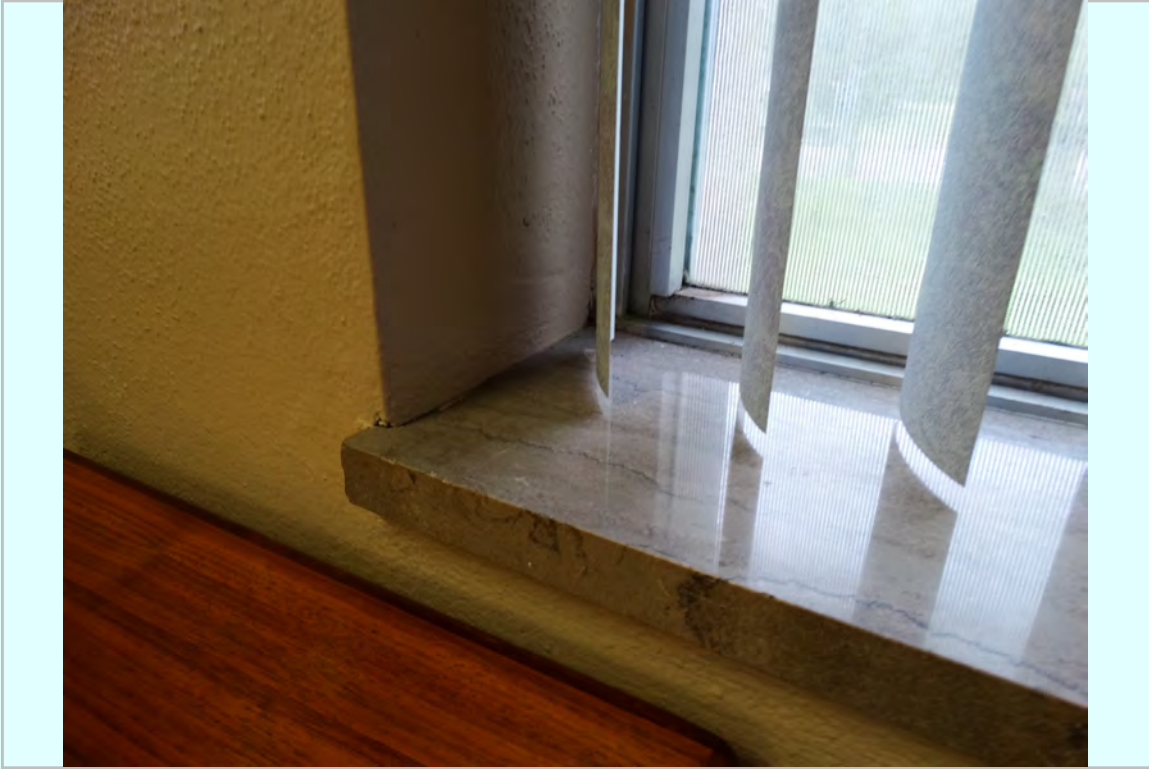
Photo: 2nd floor existing window condition
