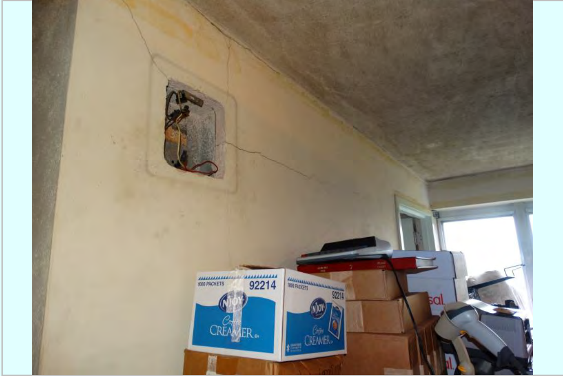
Photo: Fourth floor storage space
