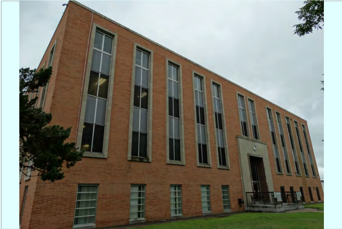
Photo: North Elevation
