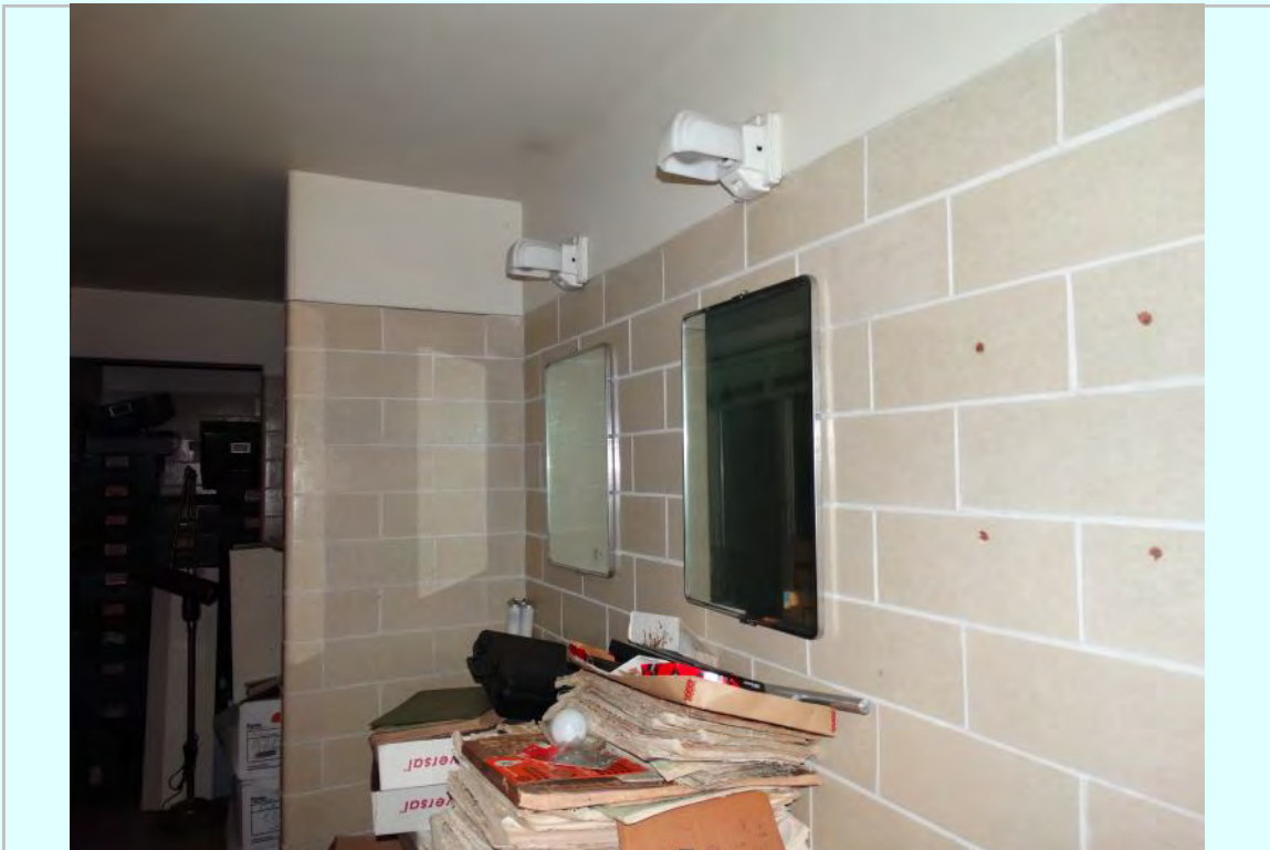
Photo: Fourth floor restrooms being used as storage space
