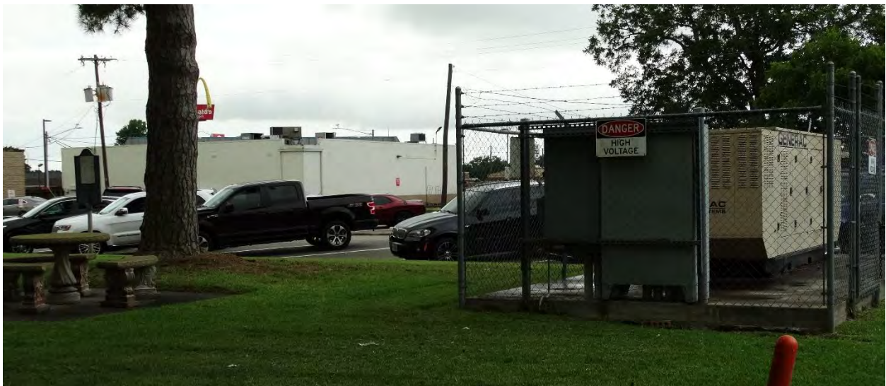
Figure 18. Chain linked fence electrical yard, for backup generator at northwest corner
