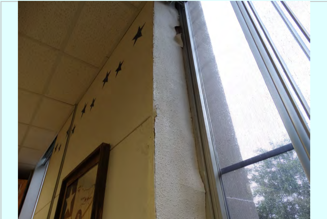
Photo: 3rd floor existing window moisture infiltration and damage
