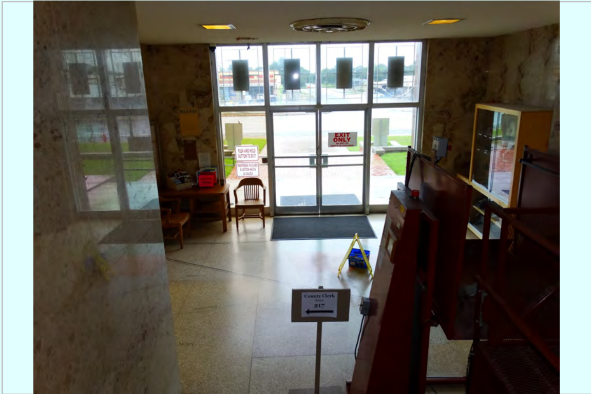
Photo: South elevation curtain wall from interior
