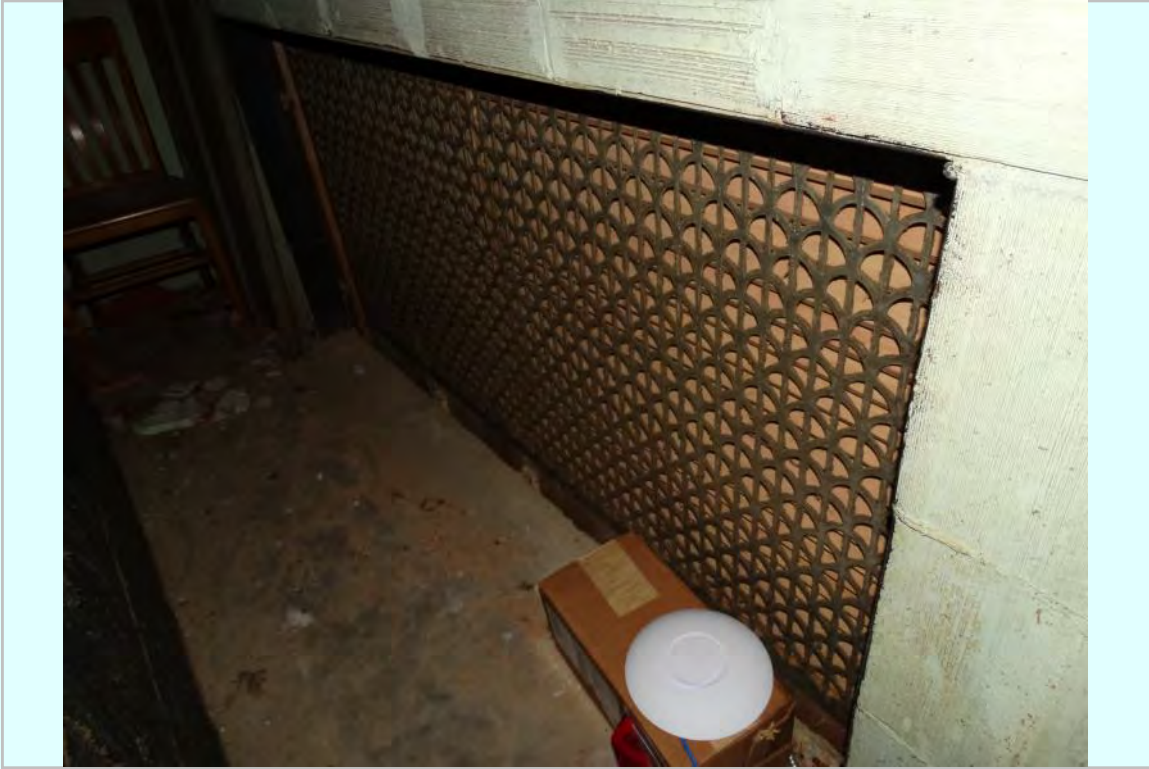
Photo: Fourth floor, mechanical space ventilation into district courtroom
