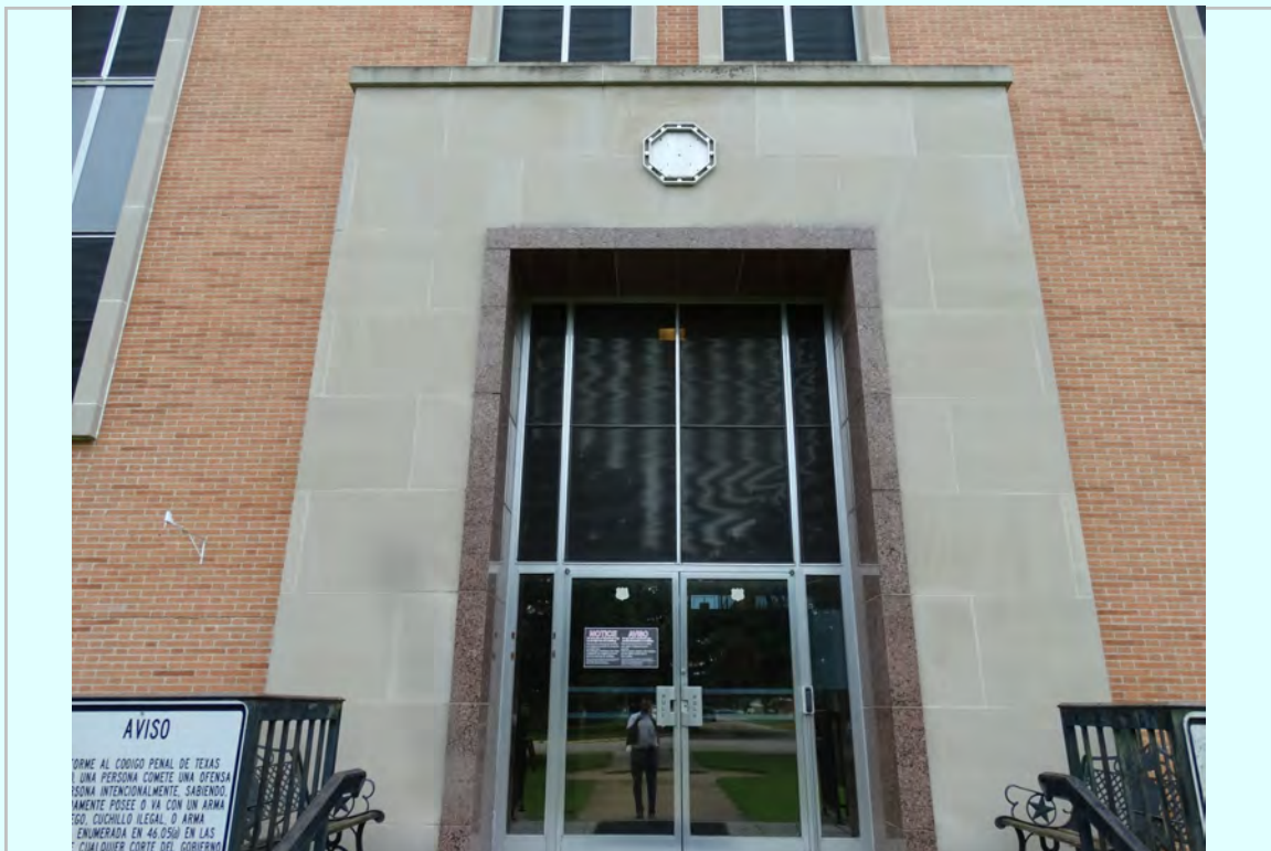
Photo: North Entry , missing clock, masonry staining
