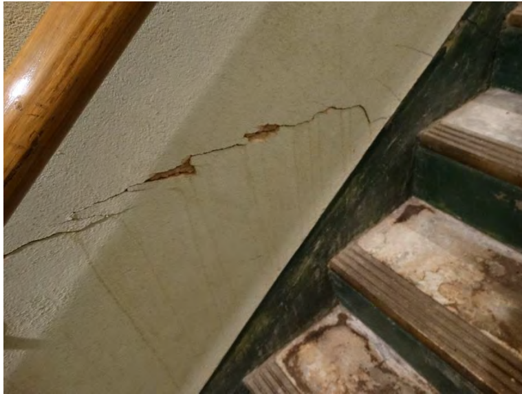
Figure 47. Existing damage at the private stairs to the fourth floor
