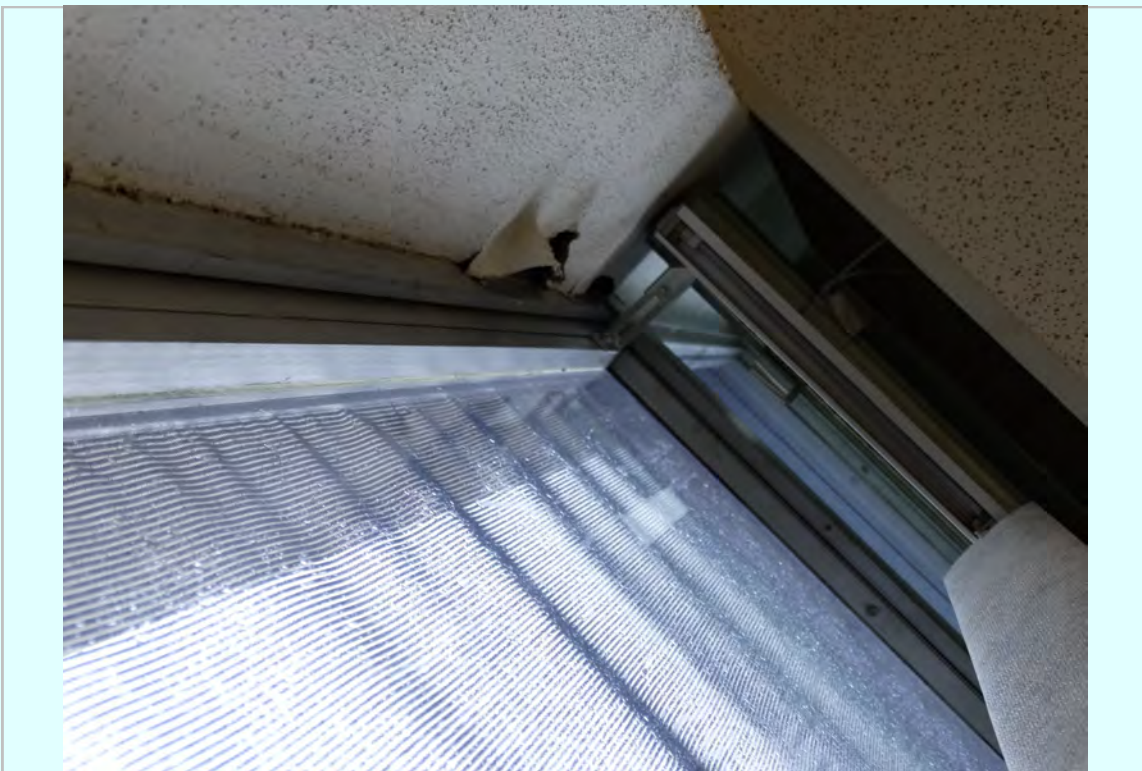
Photo: 3rd floor existing window pocket at ceiling
