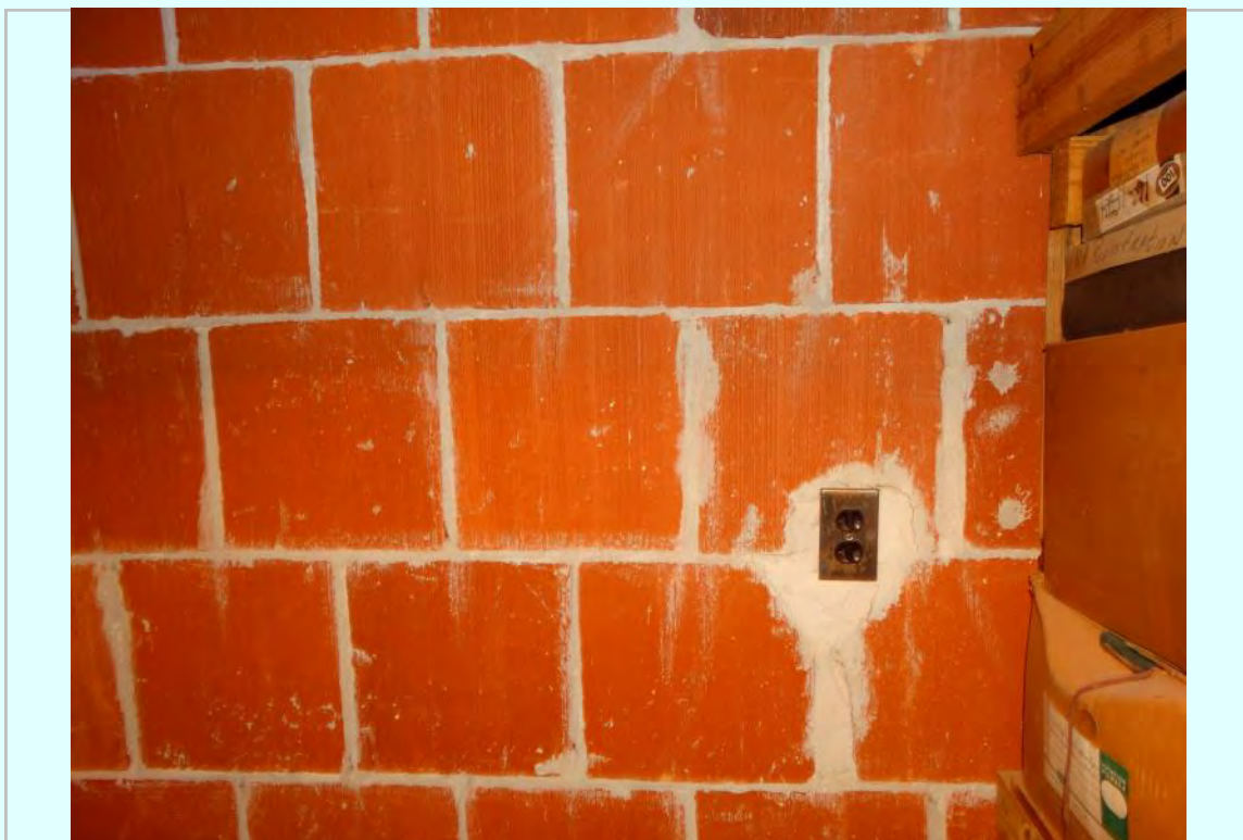
Photo: Fourth floor, typical wall construction
