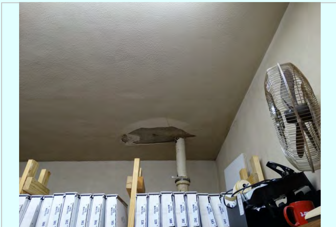
Photo: Third floor office space/storage ceiling damage, spalling
