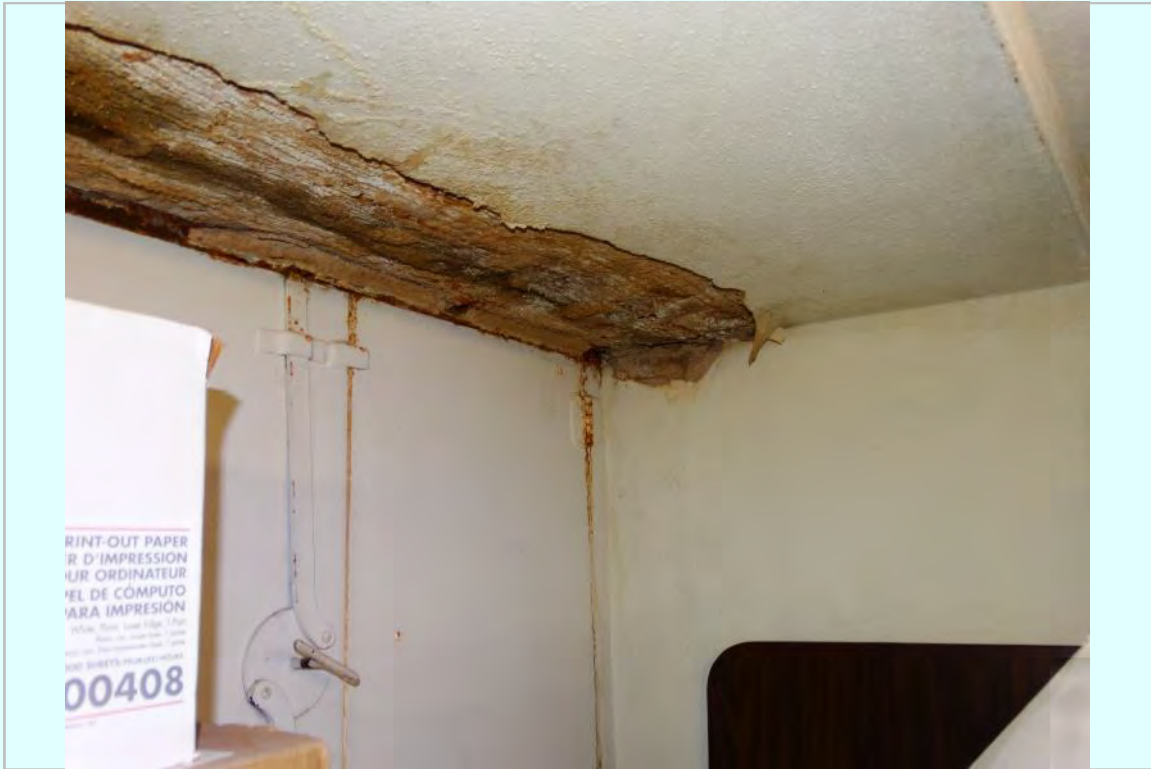
Photo: Severe moisture damage at ceiling in storage space below County Auditor
