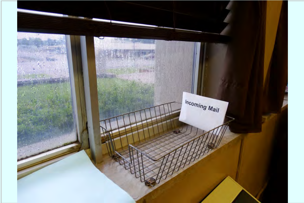
Photo: 2nd floor existing window stool
