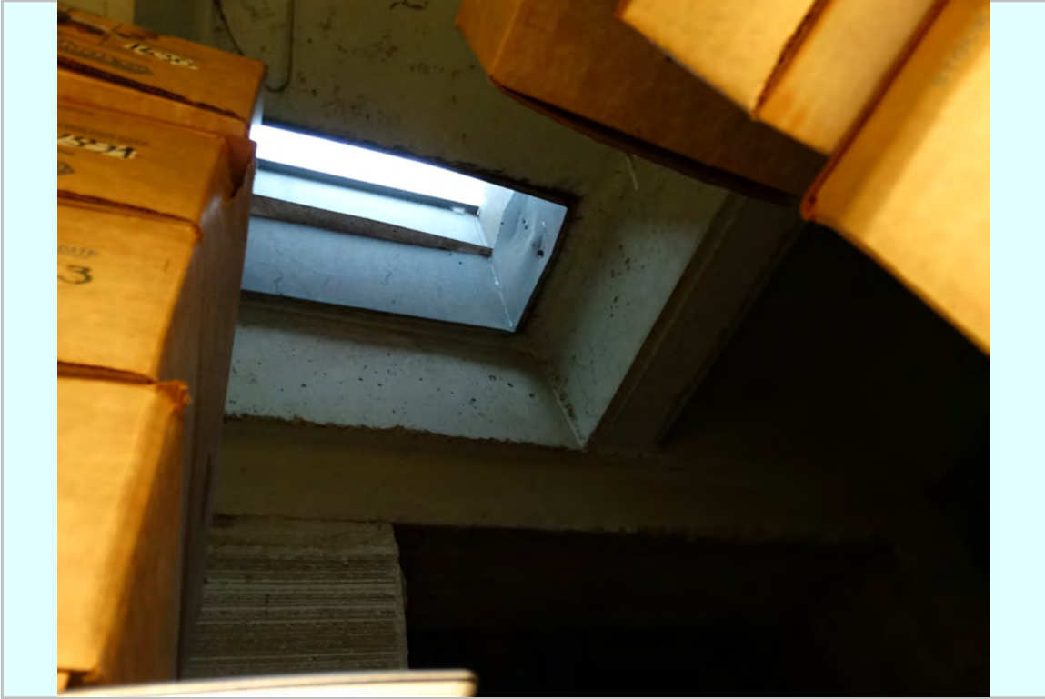
Photo: 4th floor existing skylight
