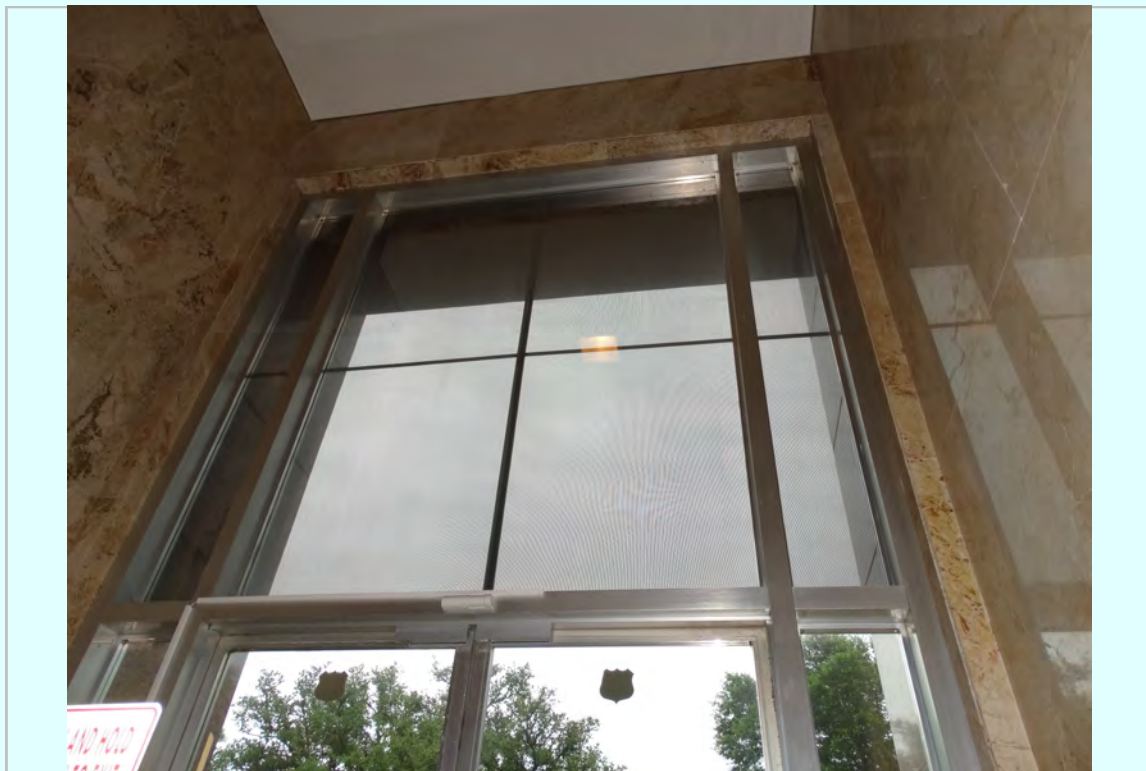
Photo: North curtain wall at central stair
