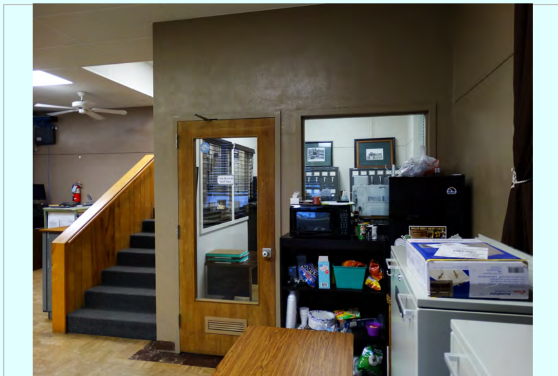
Photo: Non-compliant stair and railing
