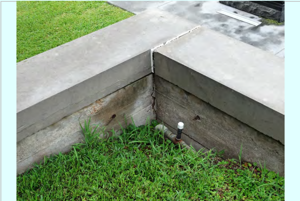
Photo: South entry retaining wall cracking and coping joint failing
