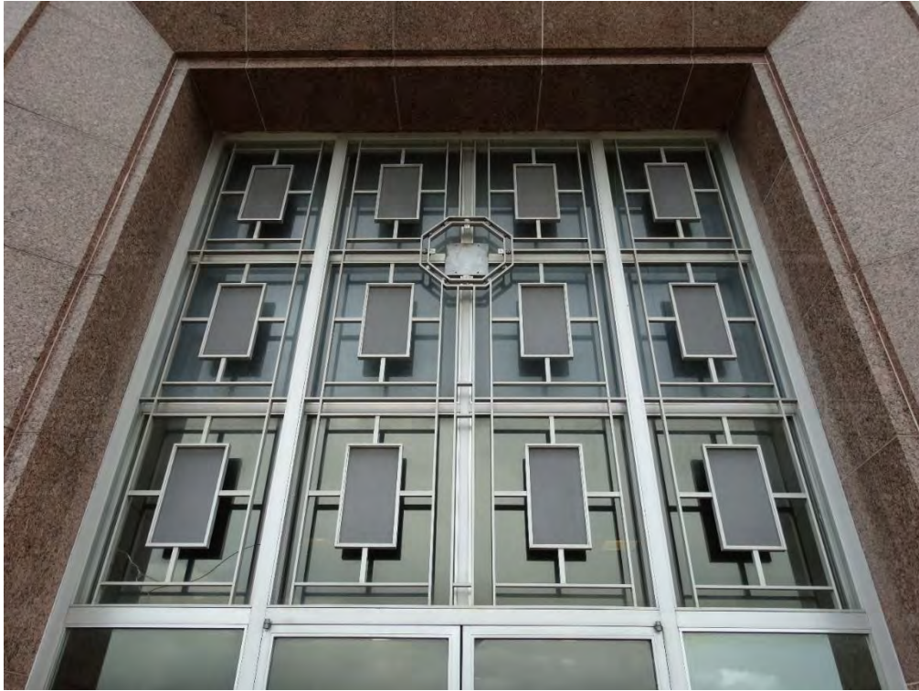
Figure 33. South façade curtain wall with aluminum shade grille and missing clock
