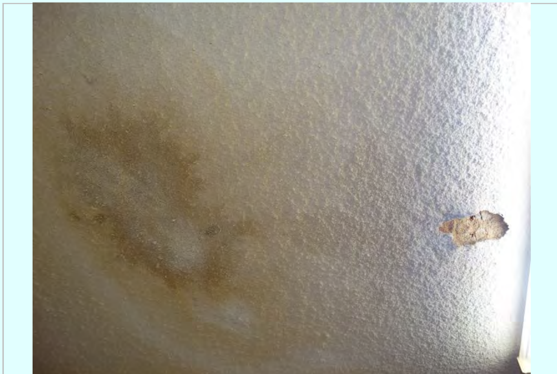
Photo: Third floor corridor ceiling damage, biological growth and spalling
