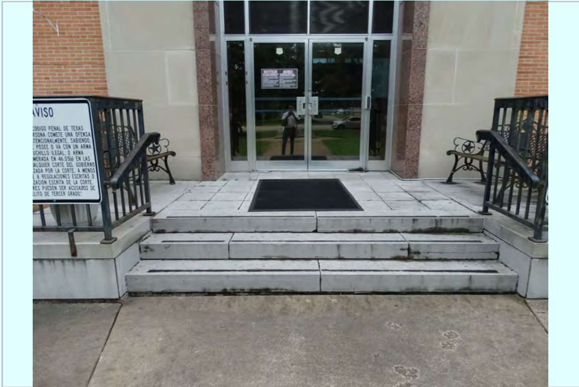
Photo: Non-accessible south entry, non-compliant handrails, non-compliant door
