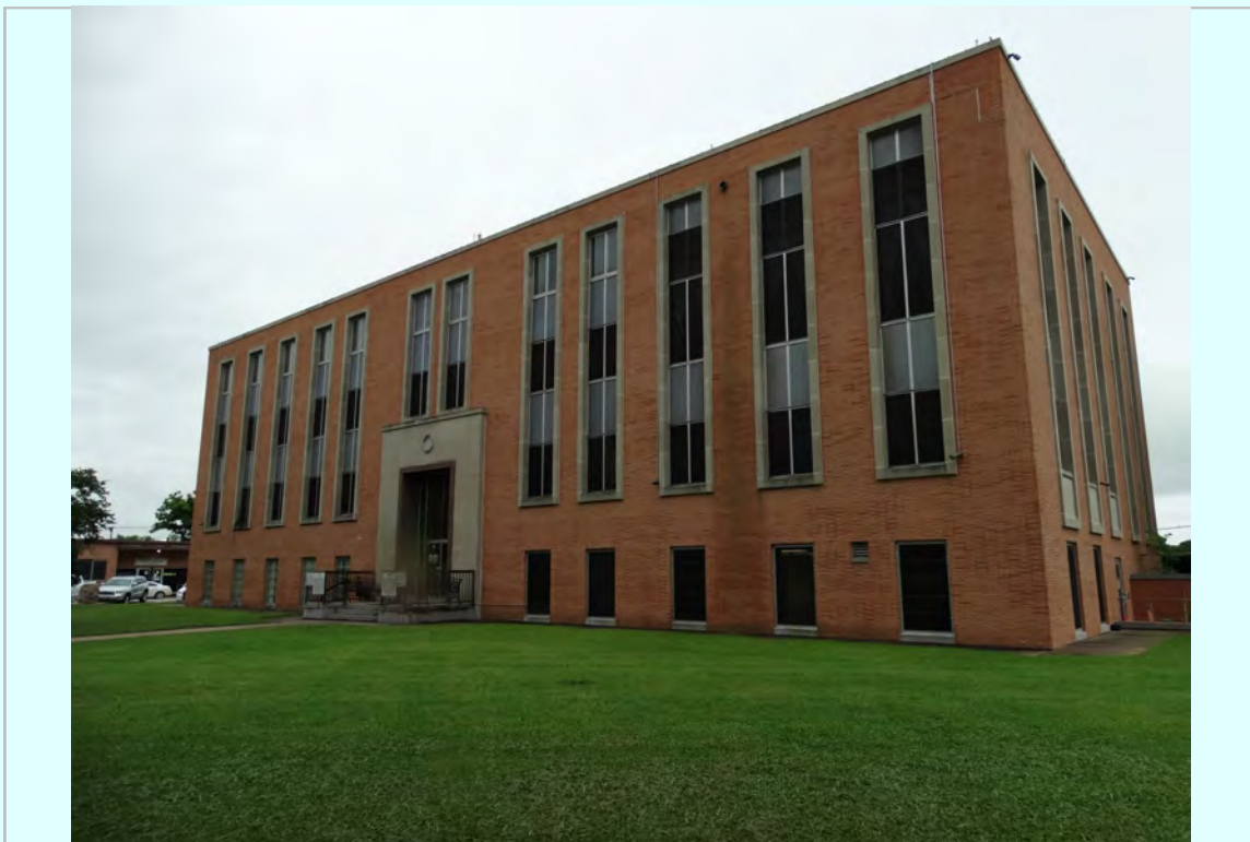
Photo: North Elevation
