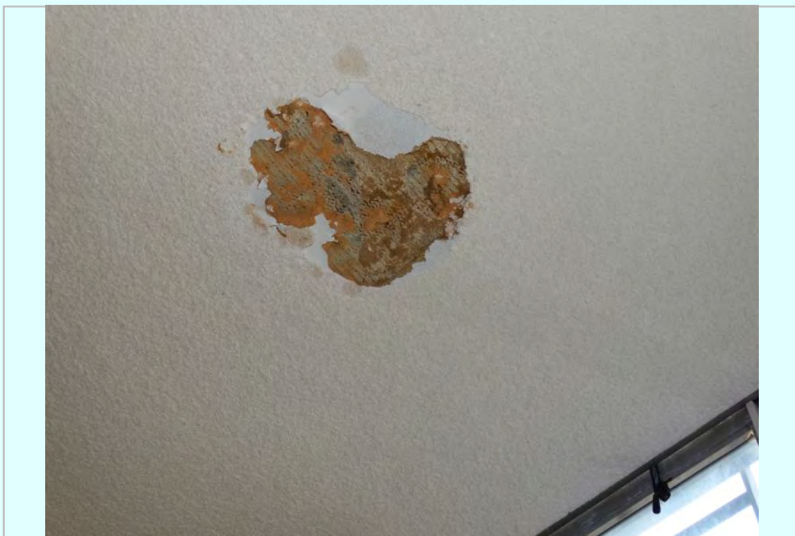
Photo: Mezzanine lobby ceiling damage
