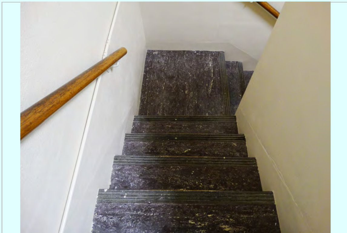
Photo: Non-compliant stair and railing
