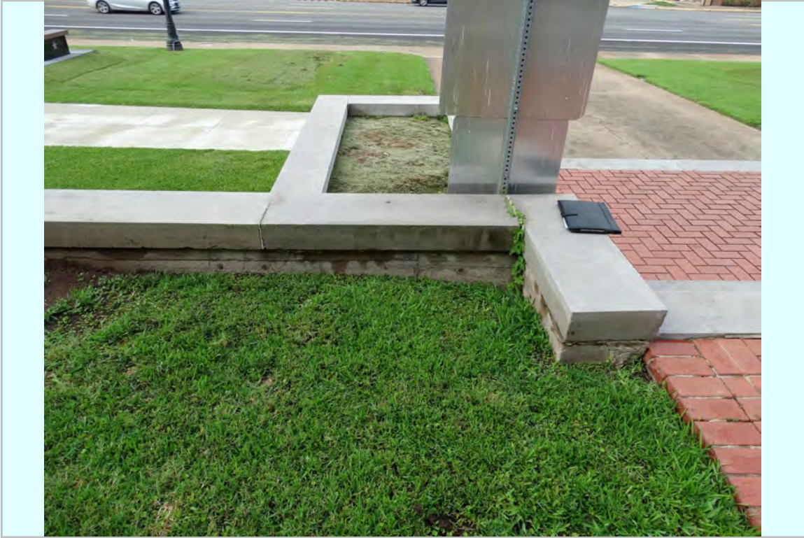
Photo: South entry retaining wall condition
