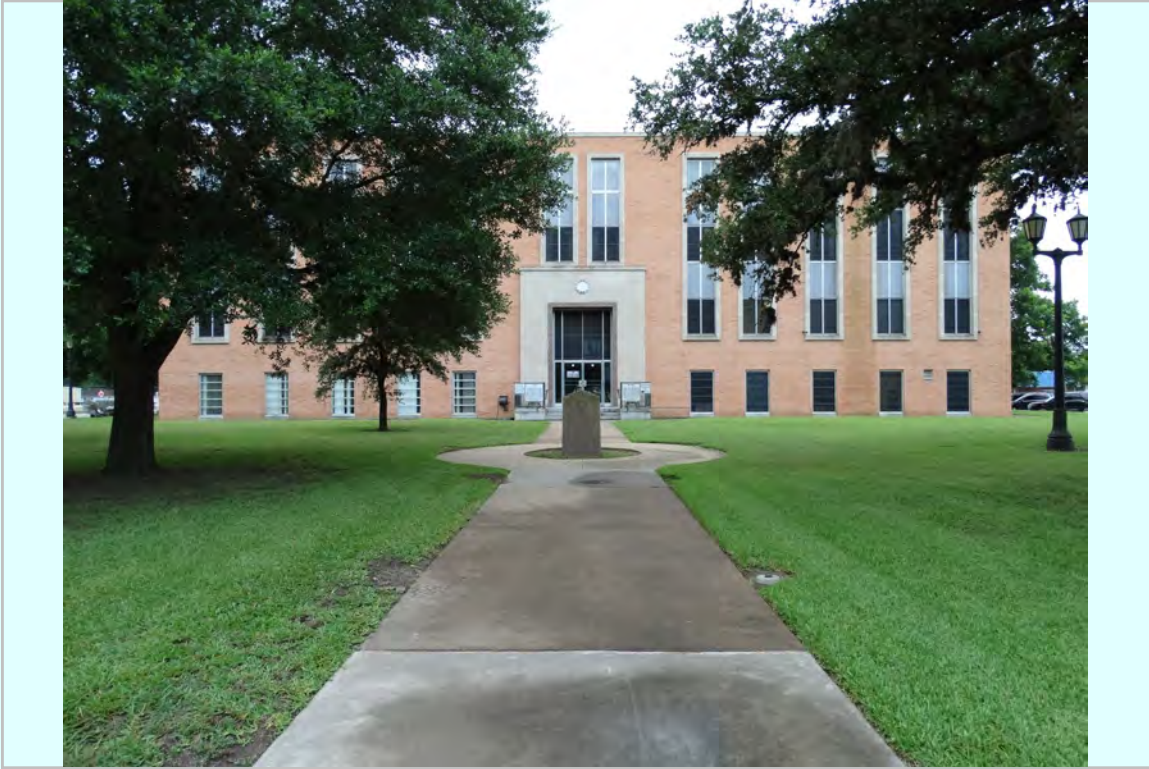
Photo: North Elevation
