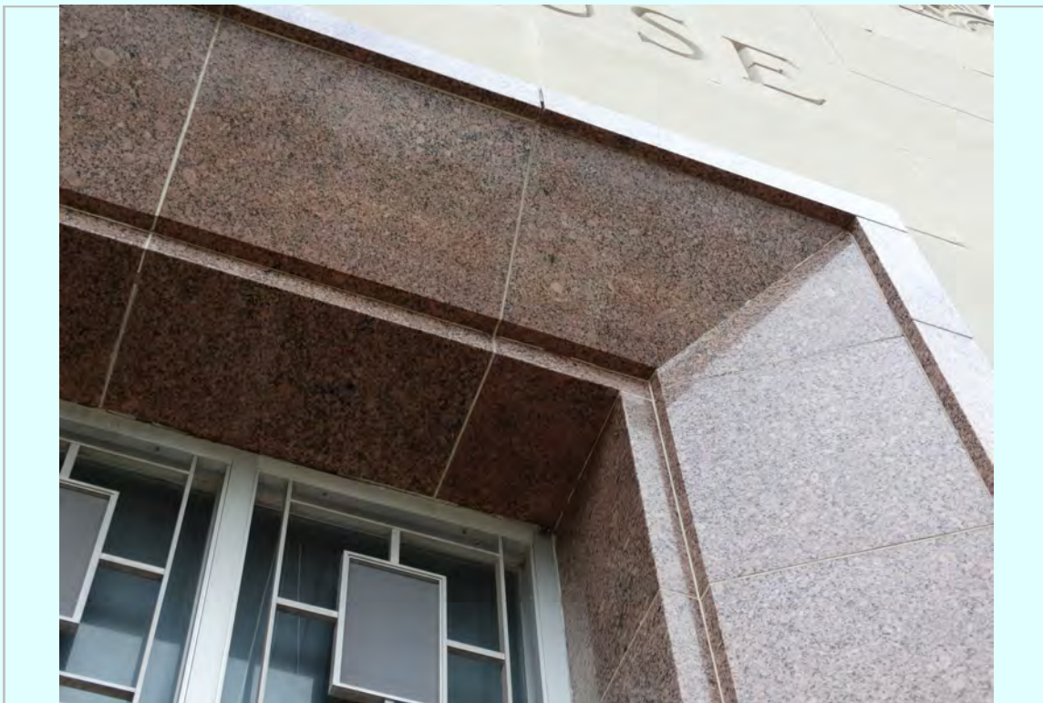
Photo: South Elevation, entry detailing
