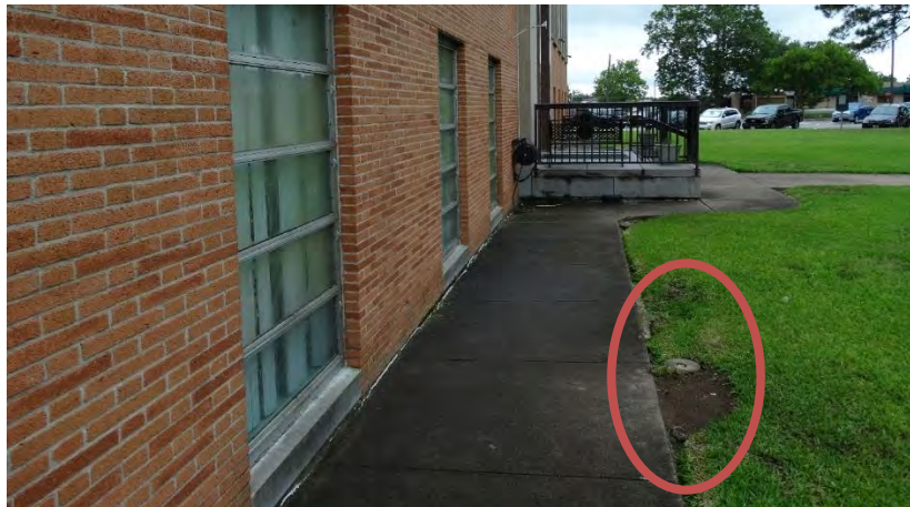
Figure 20. soil erosion occurring along north elevation walkway
