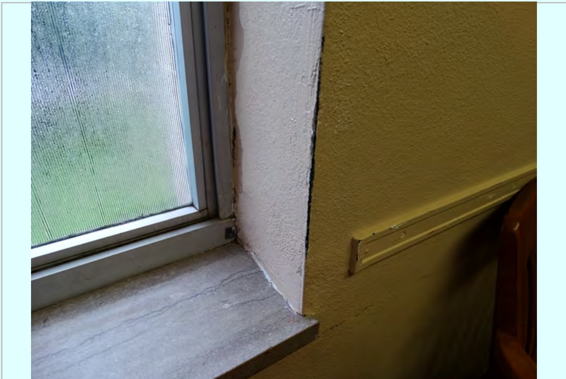
Photo: 3rd floor existing window at stool
