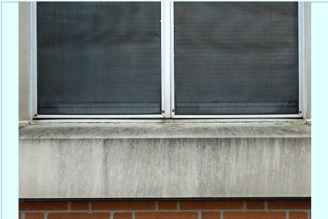
Photo: Typical sill condition
