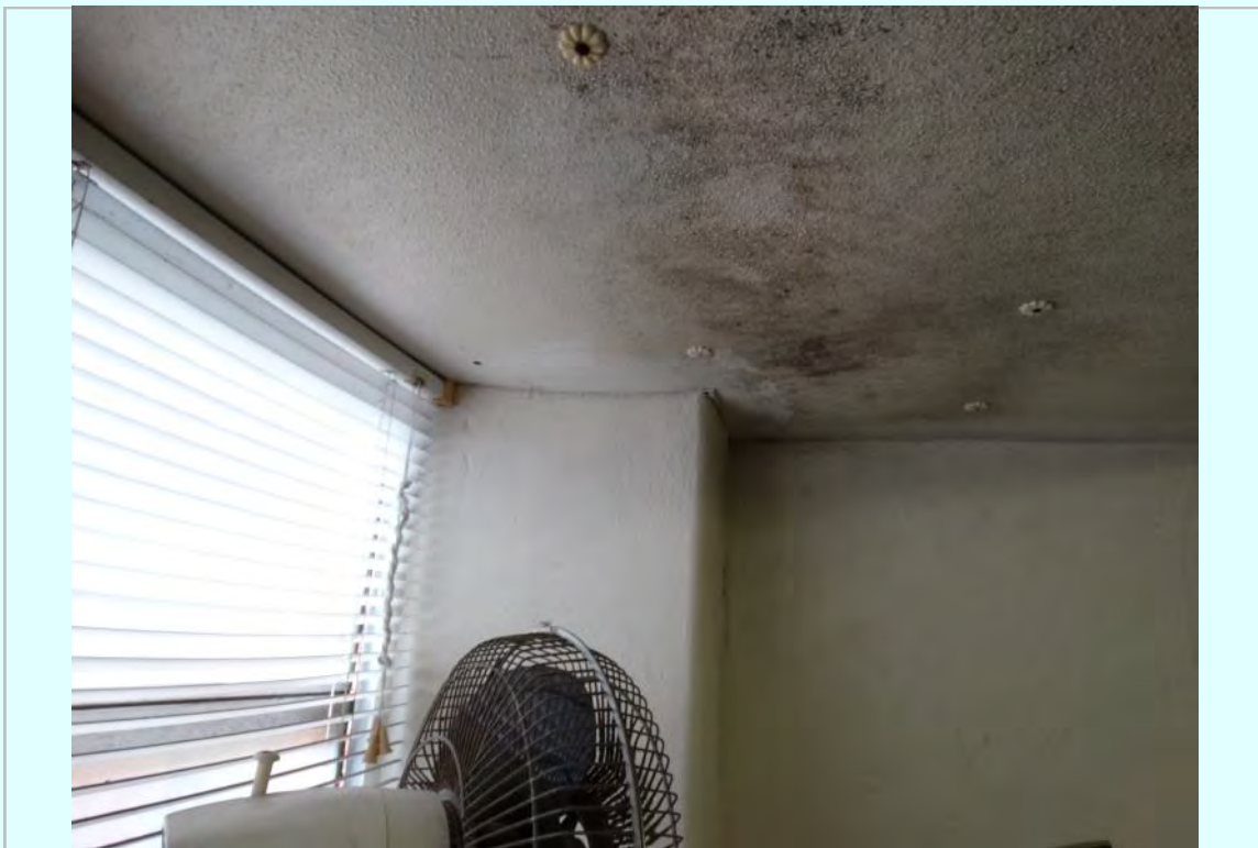
Photo: First floor ceiling moisture damage and biological growth
