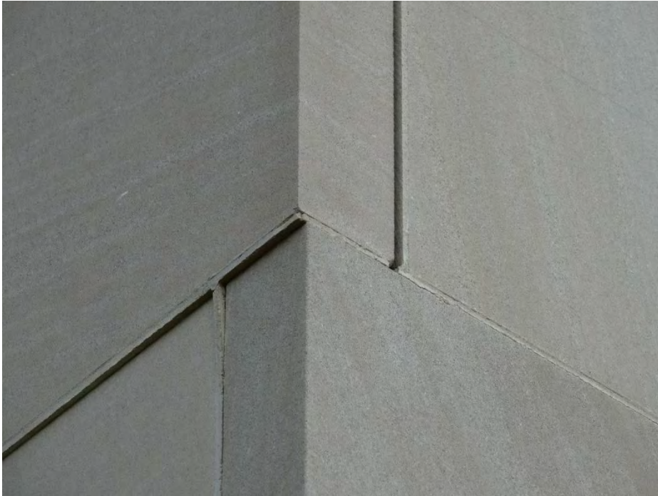
Figure 24. Limestone mortar and movement damage on south façade masonry
