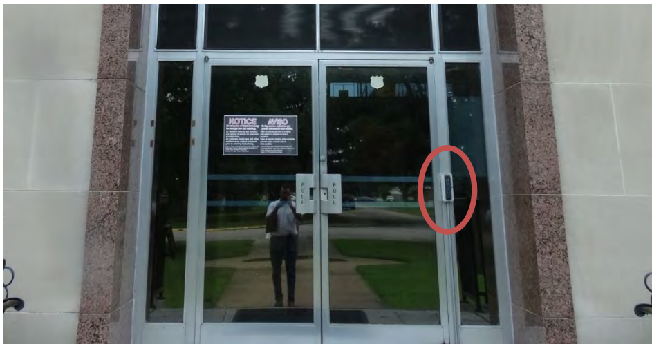
Figure 27. Keypad modification at original north entry doors
