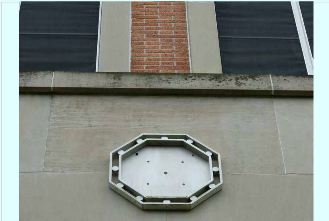
Photo: North entry, missing element, coping moisture staining and biological growth
