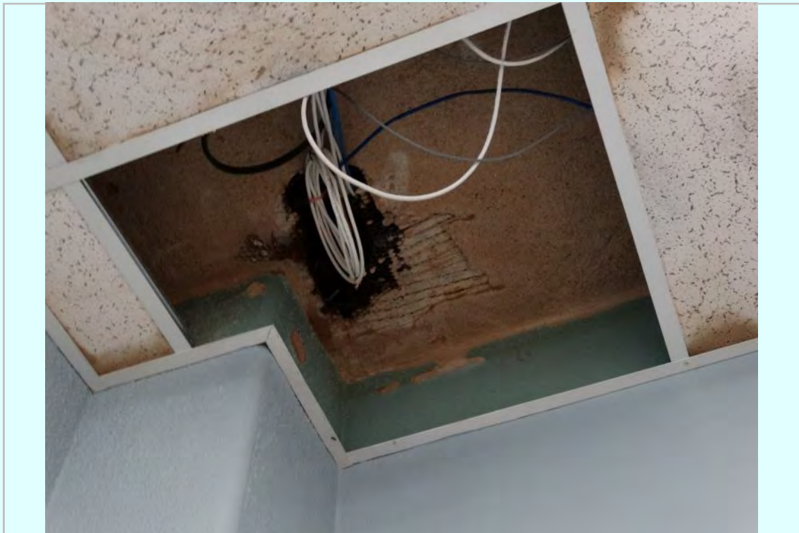
Photo: First floor plenum and possible original ceiling
