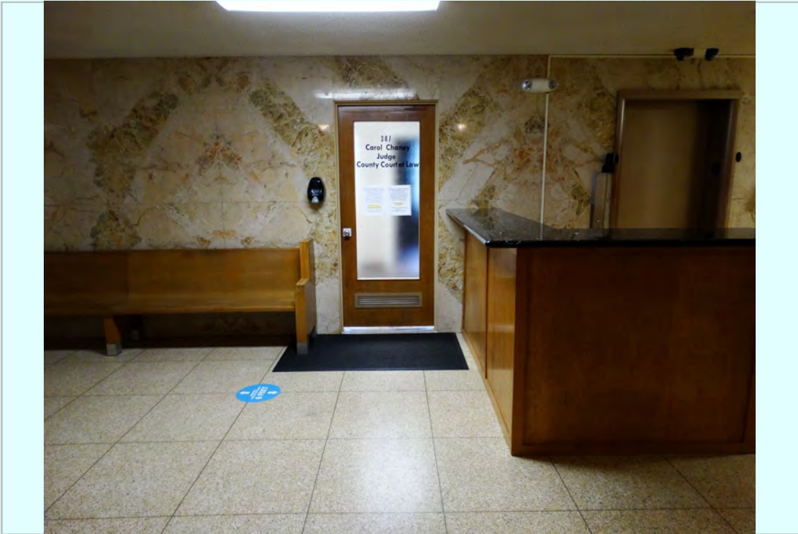
Photo: Non-compliant door hardware and help desk counter missing wheelchair access
