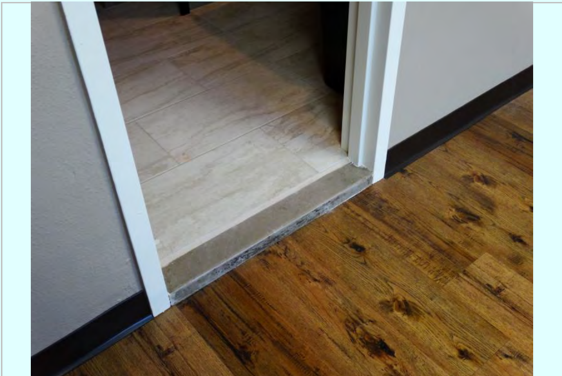
Photo: Third floor recently renovated office space
