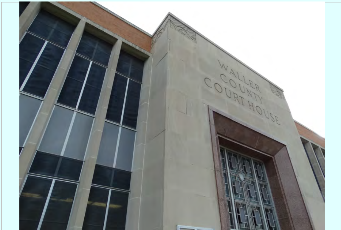
Photo: South Elevation, entry
