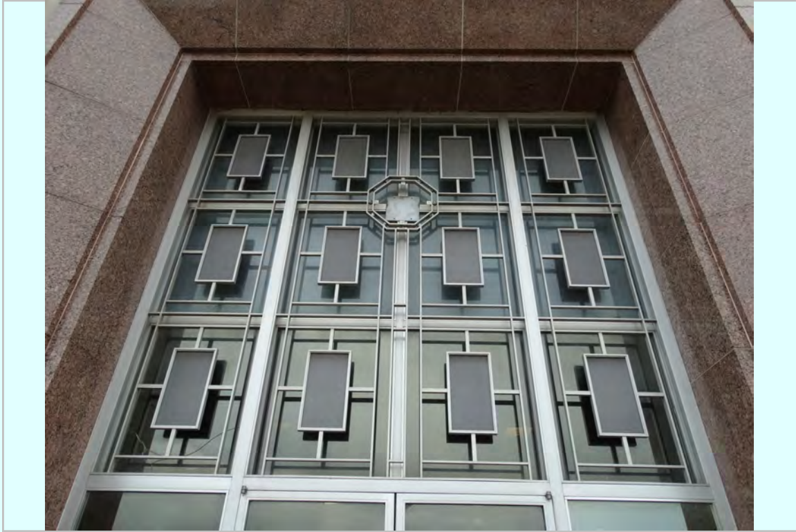
Photo: South Entry at curtain wall with aluminum screening
