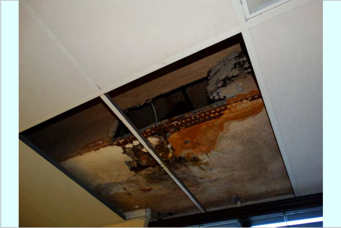
Photo: Storage space above County Clerk , moisture damage from HVAC
