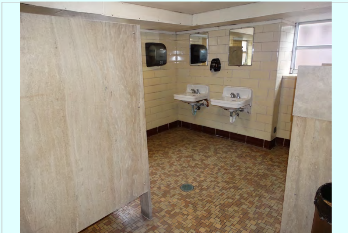
Photo: Non-compliant public restrooms at ground floor
