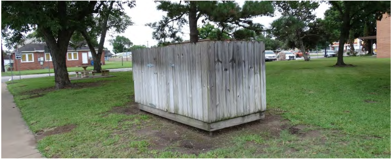
Figure 14. Wooden fence protecting exposed gas lines
