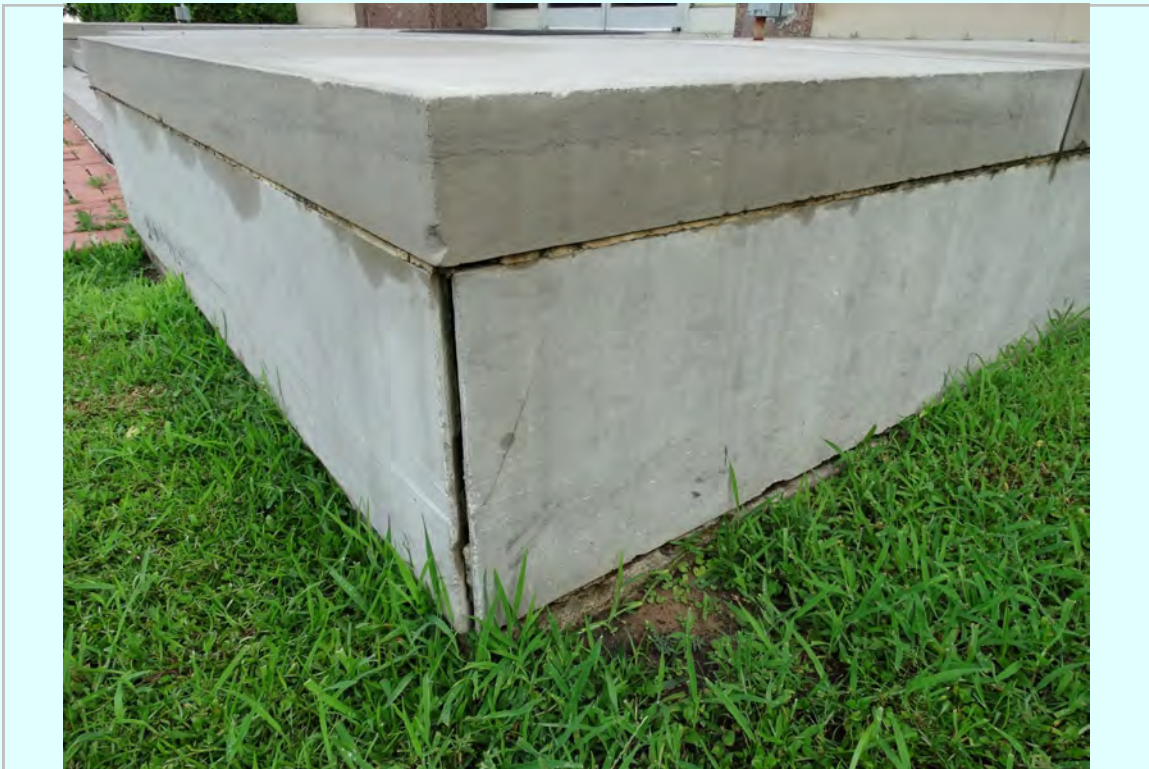
Photo: South entry patio stone joints failing and moisture staining
