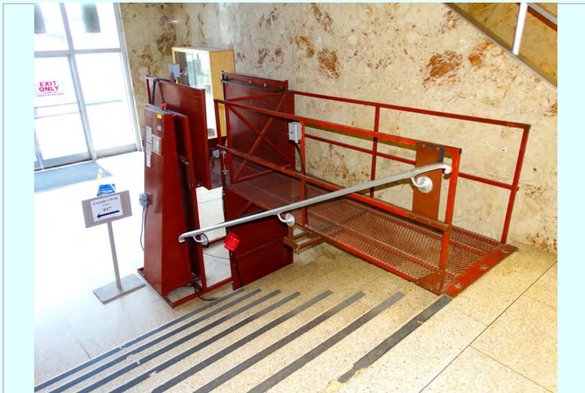
Photo: Wheel chair lift installed at grand stair from half floor to ground floor
