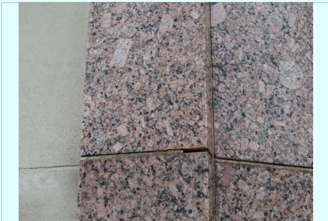
Photo: South Elevation, pink granite mortar joint failing
