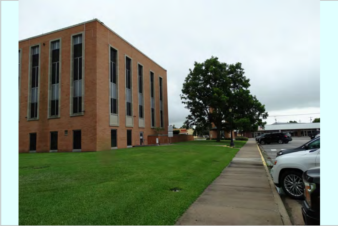
Photo: West Elevation
