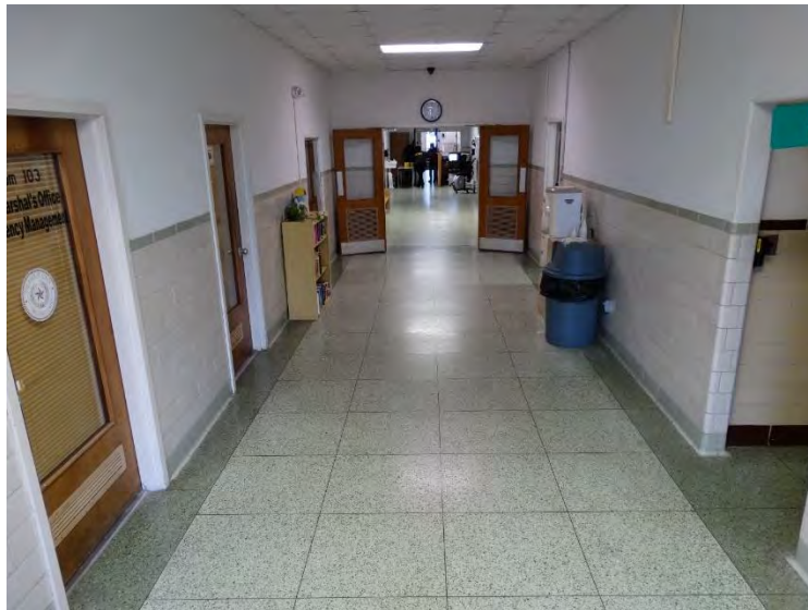
Figure 36. Existing first floor corridor, terrazzo and glazed structural wall tile
