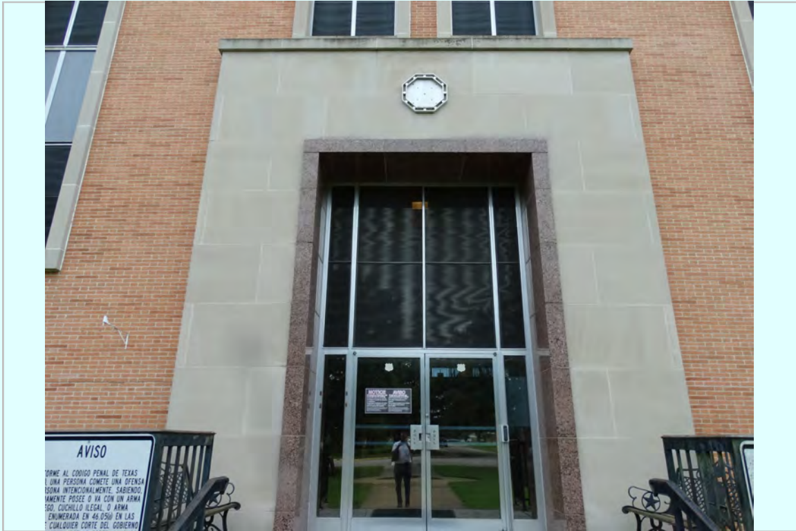
Photo: North elevation curtain wall and original glass door entry
