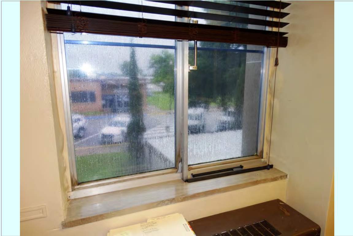
Photo: 2nd floor existing window condition
