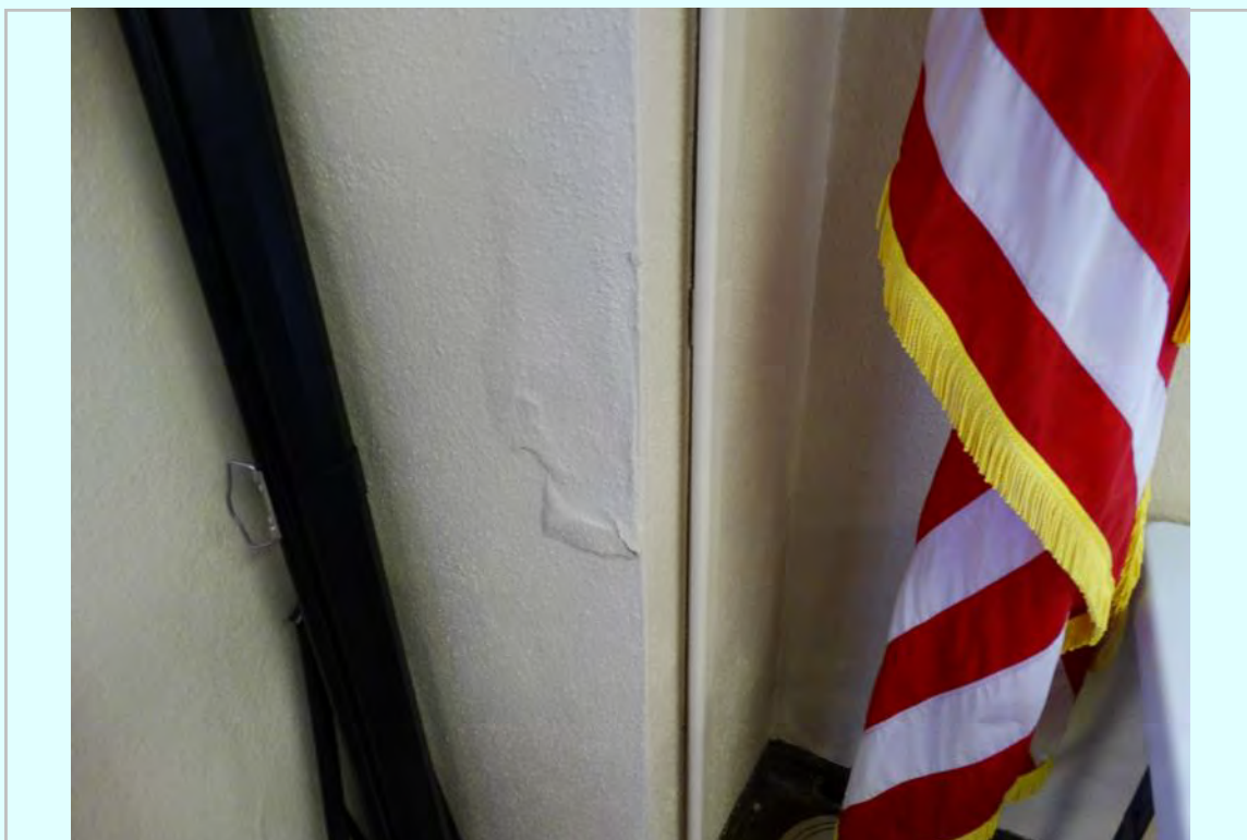
Photo: Second floor Commissioners courtroom moisture damage in outside corner
