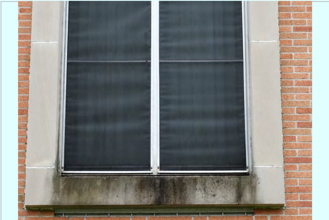
Photo: Typical sill condition at certain areas
