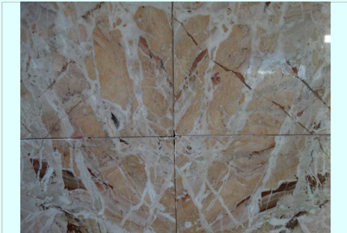
Photo: Typical marble stone condition at central stair
