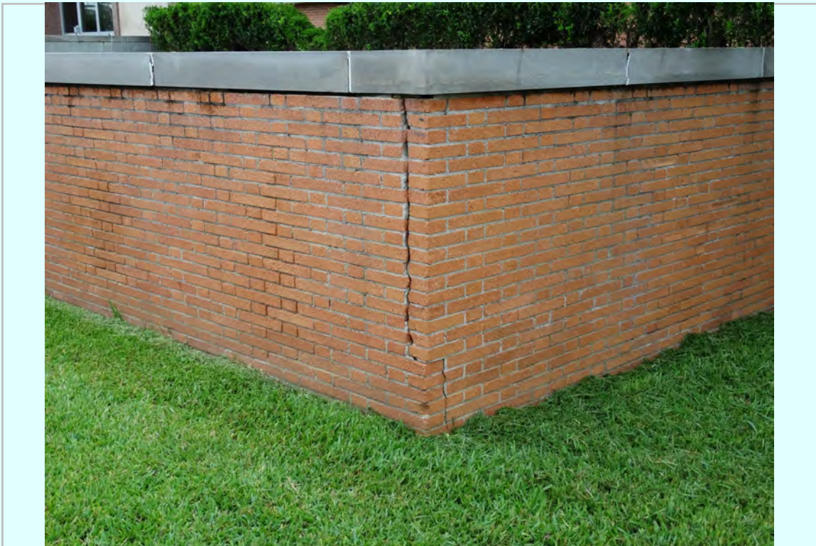
Photo: South entry East retaining wall outside corner, failing
