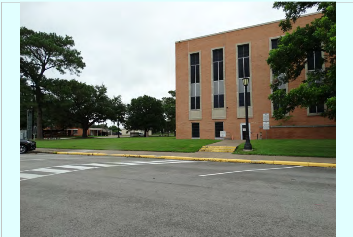
Photo: West Elevation
