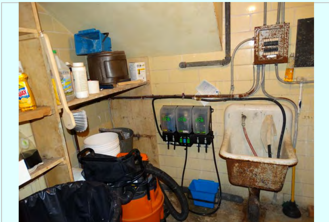
Photo: First floor janitor closet
