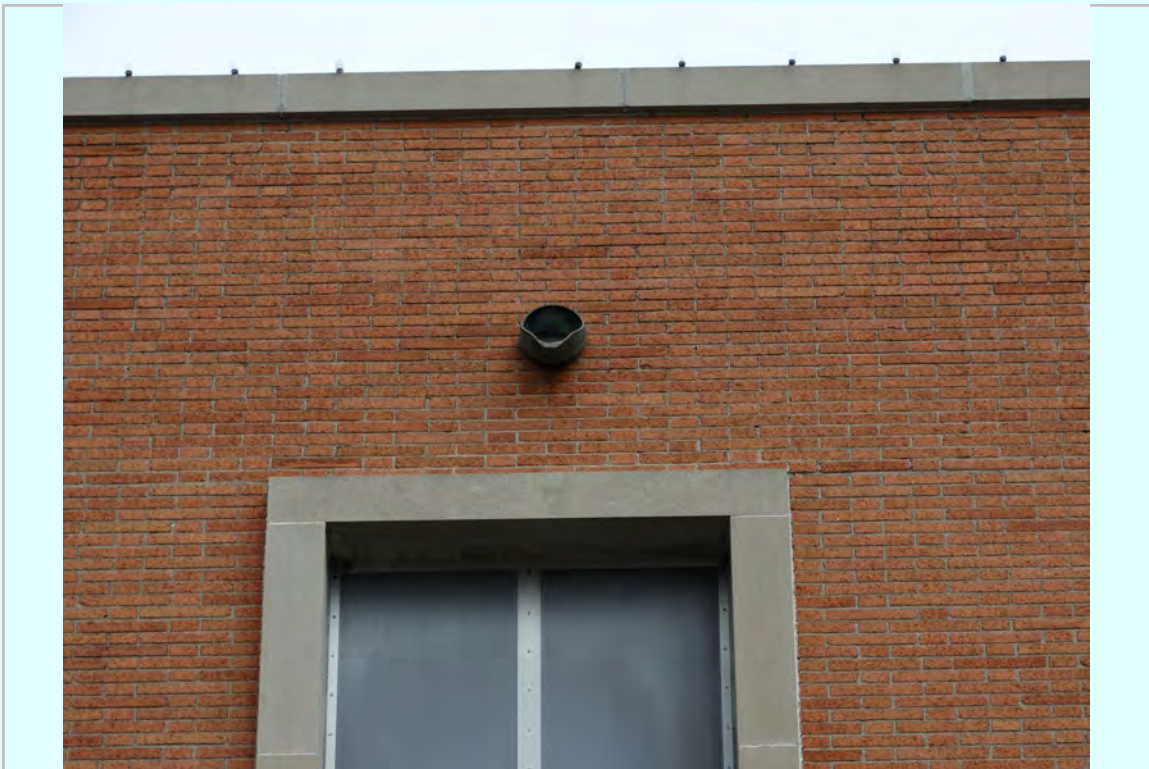
Photo: East Elevation, thru wall scupper, assuming original
