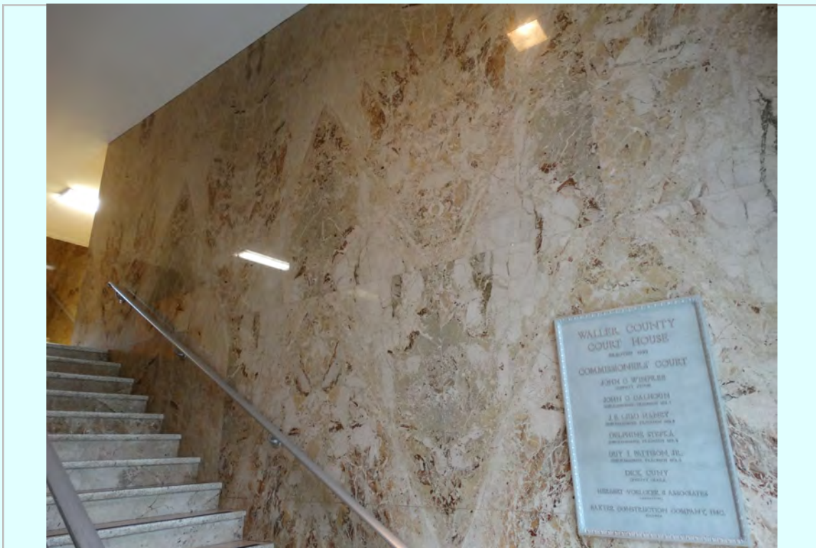
Photo: Central stair typical condition and non compliant handrail
