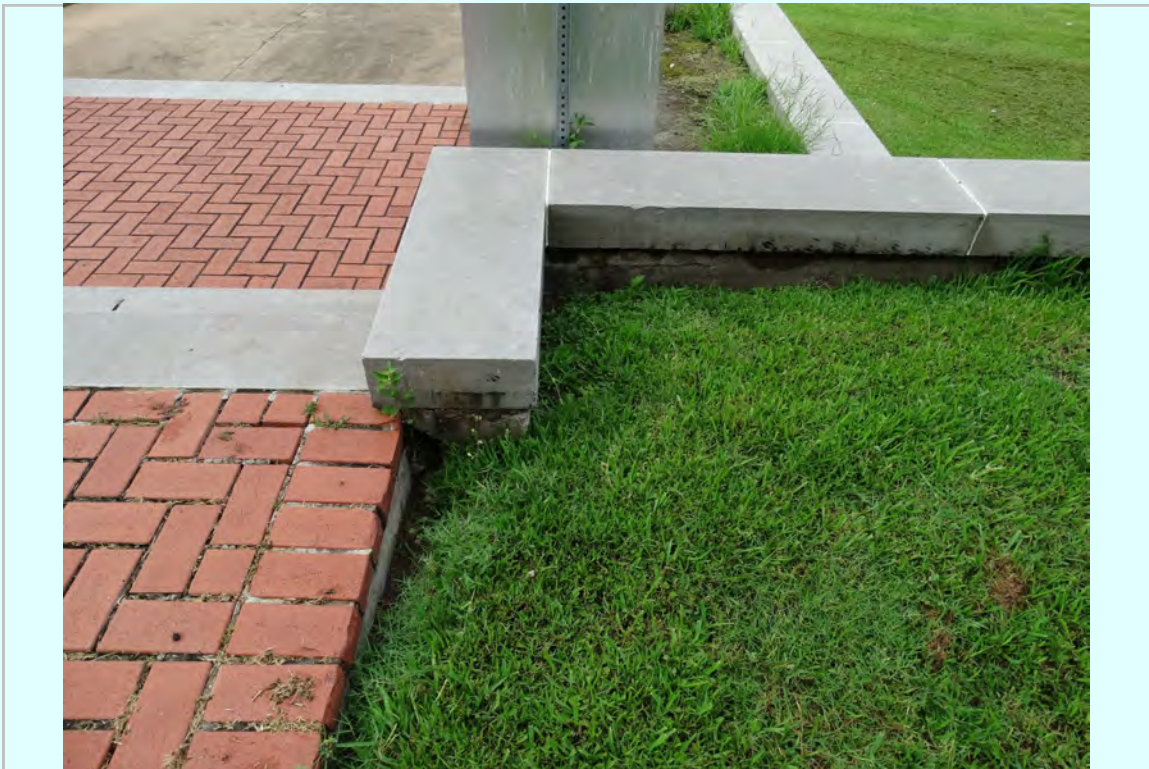
Photo: South entry retaining wall and erosion
