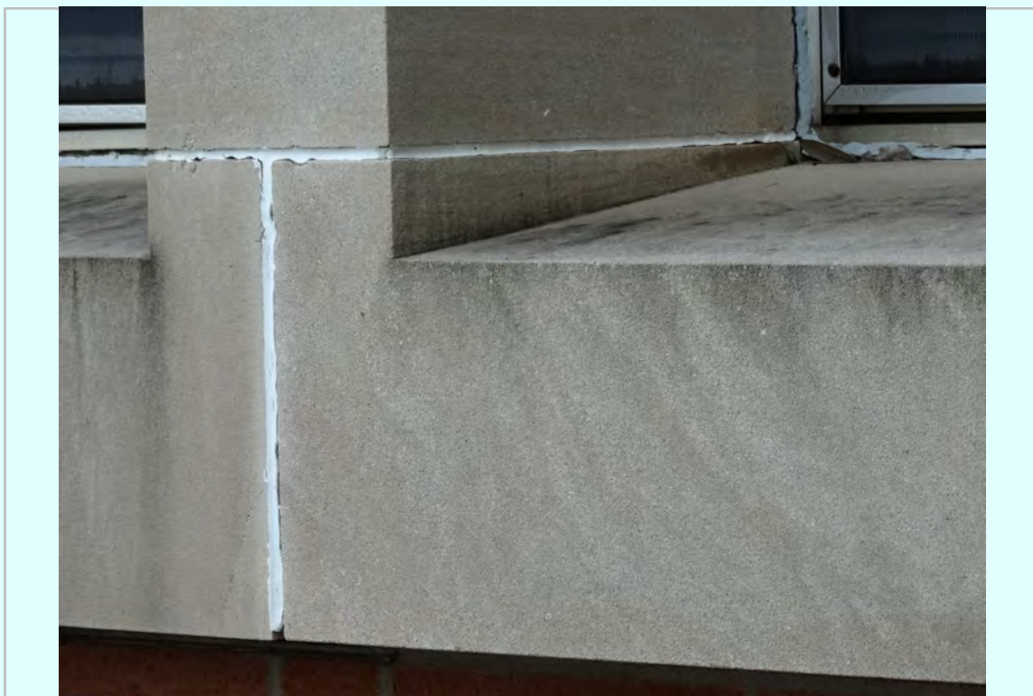
Photo: South Elevation, masonry junction failing, replacement sealant failing
