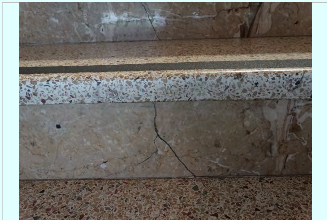
Photo: Crack at marble riser
