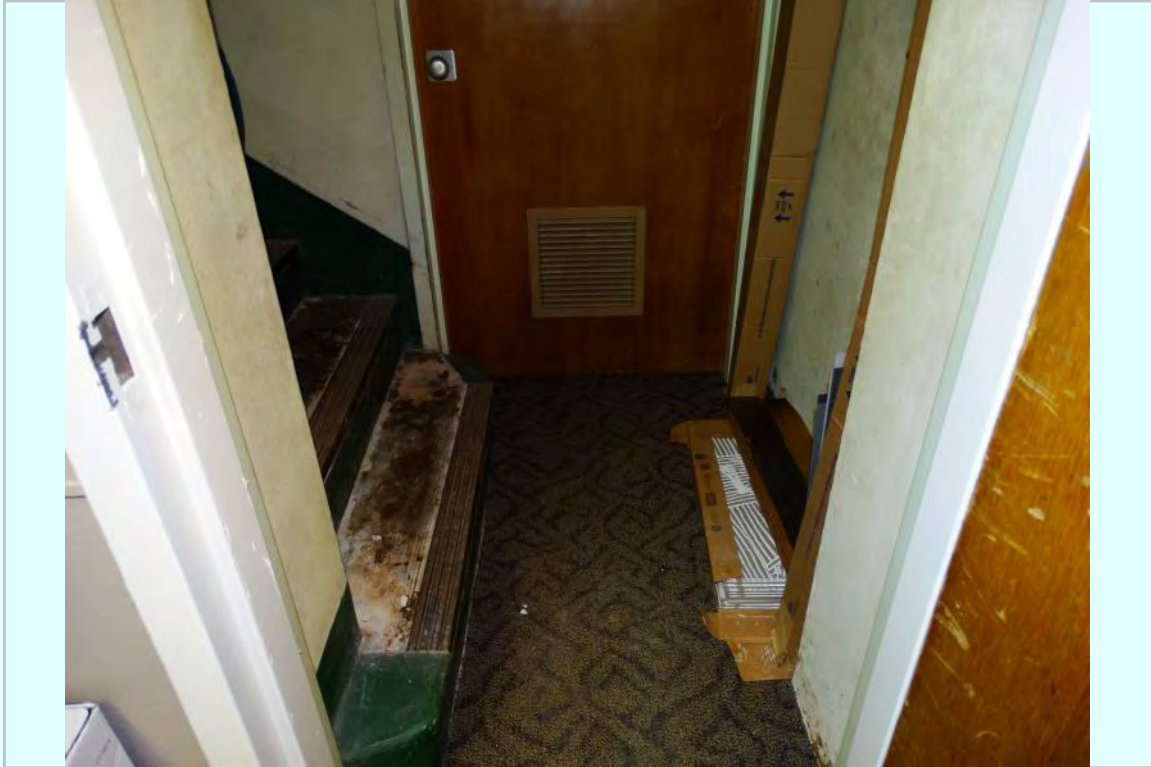
Photo: Third floor private stairs to fourth floor
