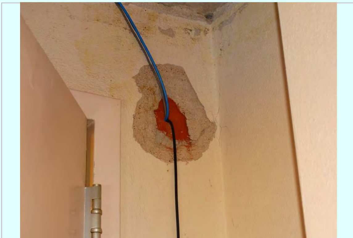
Photo: Fourth floor damage caused by updating for data
