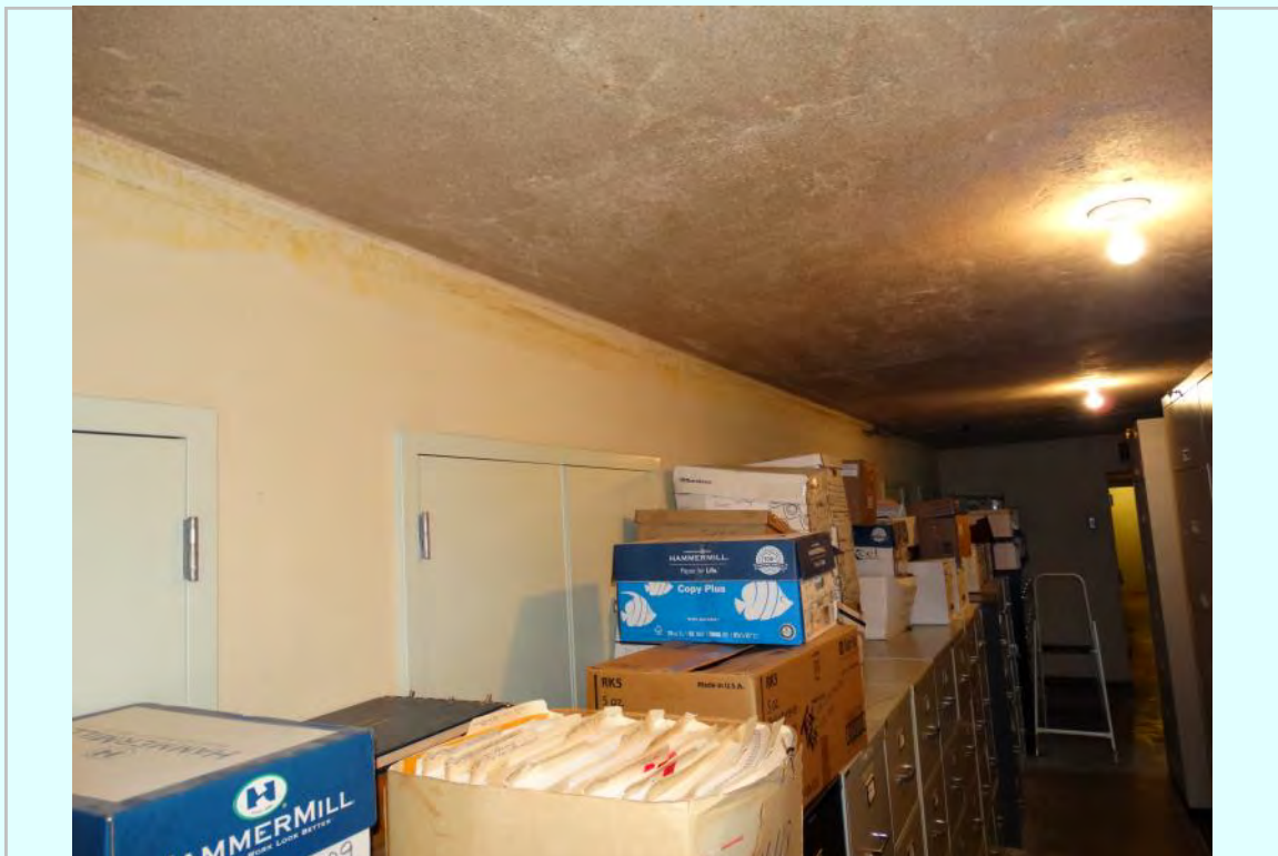
Photo: Fourth floor storage space
