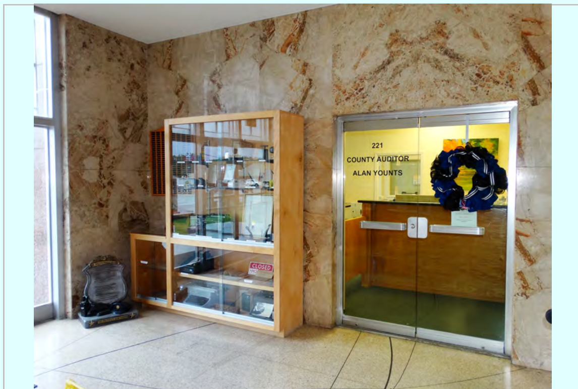
Photo: Non-compliant doors
