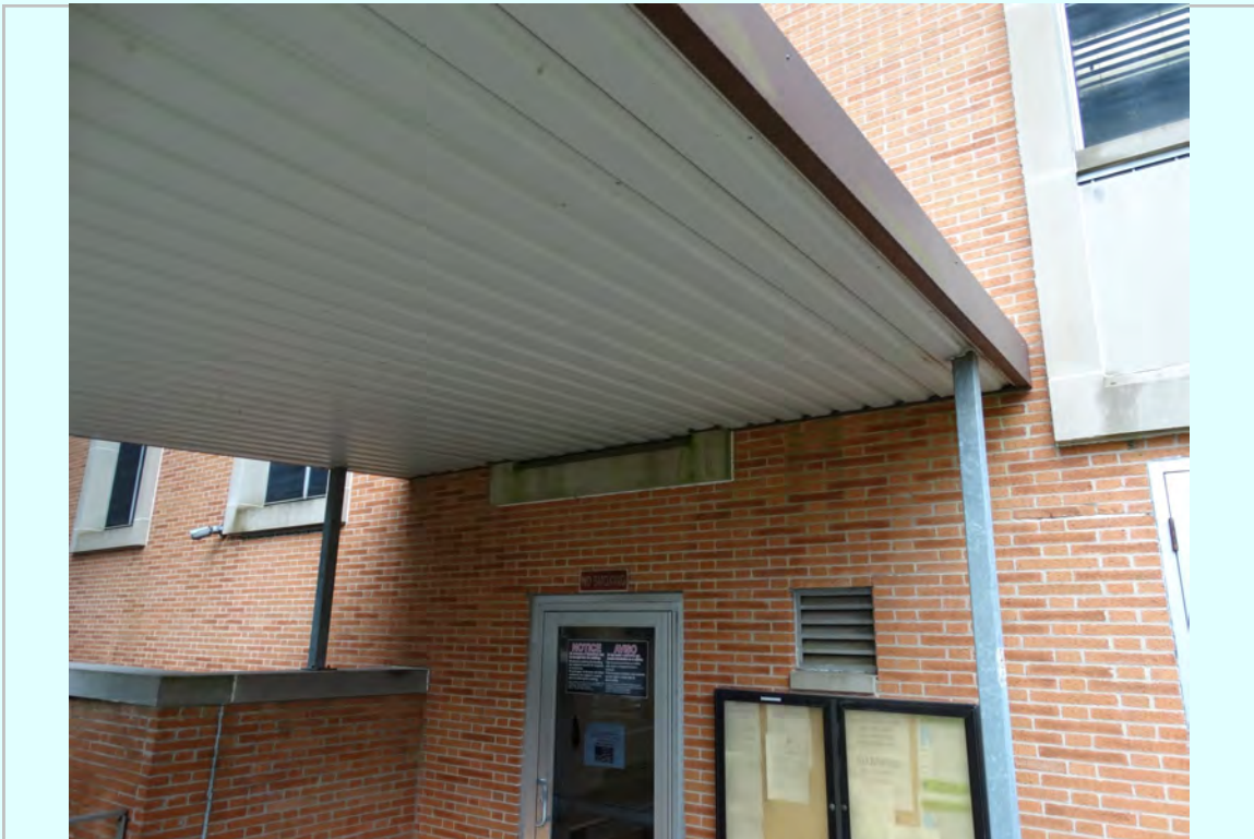
Photo: East Elevation, non original entry canopy, at window sill
