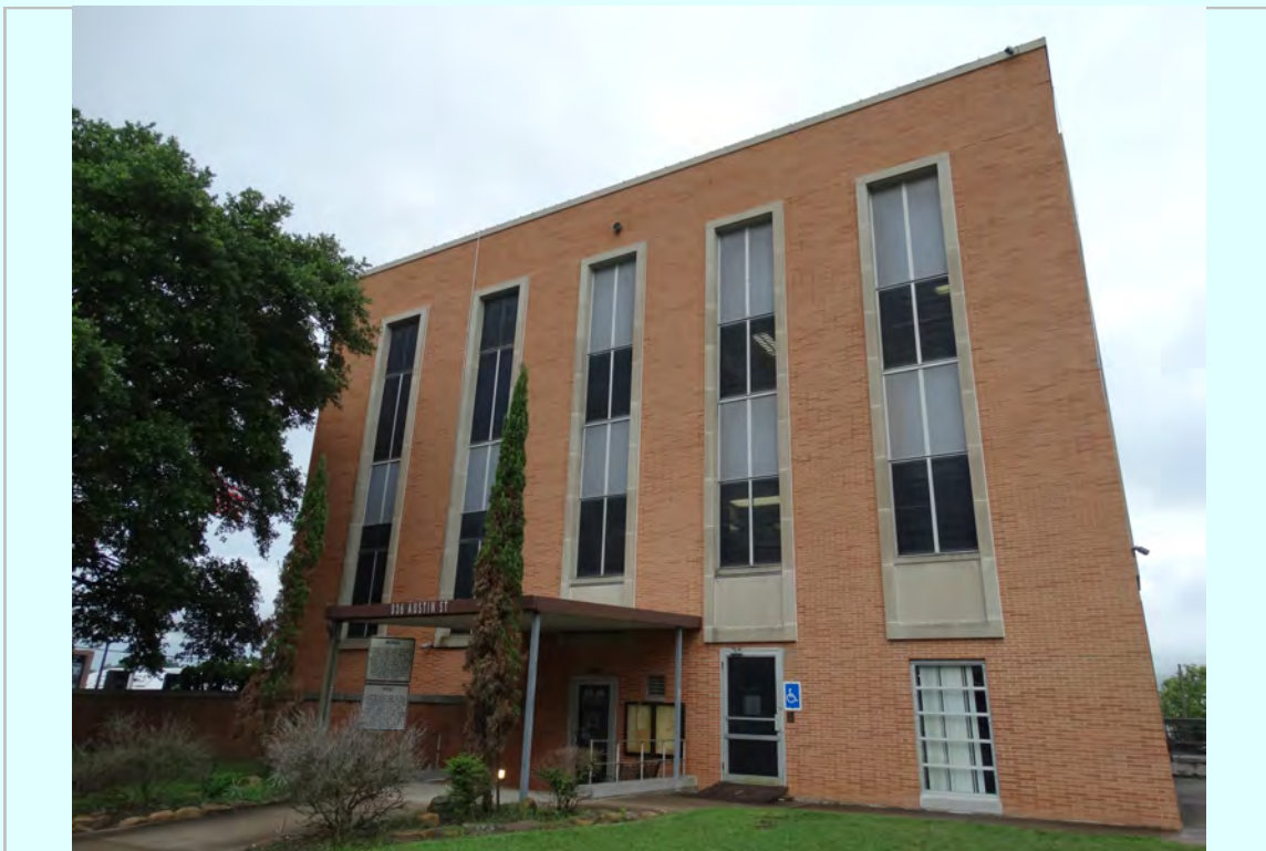
Photo: East Elevation
