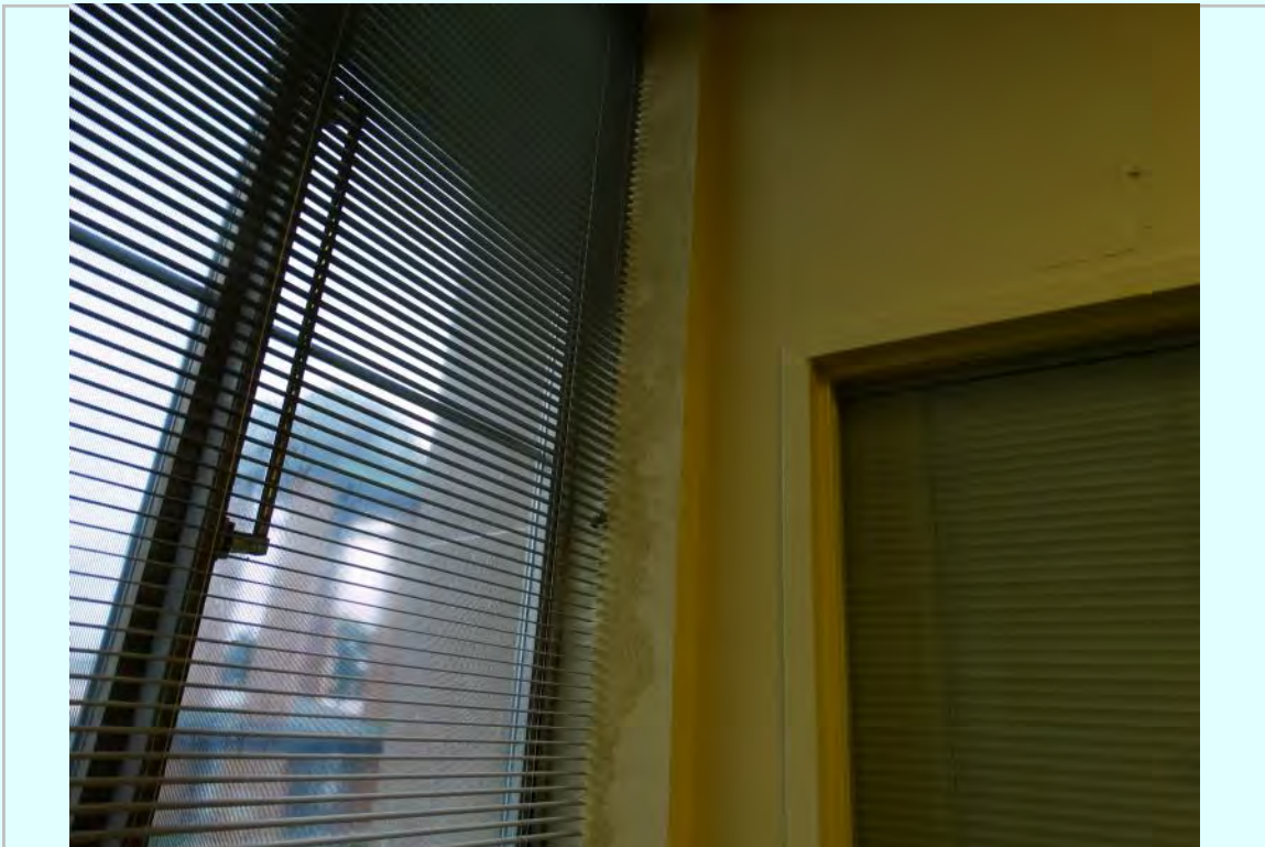
Photo: Mezzanine office, damage at window jamb
