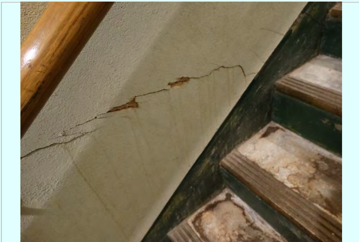
Photo: Fourth floor private stairs, plaster cracking
