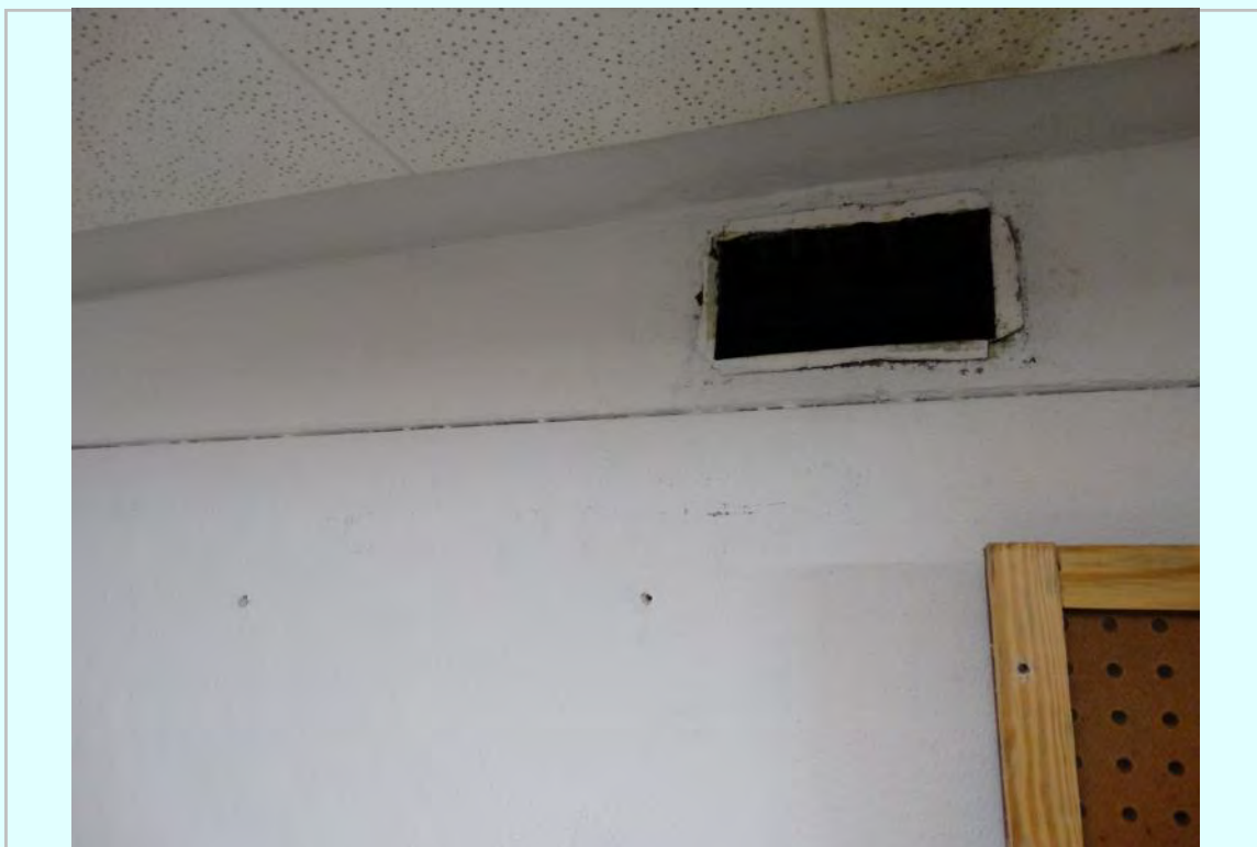
Photo: First floor office HVAC improper supply vent, missing grille
