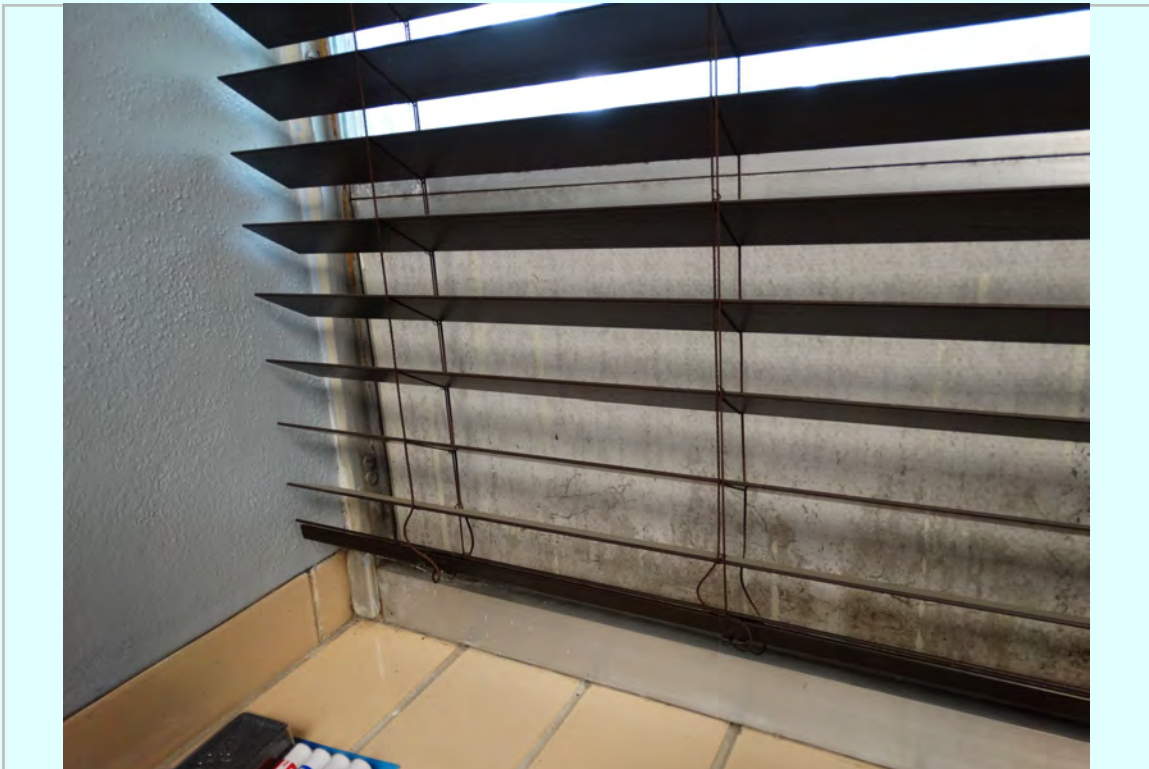
Photo: 1st floor window existing condition
