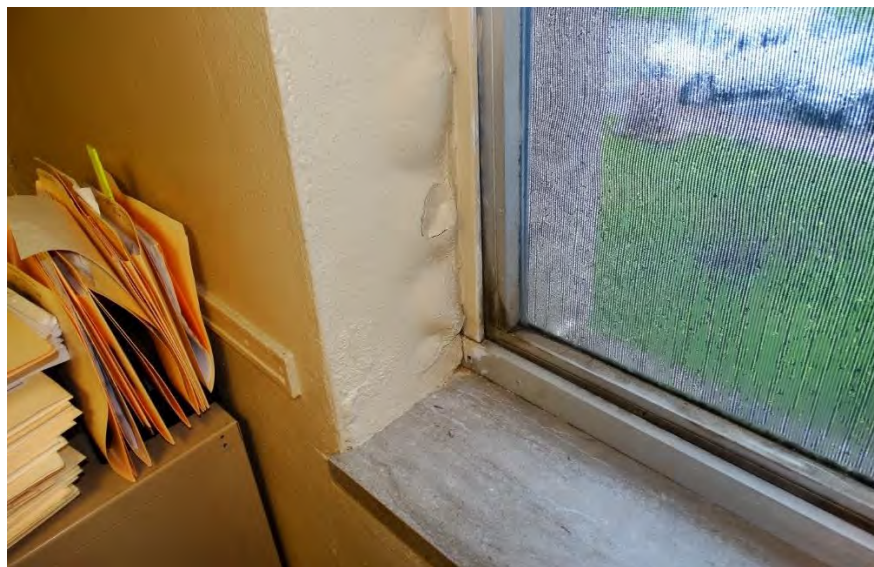
Figure 43. Existing moisture damage at County Clerk office
