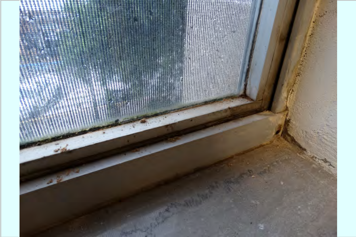
Photo: 3rd floor existing window condition
