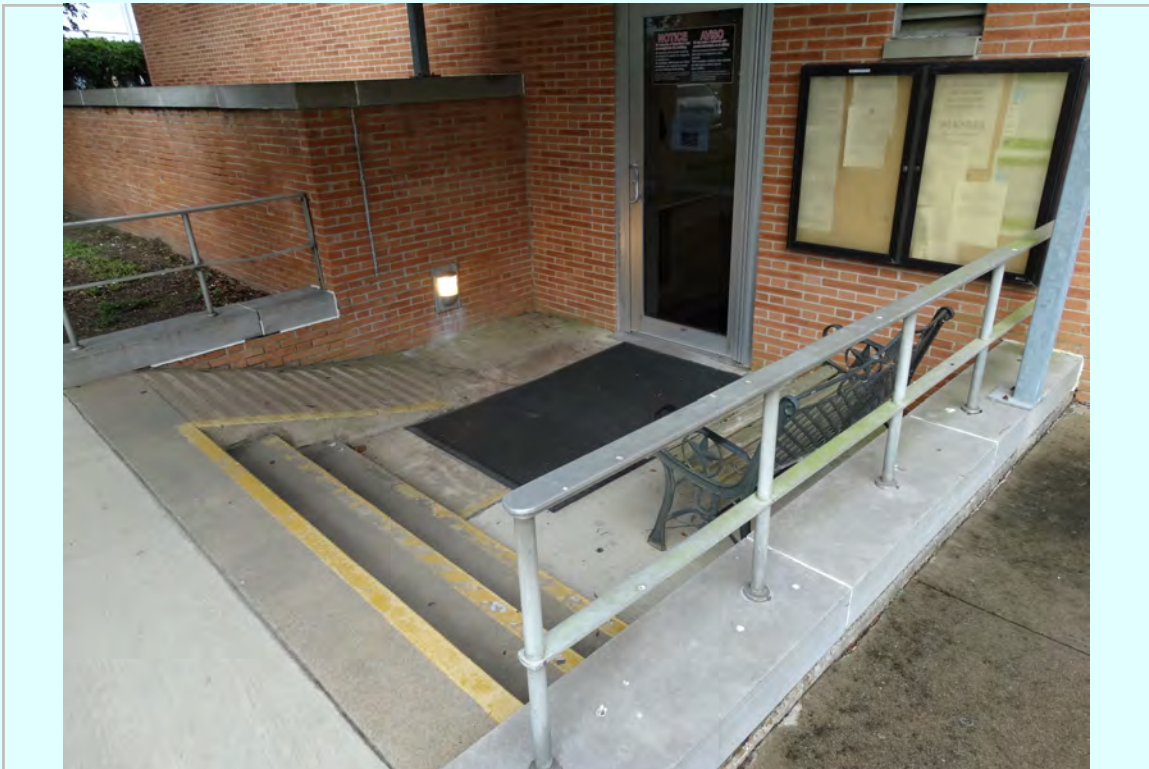
Photo: East elevation aluminum and glass door
