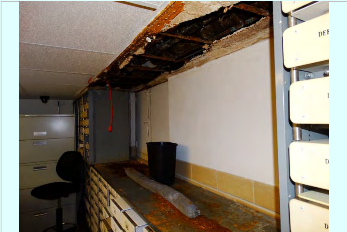
Photo: Storage space below County Clerk , ceiling damage, from moisture
