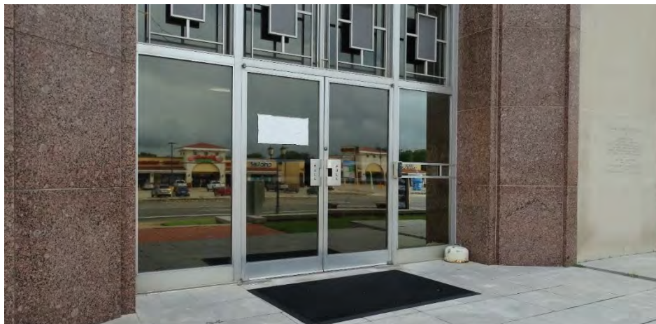
Figure 28. Existing south entry doors
