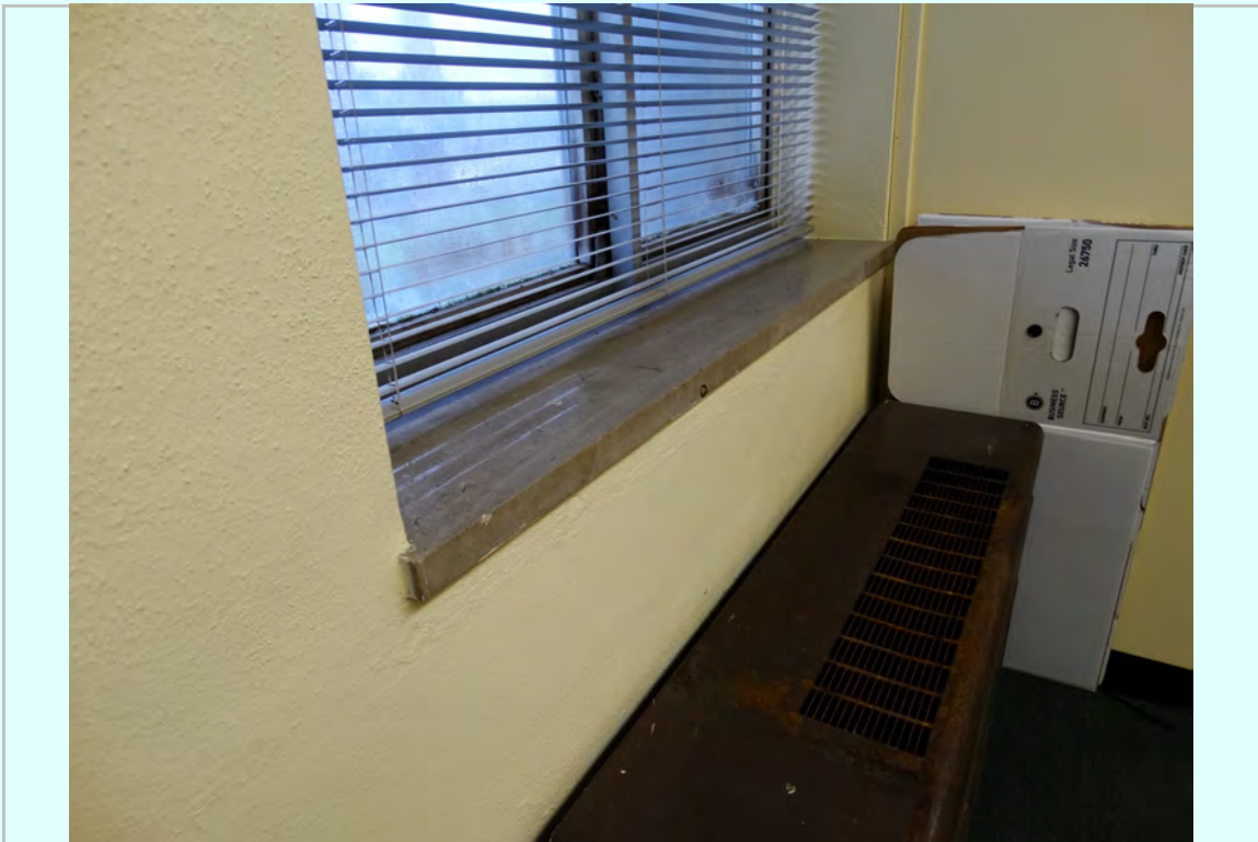
Photo: 2nd floor window existing condition, stone stool
