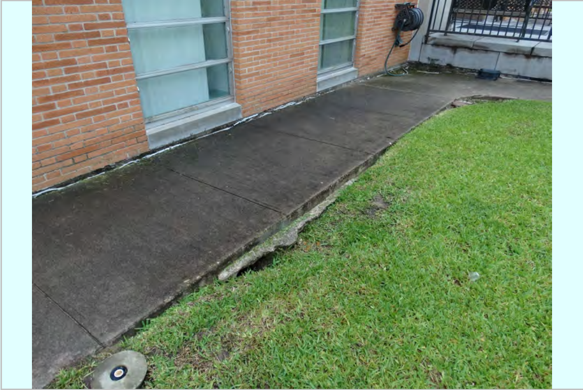
Photo: North Elevation ground floor windows and site erosion
