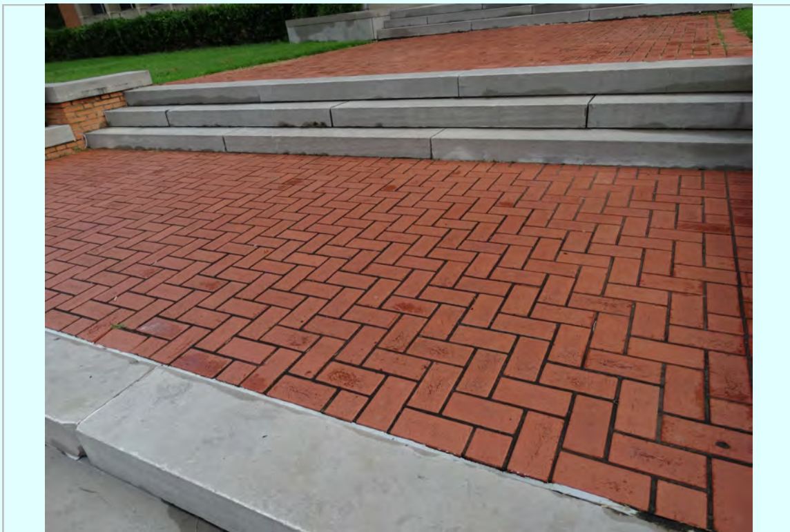
Photo: South entry clay pavers condition
