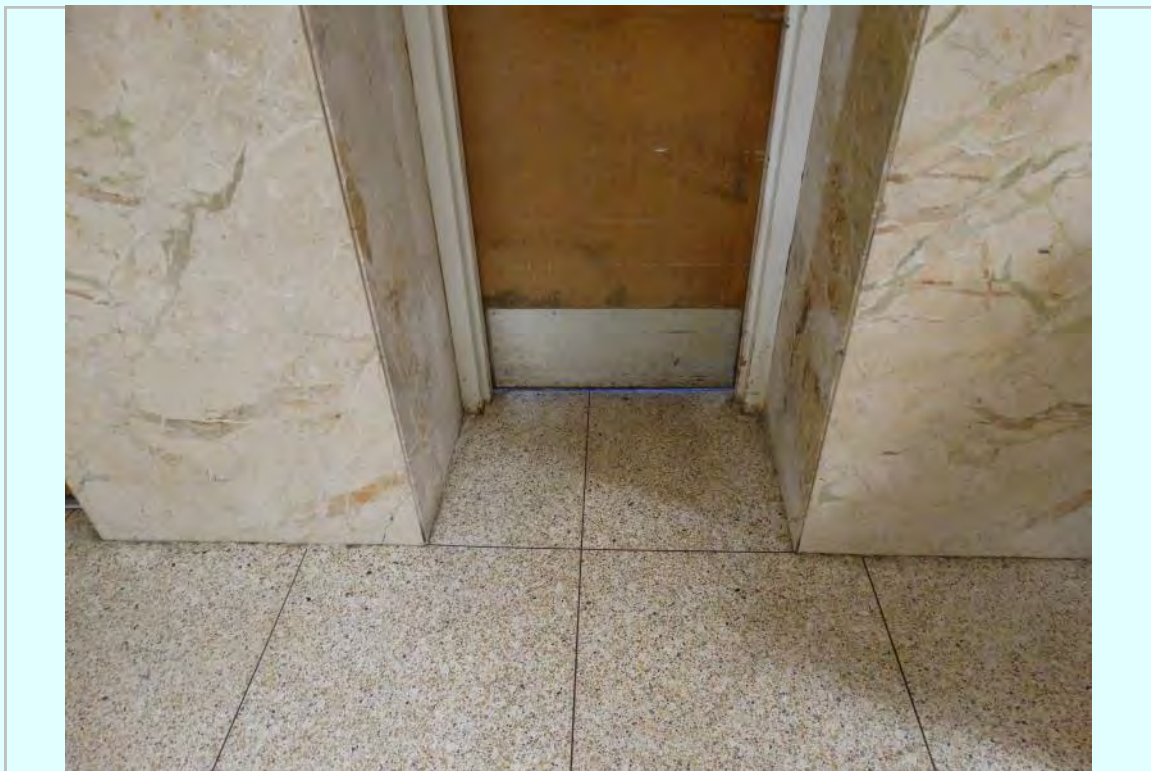
Photo: Third floor corridor
