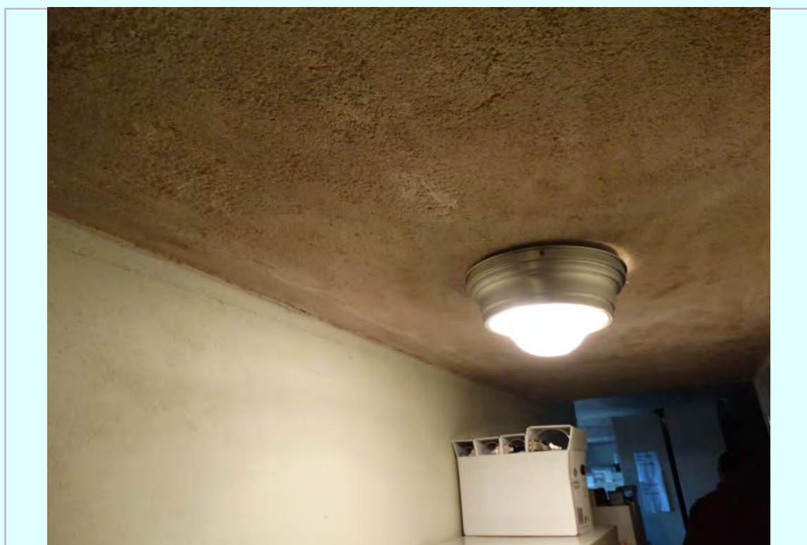
Photo: Fourth floor corridor typical light fixture
