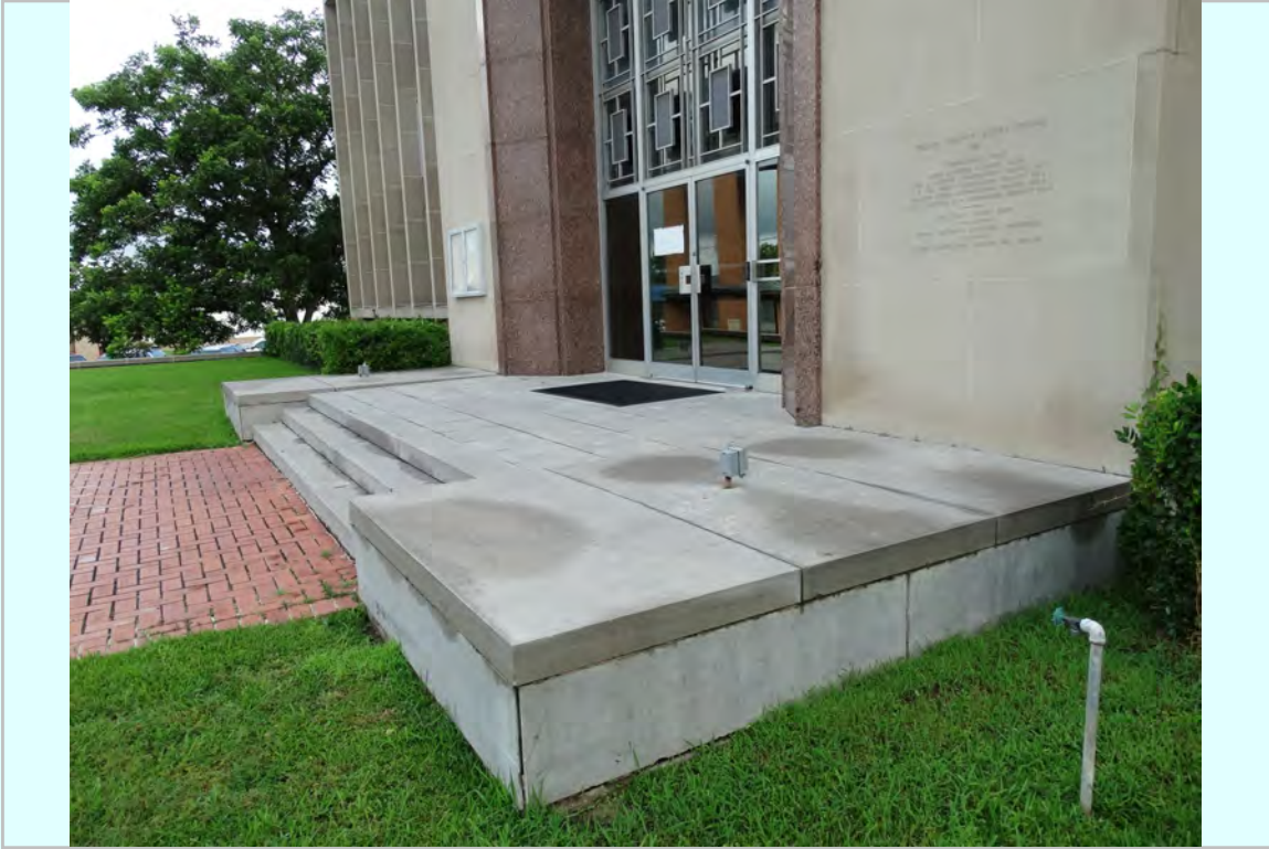
Photo: South entry patio stone condition
