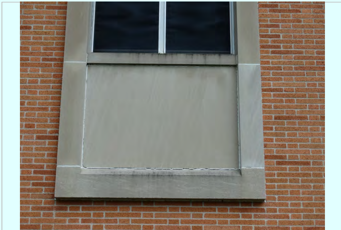
Photo: East Elevation, spandrel panel, assumed original, failing masonry joints
