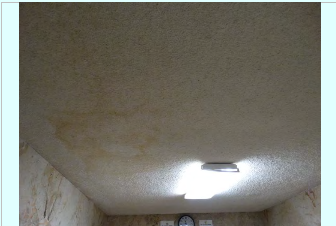
Photo: Third floor corridor ceiling damage and staining
