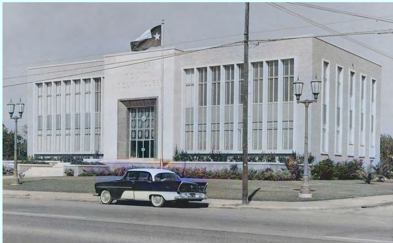
Photo: Photo of 1955 courthouse in construction, circa 1958
