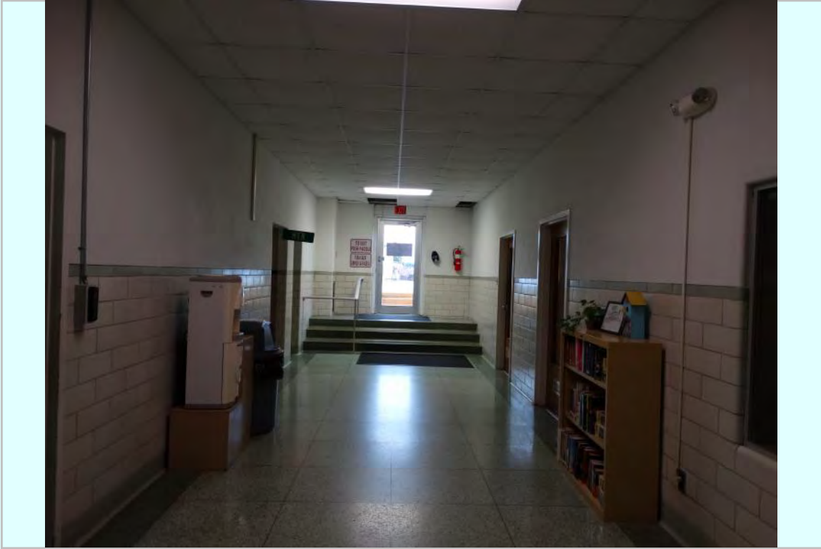
Photo: First floor corridor
