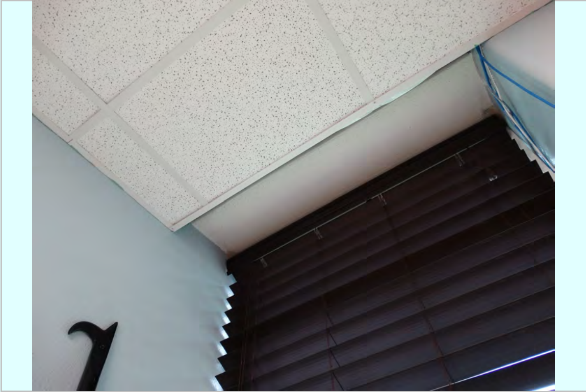
Photo: 1st floor window existing condition
