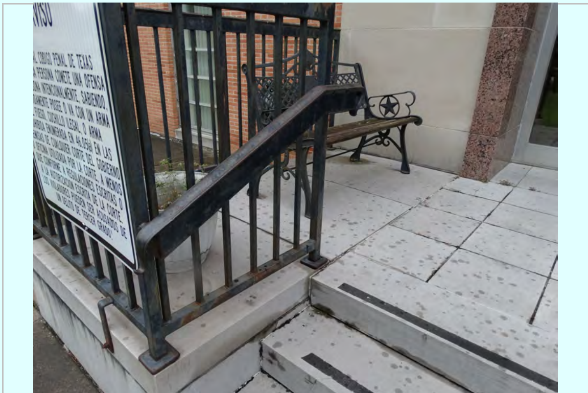
Photo: North Entry , non compliant railing
