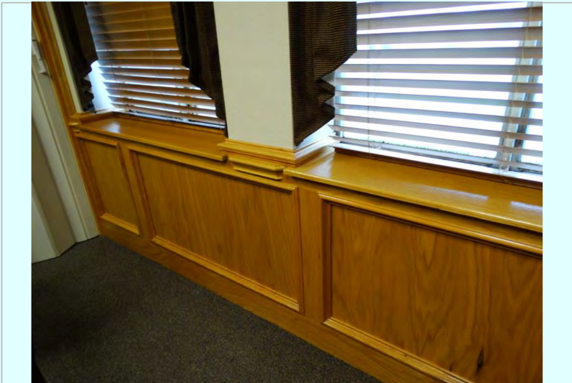
Photo: Third floor office space, non original millwork
