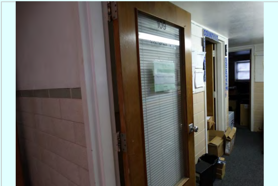
Photo: First floor office circulation space
