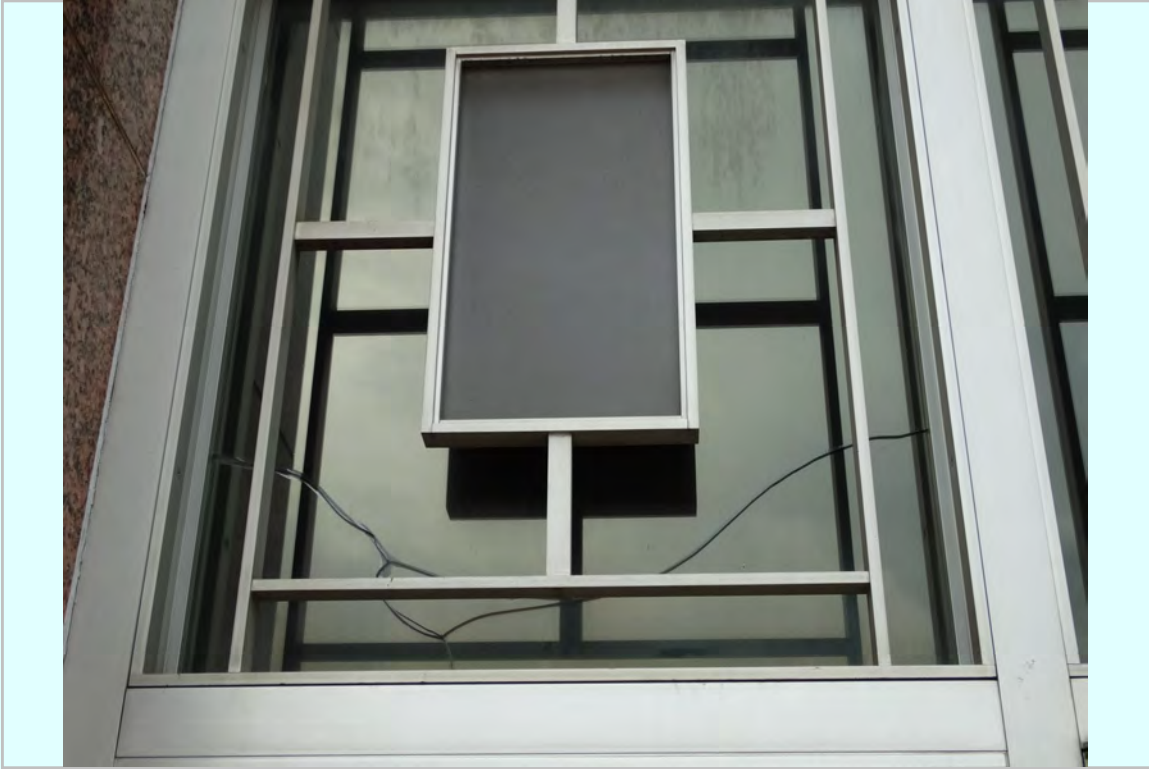
Photo: South Entry aluminum screen detailing
