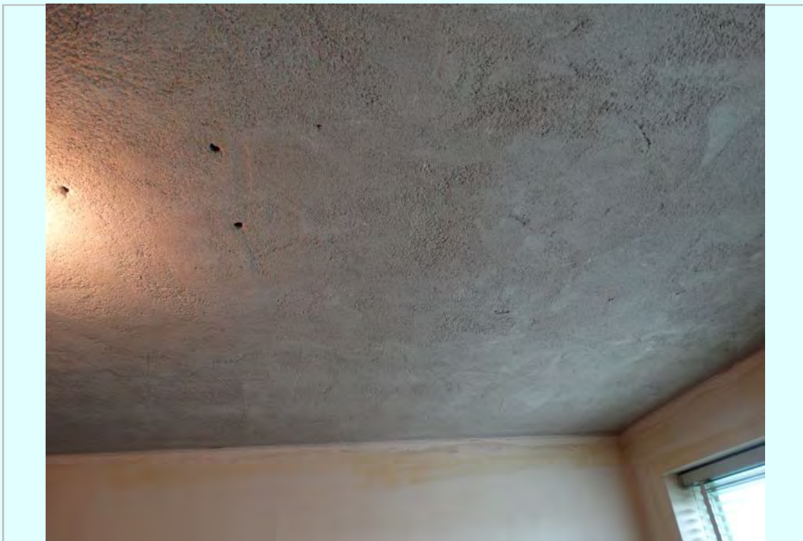
Photo: Fourth floor typical ceiling condition
