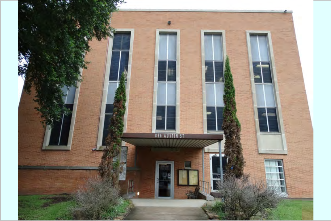
Photo: East Elevation, ground floor entry
