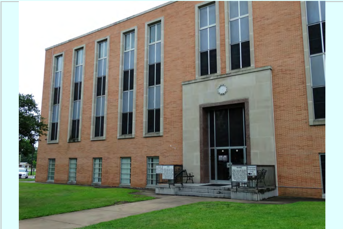
Photo: North Elevation
