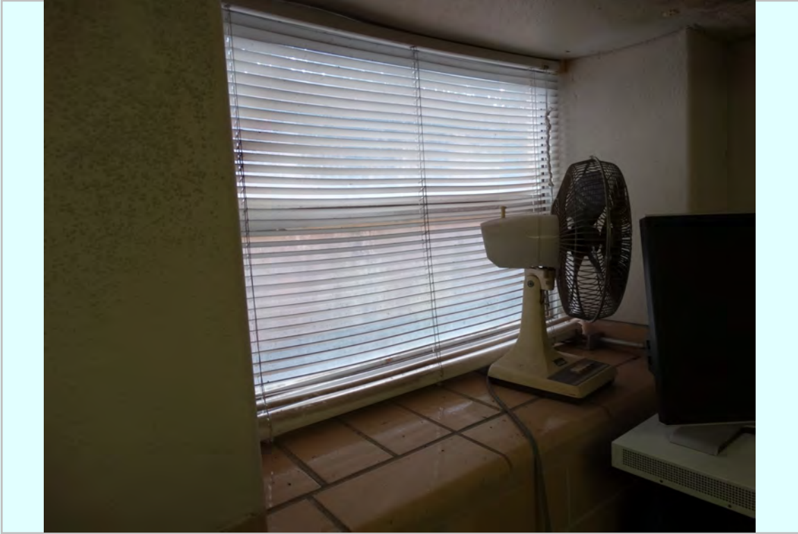
Photo: 1st floor window existing condition
