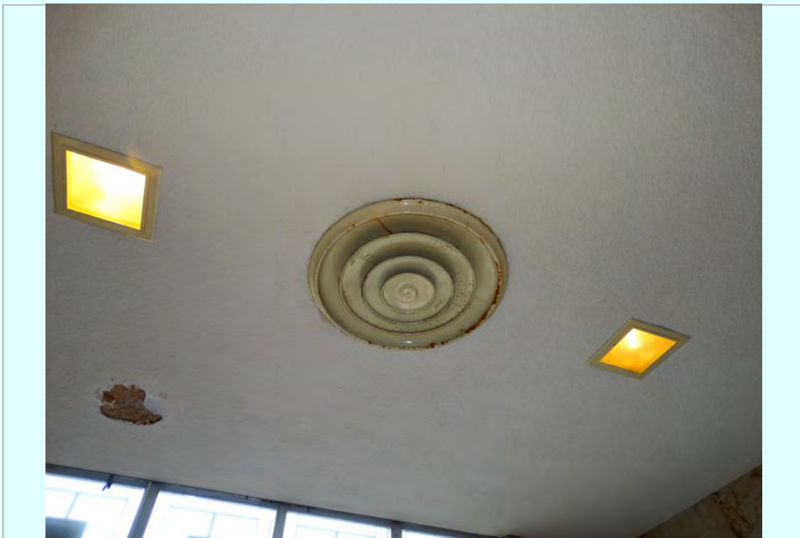
Photo: Mezzanine lobby ceiling, damage and supply vent rusting
