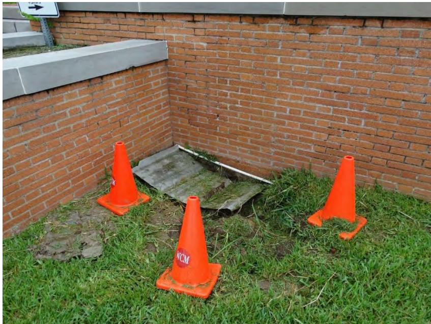
Figure 7. South lawn inside corner of cheek wall and east retaining wall, where there has been soil erosion
