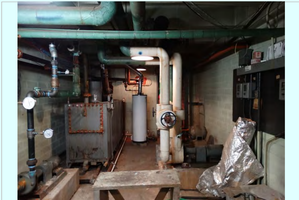
Photo: Fourth floor, mechanical space
