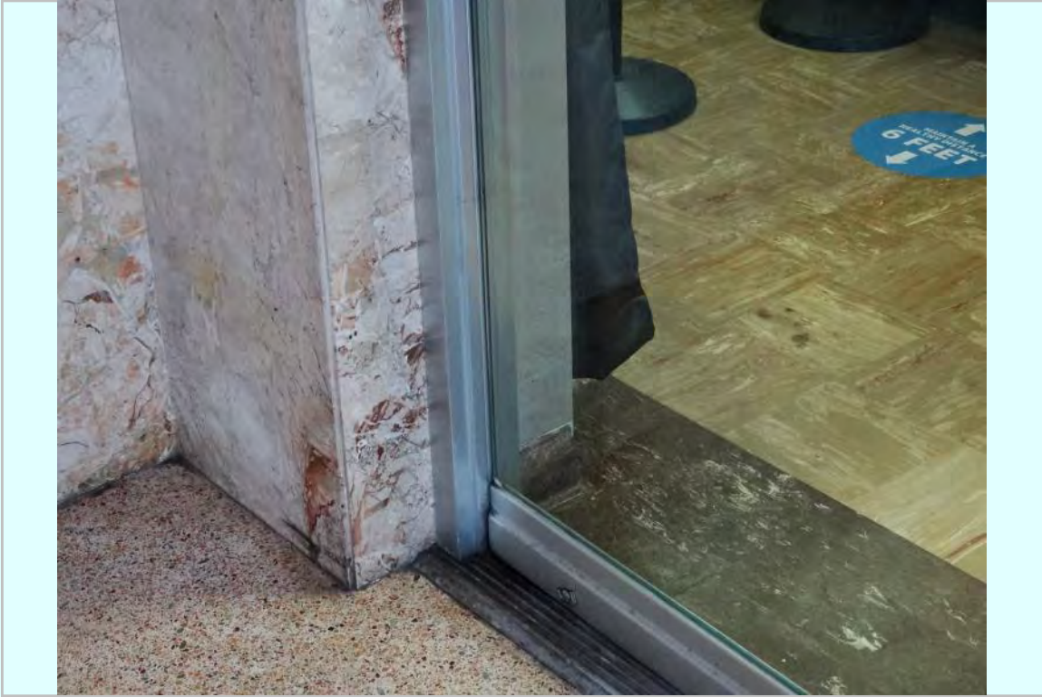
Photo: Mezzanine Level to County Clerk Office pivot door detailing
