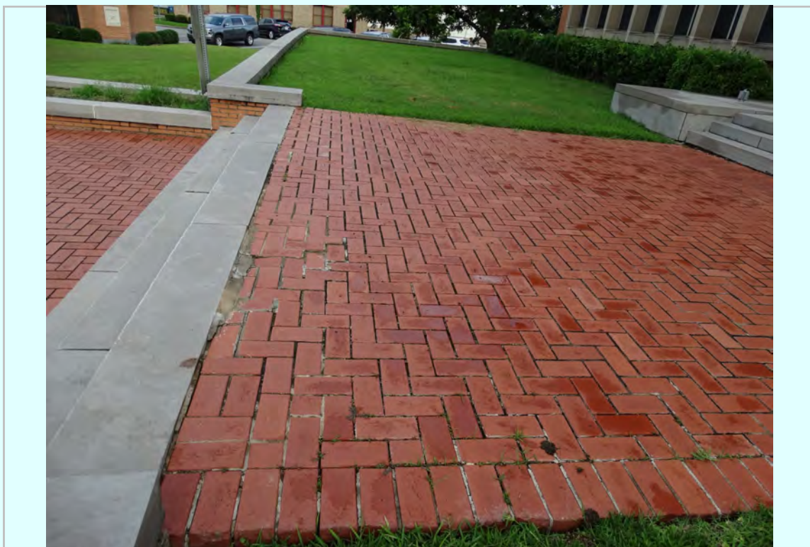
Photo: South entry clay paver existing condition
