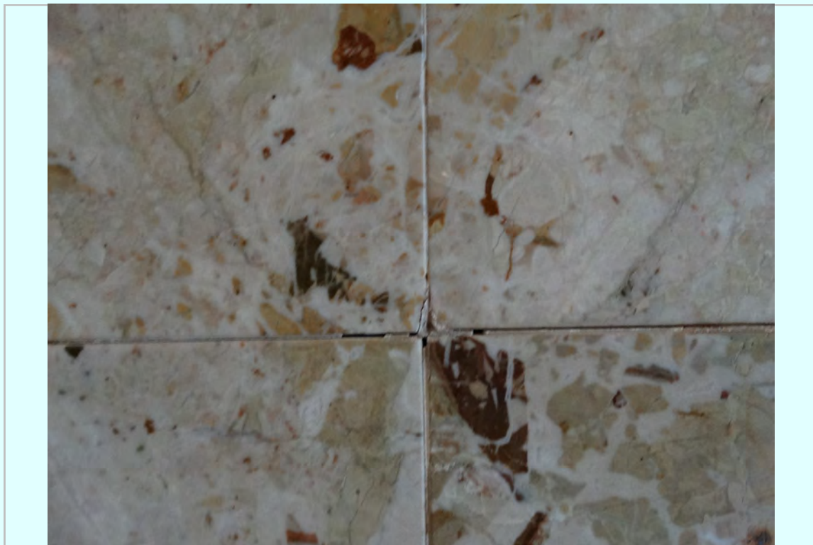
Photo: Typical stone condition at joints
