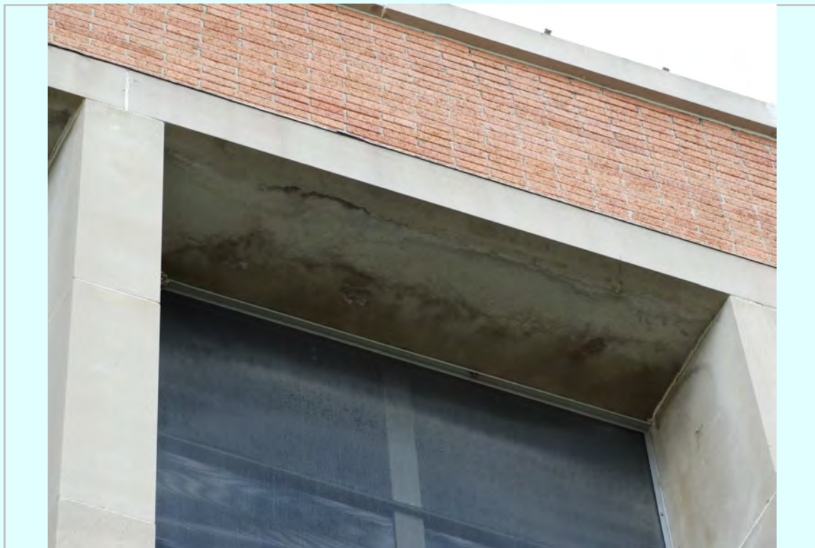
Photo: Typical screens and stone condition at curtain wall
