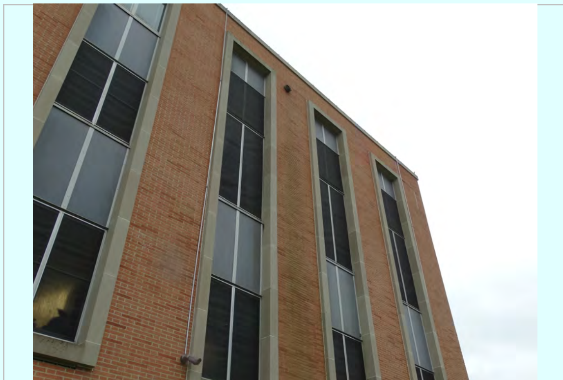
Photo: North Entry , moisture staining at masonry and biological growth, exposed conduit
