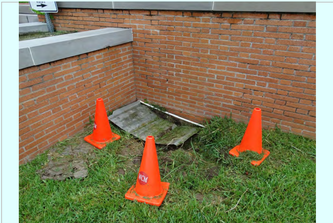
Photo: Site erosion/drainage pot hole
