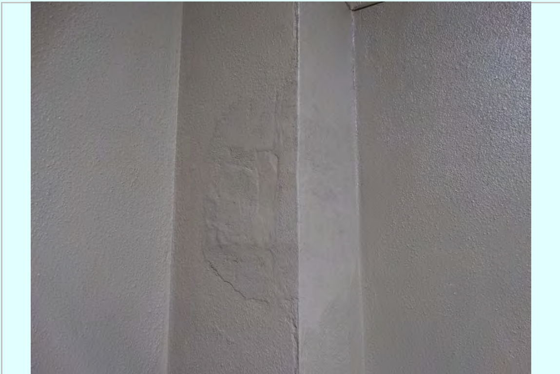
Photo: County Clerk office wall damage and poor repairs
