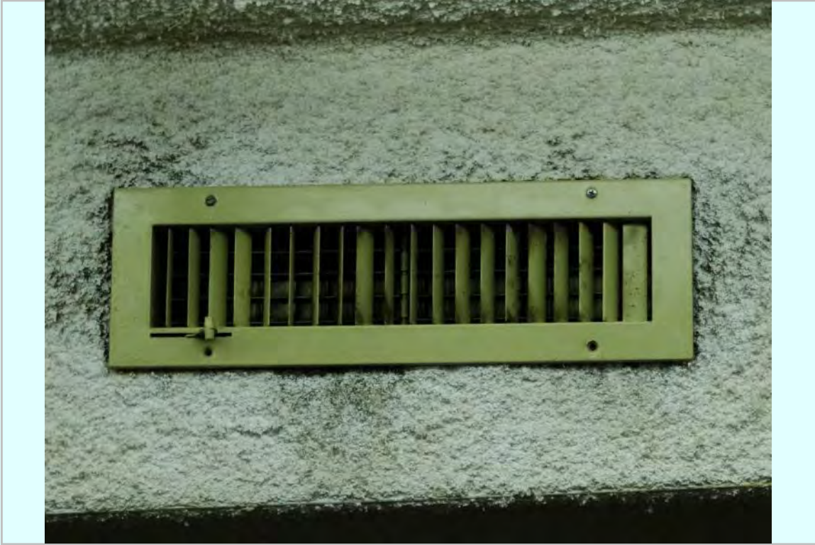
Photo: HVAC supply duct vent into County Court deliberation room
