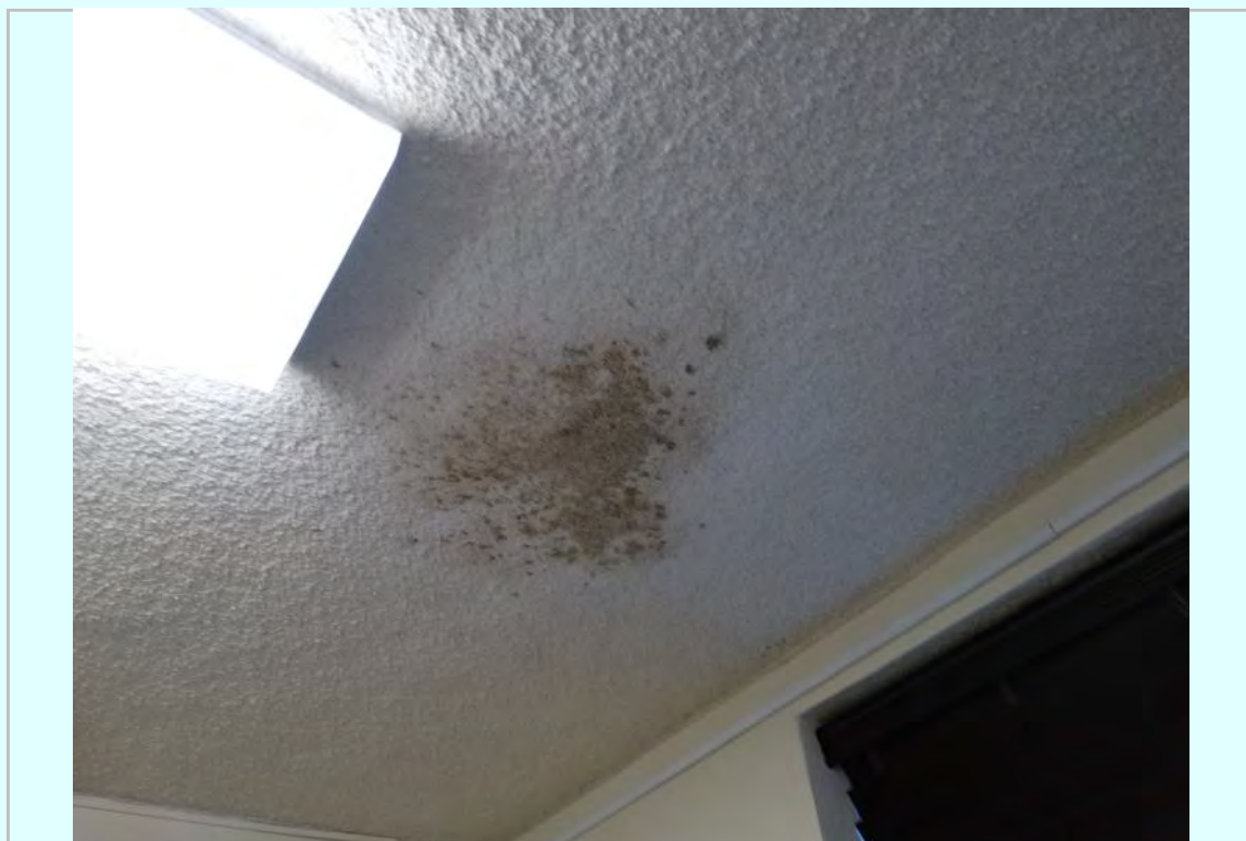
Photo: Third floor moisture damage at ceiling, biological growth
