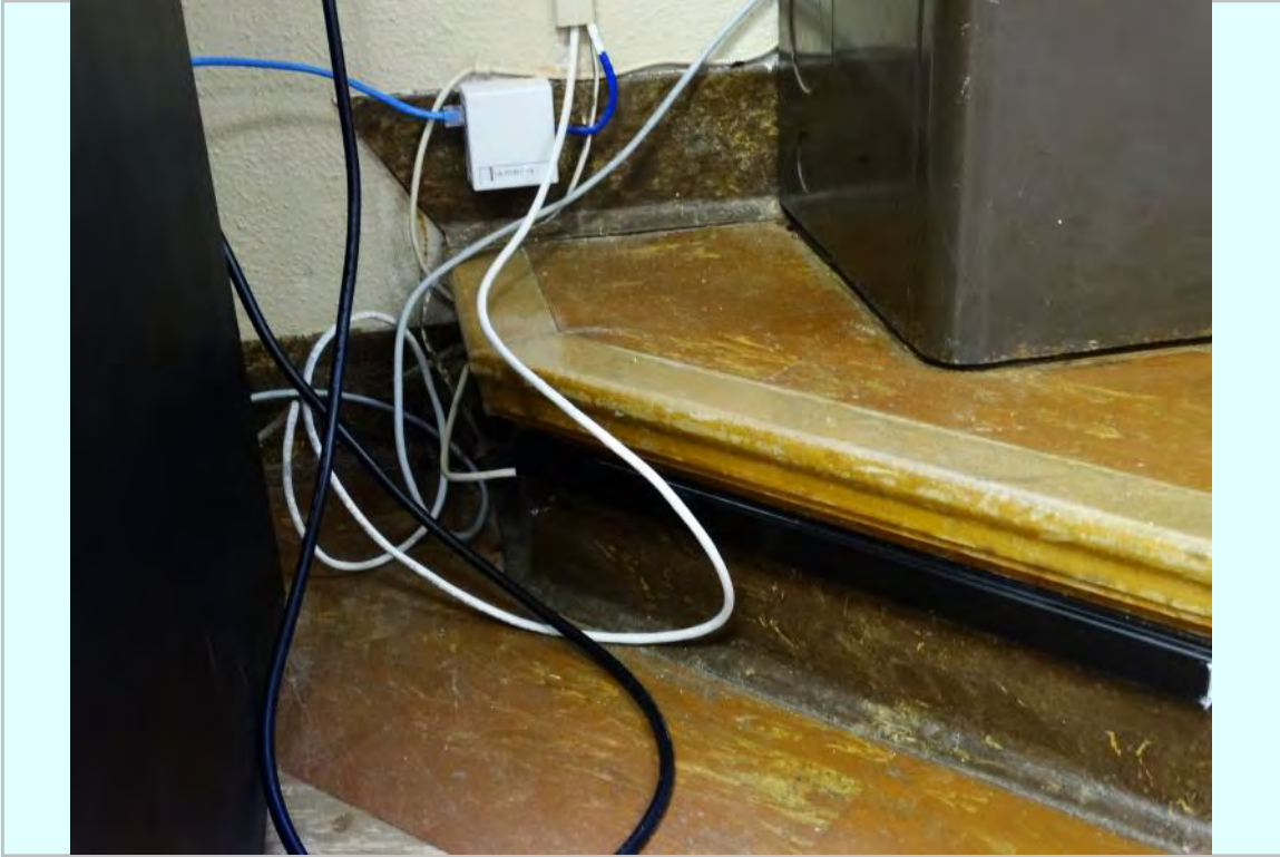
Photo: Second floor courtroom Commissioners Bench platform
