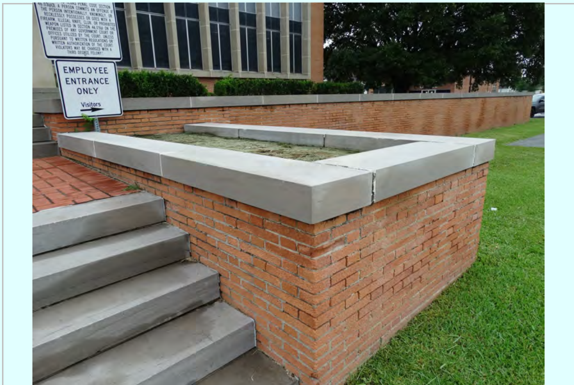
Photo: South entry retaining wall planters, coping joints failing and mortar deterioration
