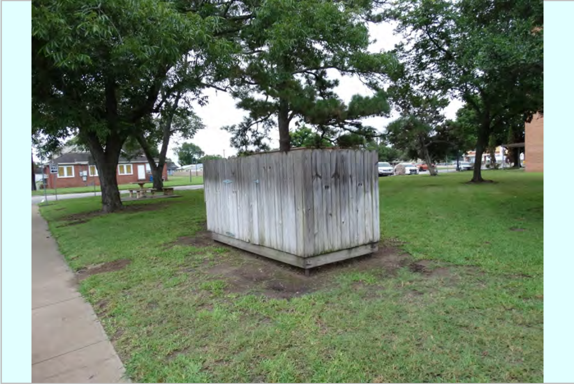
Photo: Wood utility yard fencing
