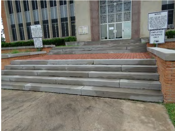
Figure 4. (Left) South walkway entrance with limestone steps and clay pavers. Figure 5. (Right) South walkway entrance masonry cheek wall with planter
