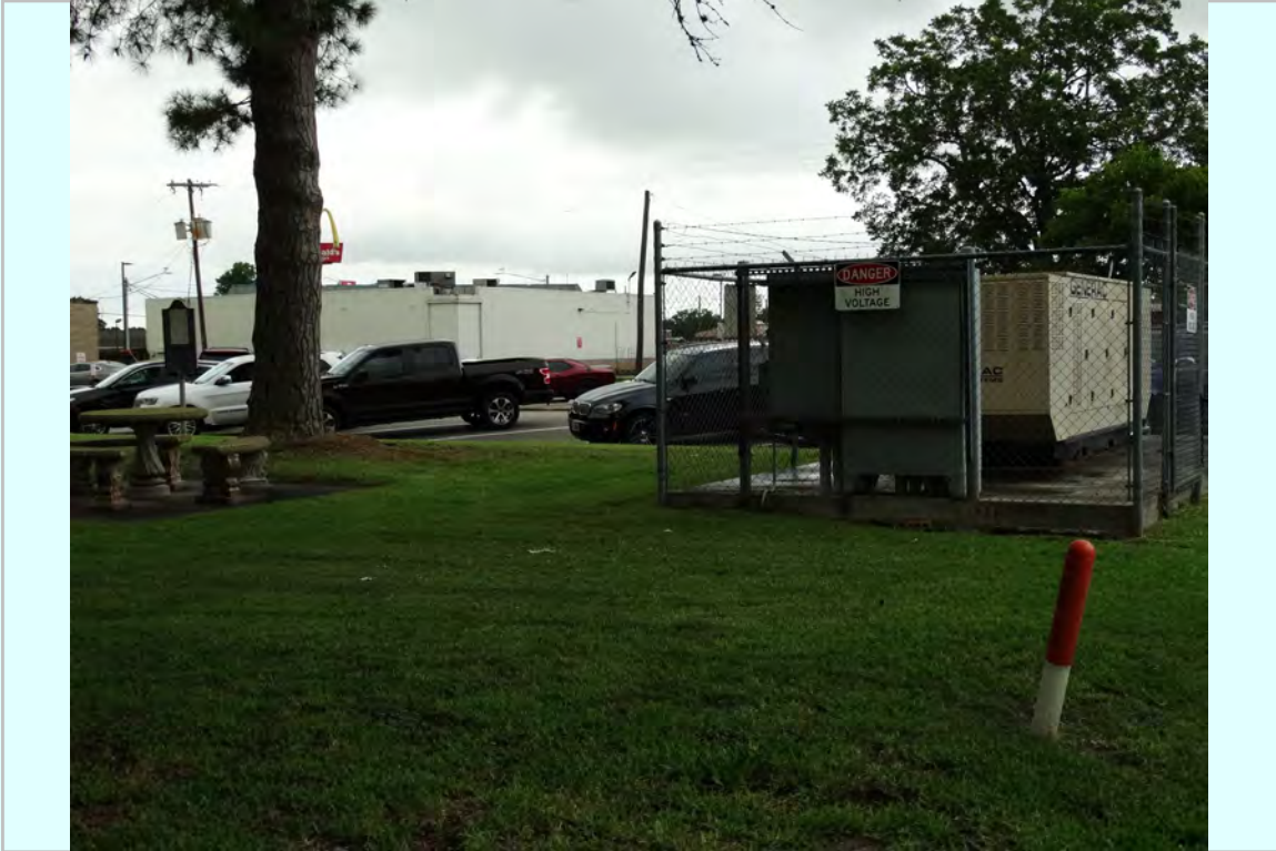
Photo: Mechanical Yard at north west corner of square
