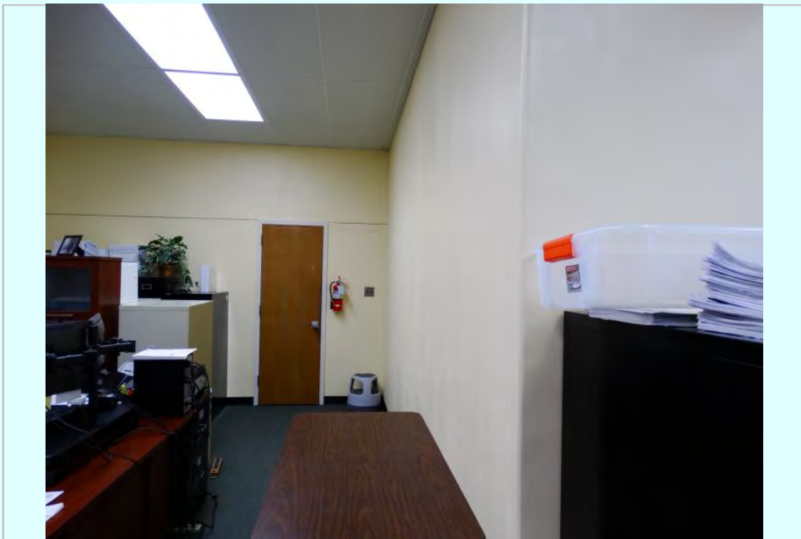
Photo: Mezzanine office space
