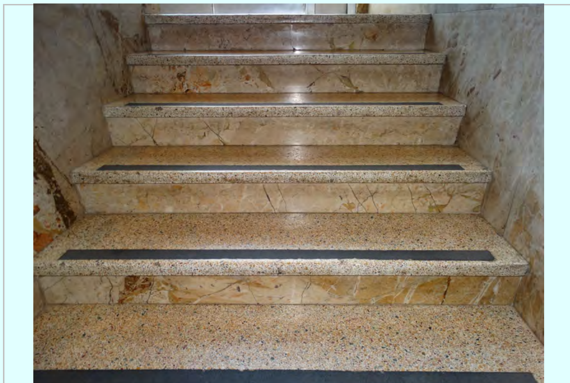
Photo: Typical riser and tread condition at central stair
