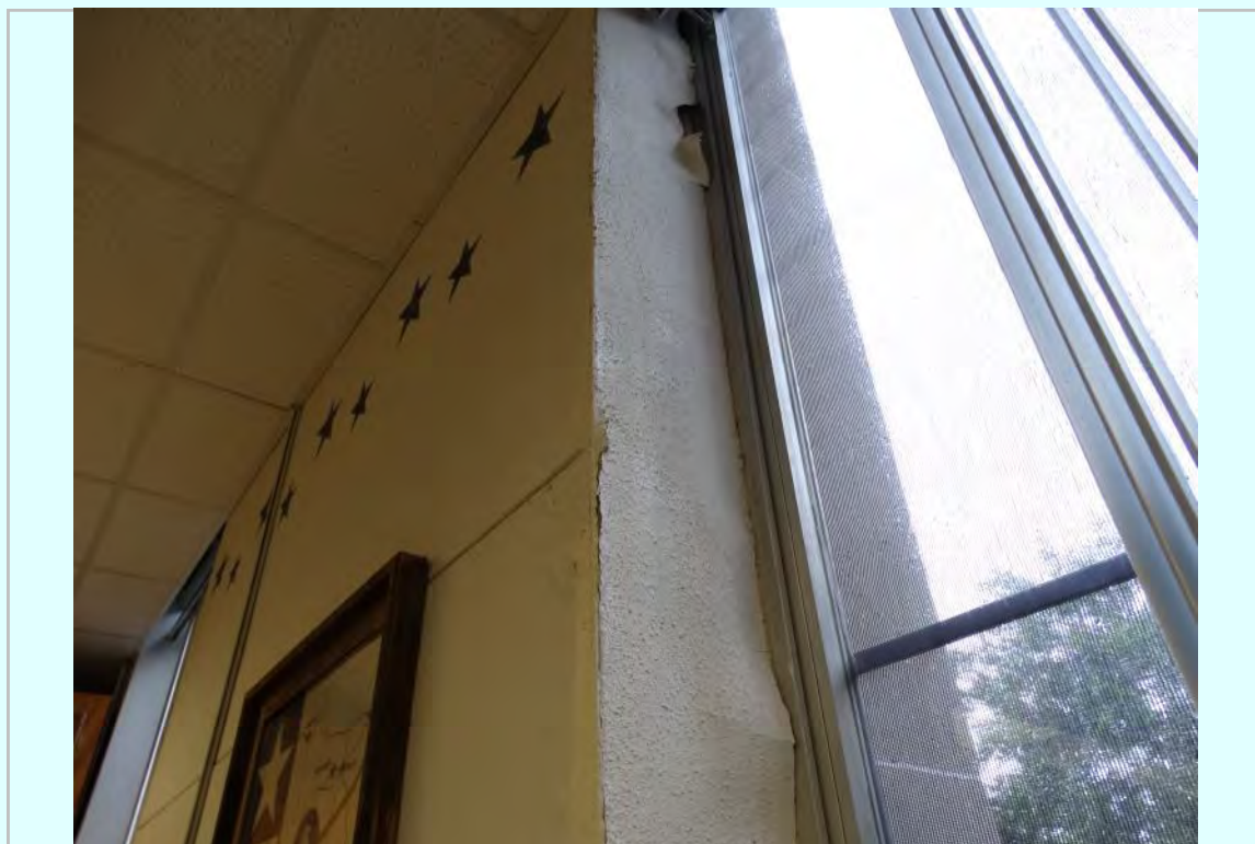
Photo: Third floor district clerk space, damage at windows, spalling and cracking
