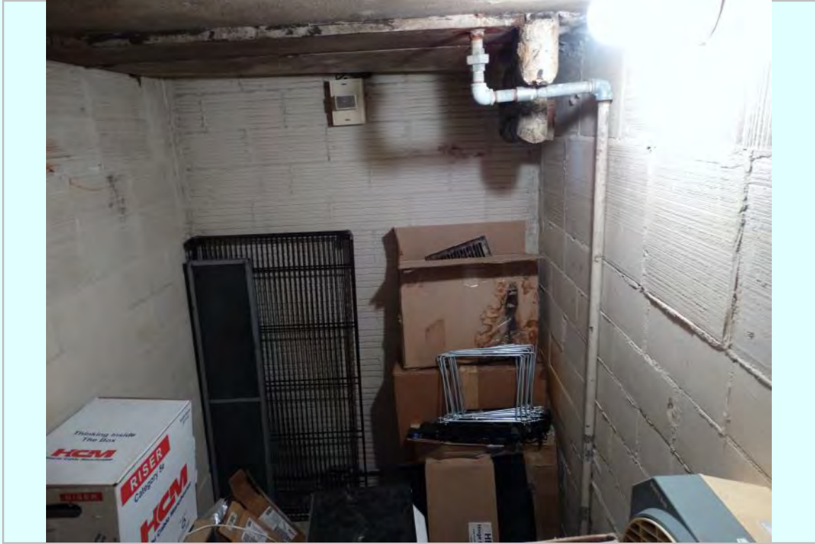
Photo: First floor storage
