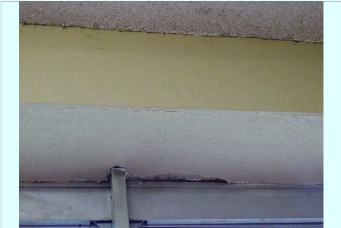
Photo: County Courtroom jury deliberation room damage at windows and soffit
