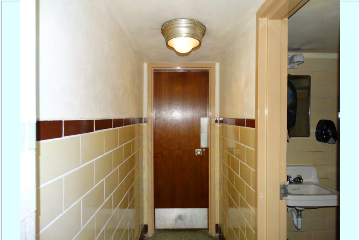
Photo: Non-compliant entry into public restrooms on ground floor
