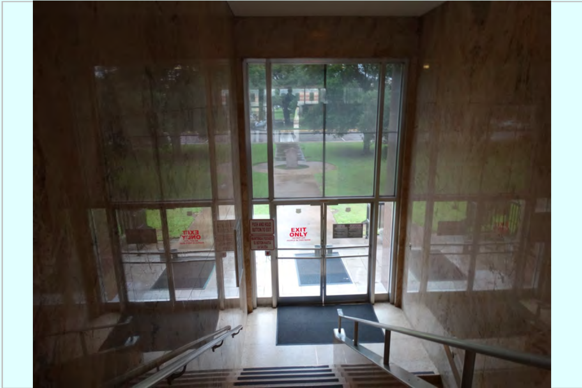
Photo: North elevation curtain wall from interior
