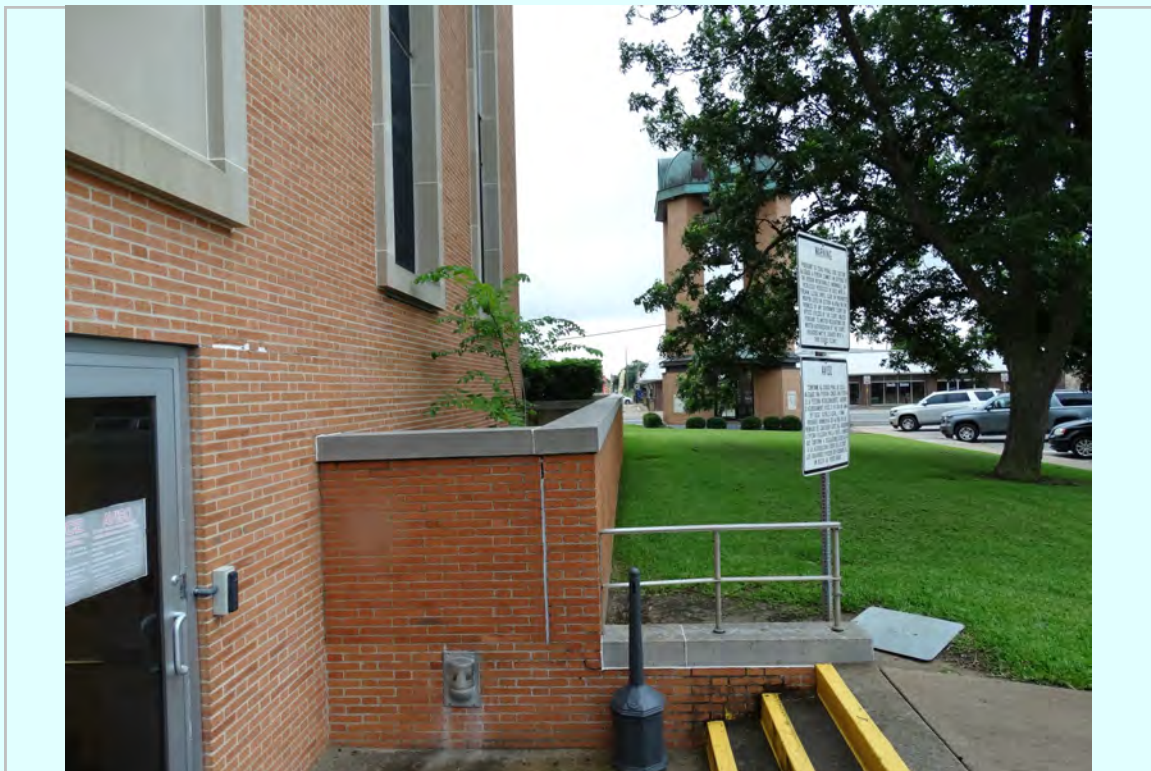
Photo: West Elevation, retaining wall
