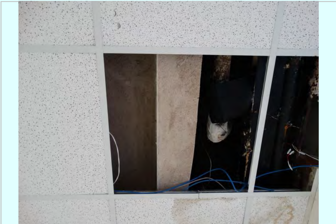
Photo: First floor plenum and original structure
