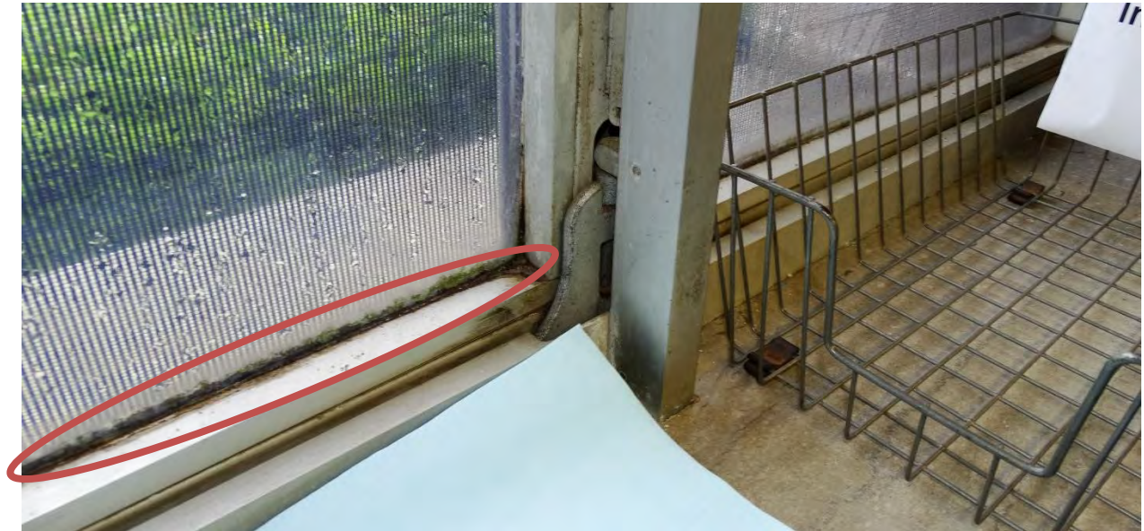
Figure 30. staining and biological growth at lower window sash
