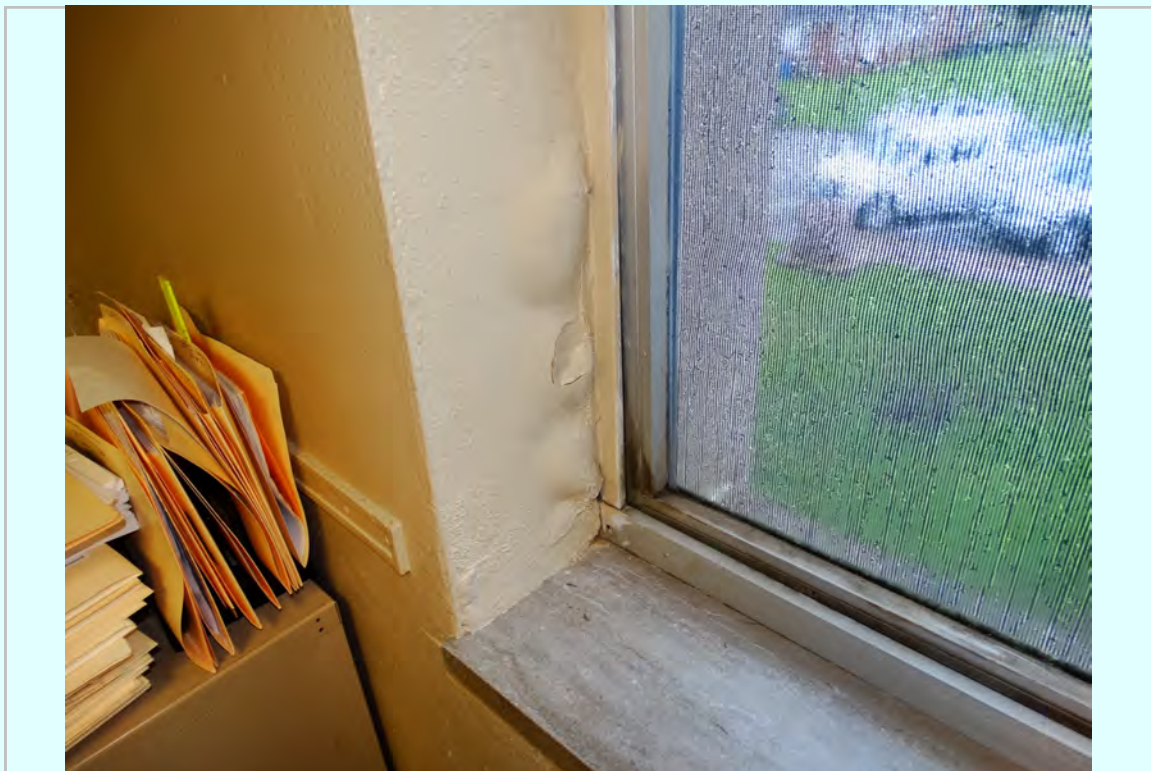
Photo: 2nd floor window existing moisture intrusion
