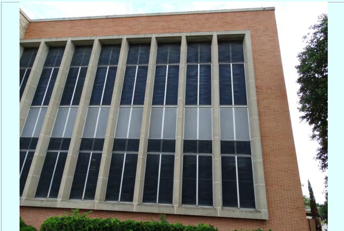
Photo: Typical Curtain walls at North and South elevations
