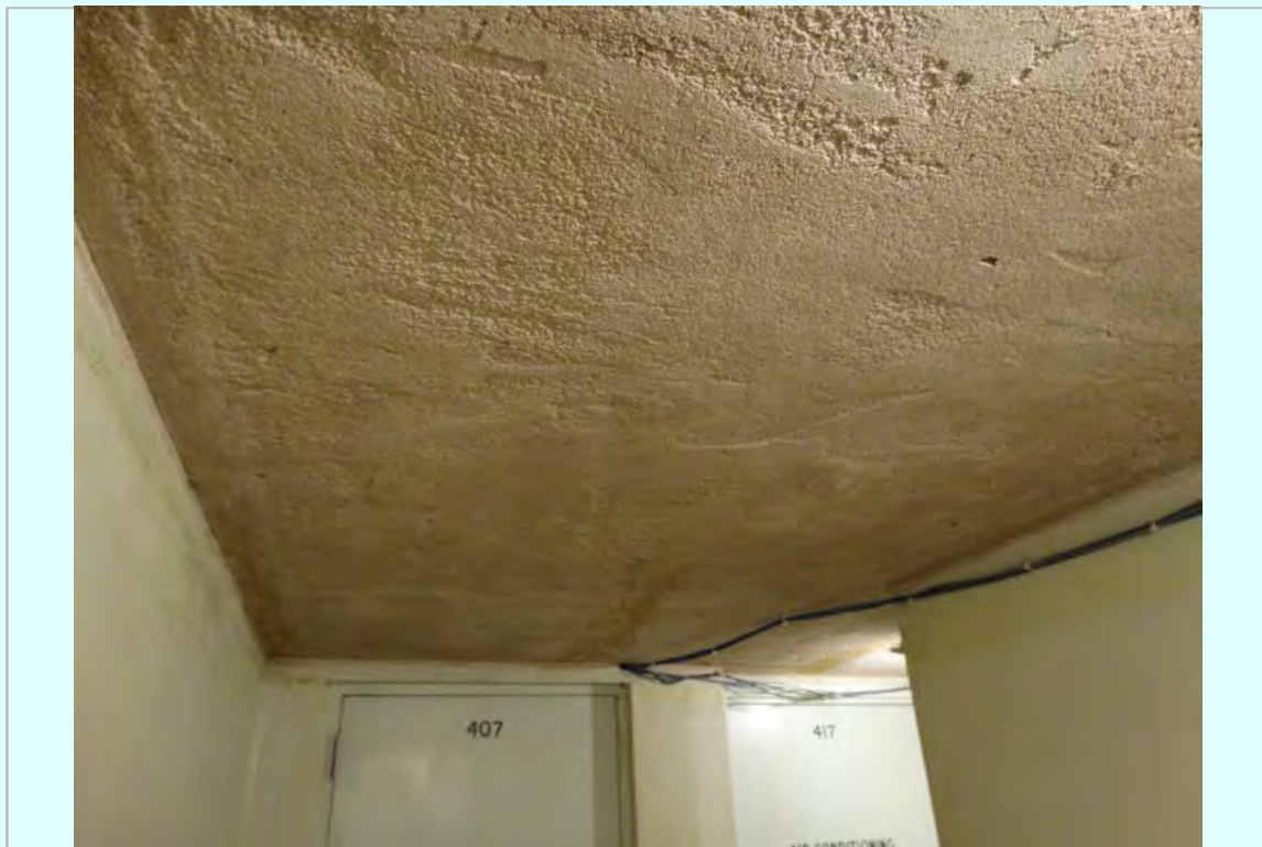
Photo: Fourth floor corridor typical ceiling condition
