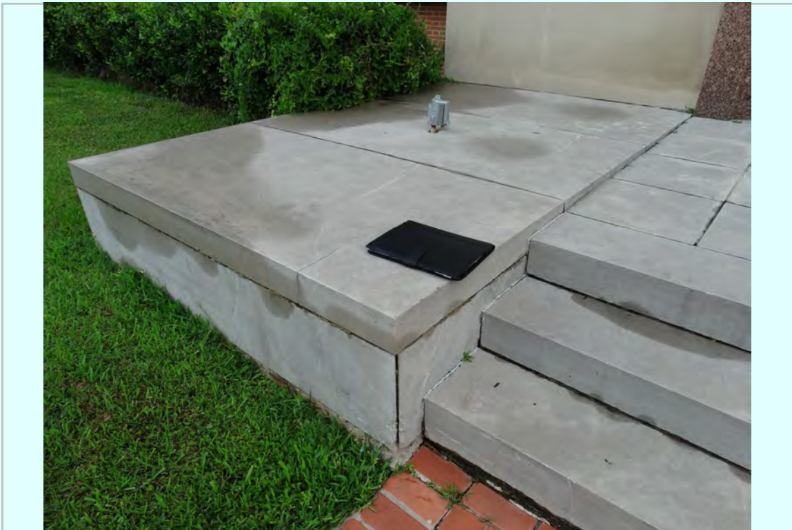
Photo: South entry patio stone joints failing and moisture staining and cracking
