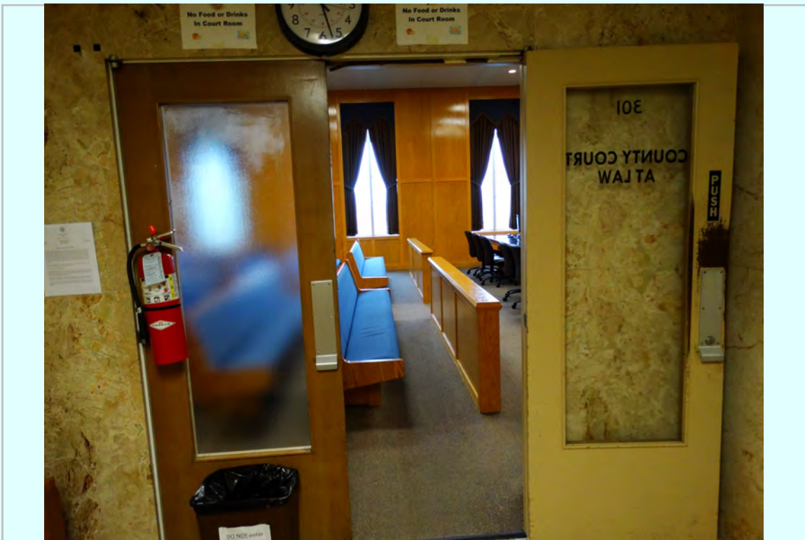
Photo: Non-compliant door
