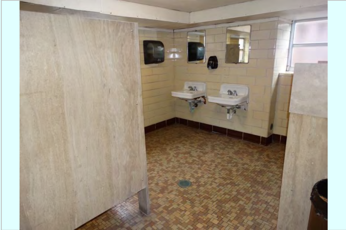
Photo: First floor typical restroom
