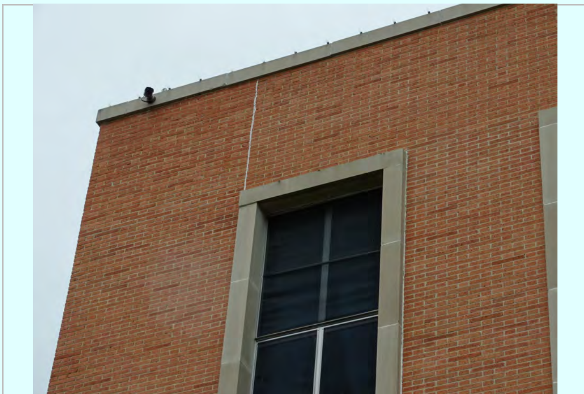
Photo: West Elevation, masonry control joint, discolored clay bricks
