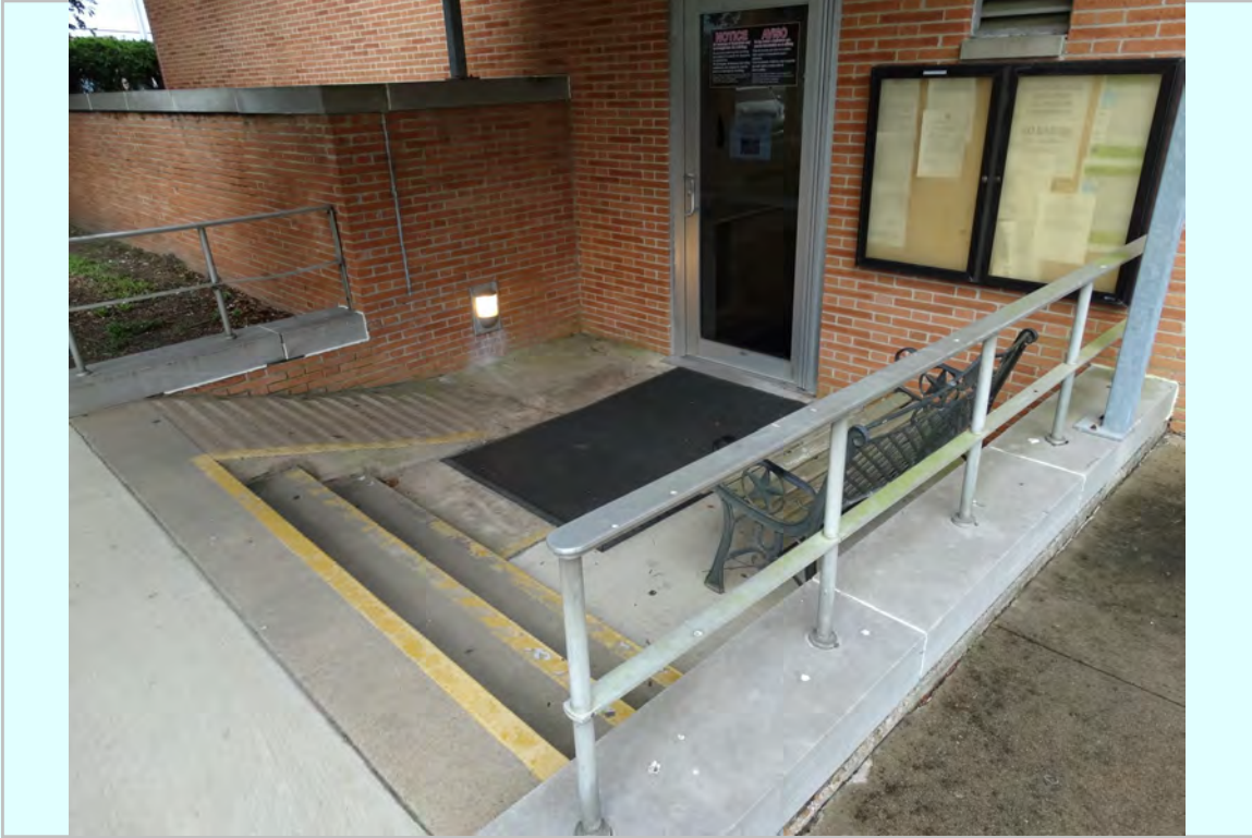
Photo: East Elevation, ground floor entry
