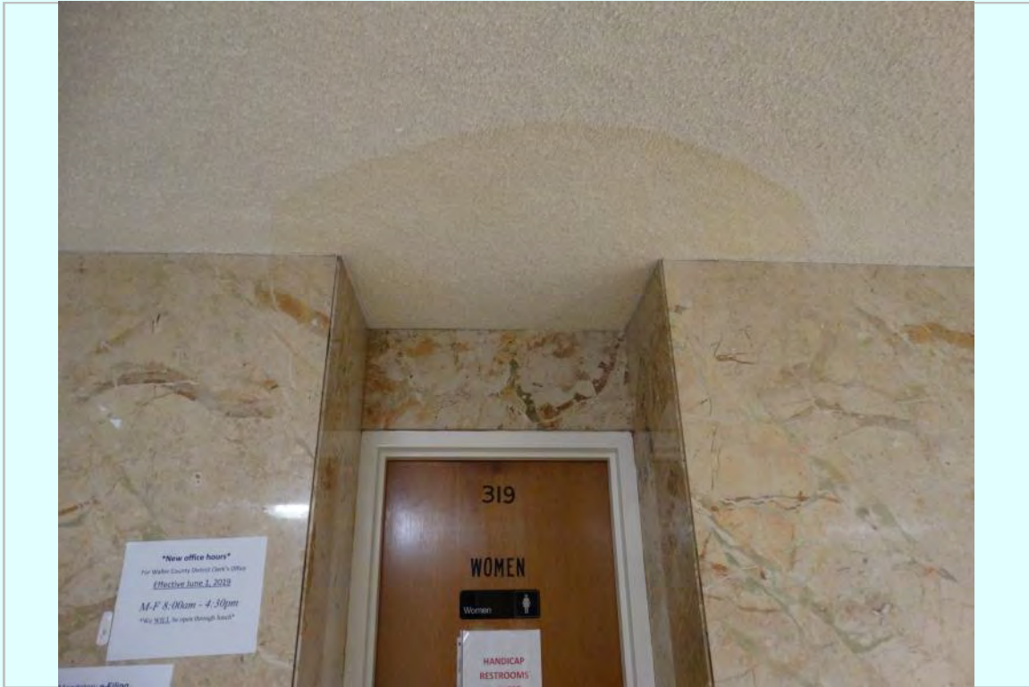
Photo: Third floor corridor moisture damage at ceiling
