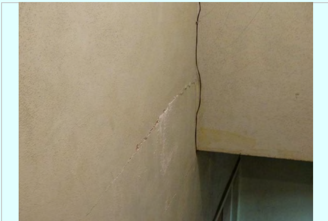
Photo: Fourth floor private stairs wall plaster cacking
