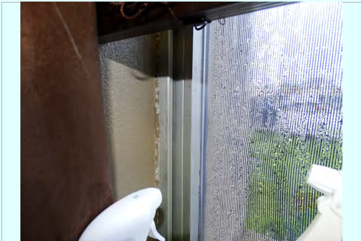
Photo: 2nd floor window existing condition at jamb
