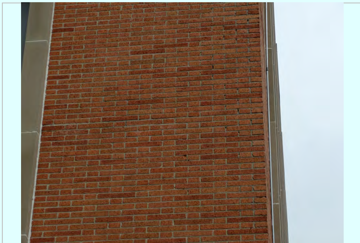
Photo: East Elevation, mortar joint deterioration
