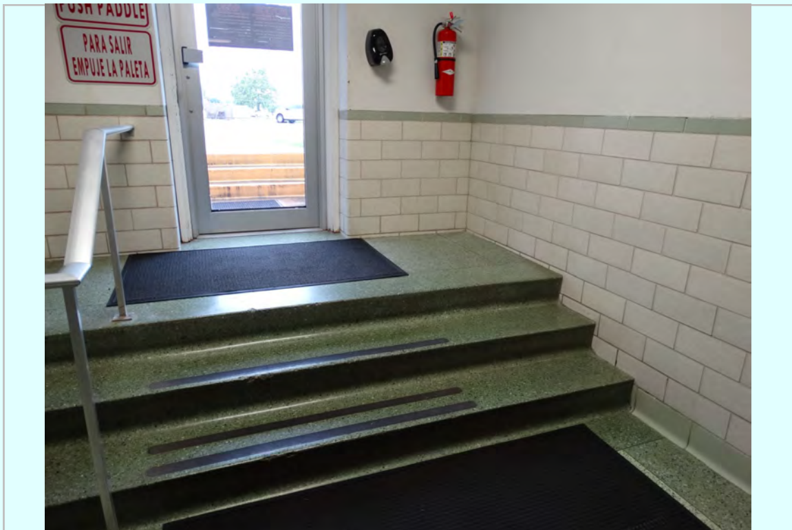
Photo: West door from the interior
