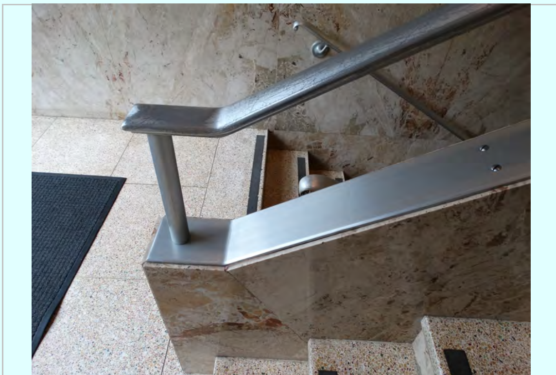
Photo: Typical handrail at central stair
