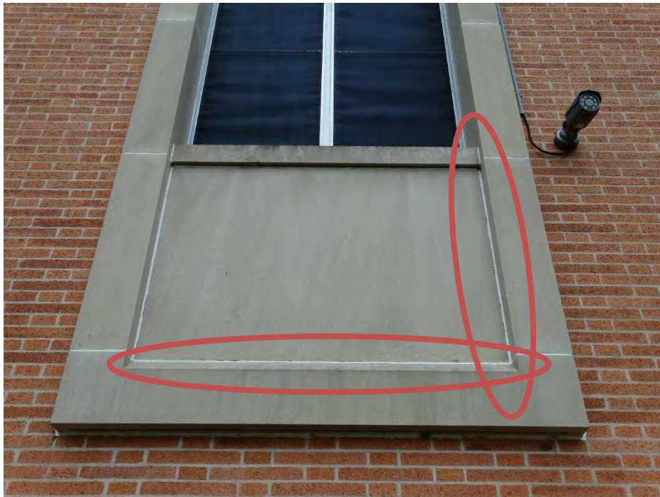
Figure 25. Limestone mortar replacement with non-compatible caulking, typical at all windows
