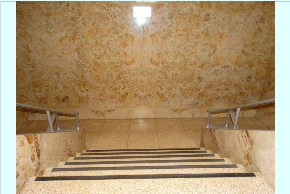
Photo: Typical stone condition at central stair
