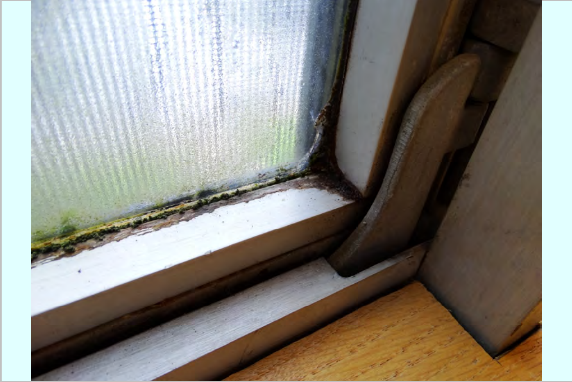
Photo: 3rd floor existing window condition
