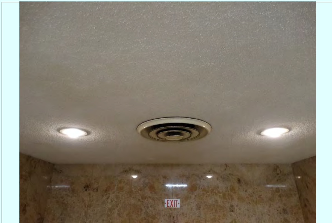
Photo: Third floor corridor moisture damage at ceiling and supply vent
