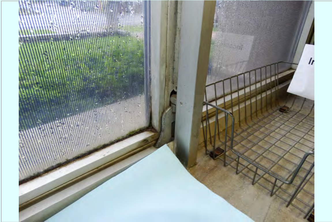
Photo: 2nd floor existing window operator
