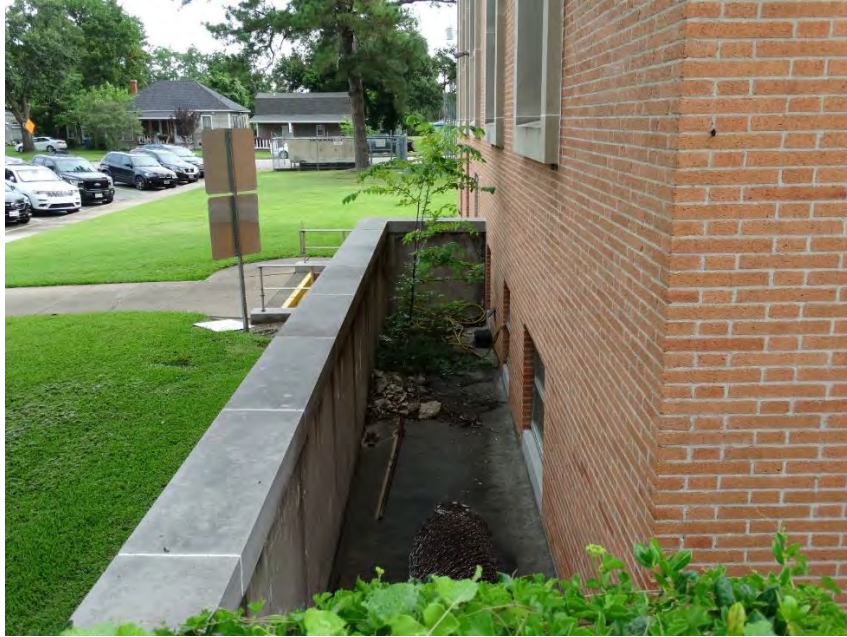
Figure 6. area well on west façade, showing wild planting and ponding of debris
