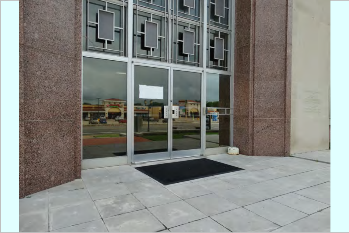
Photo: Original Curtain wall entry door
