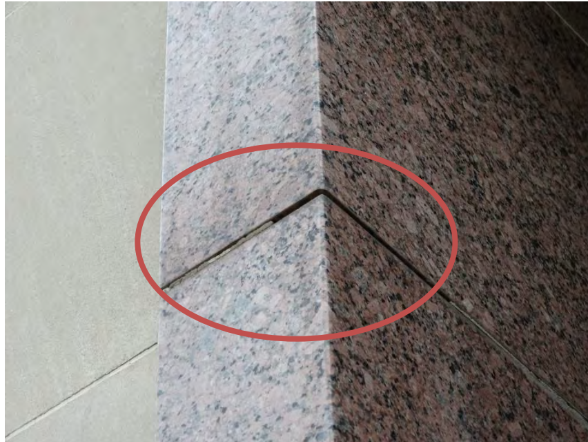
Figure 26. Typical mortar joint deterioration at north pink granite entry
