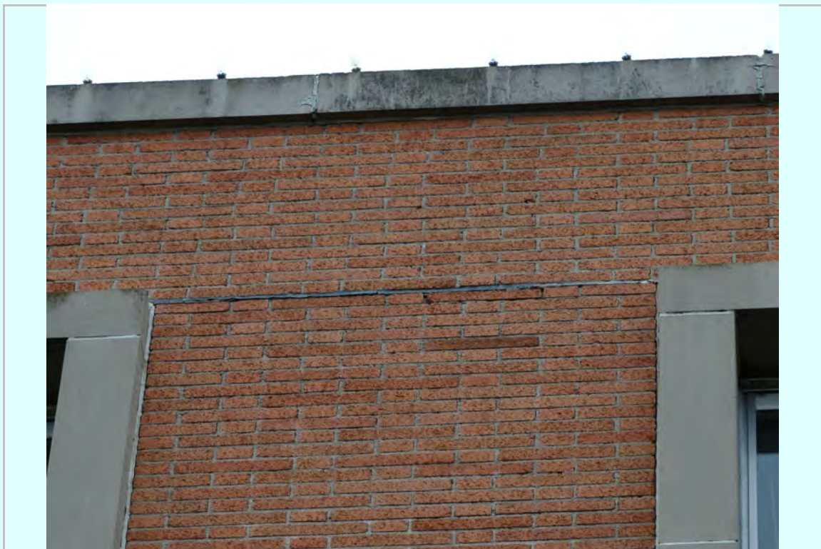
Photo: Deterioration, masonry joint and coping staining
