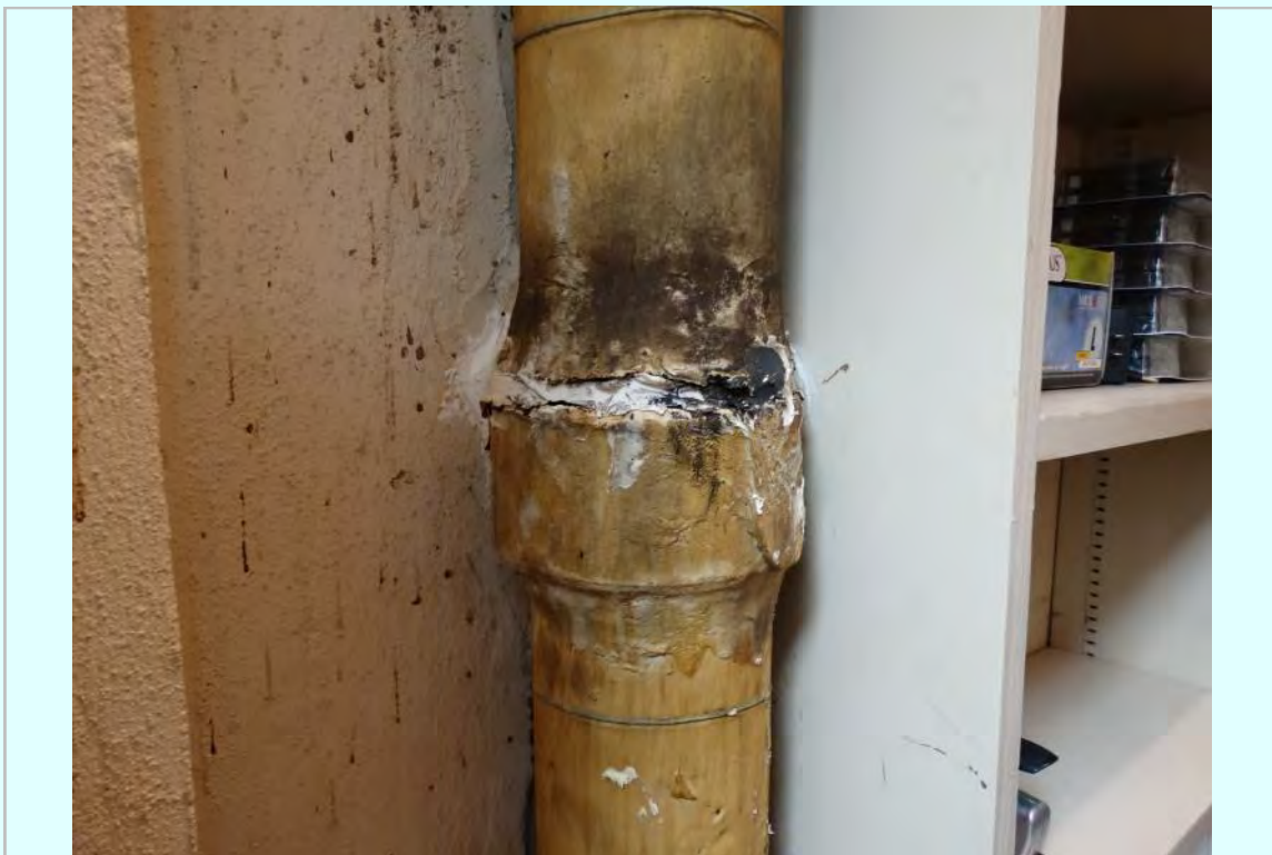
Photo: Third floor office space, internal roof drain damaged
