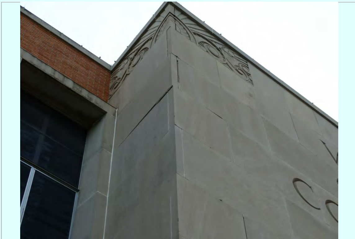
Photo: South Elevation, entry stone joints failing
