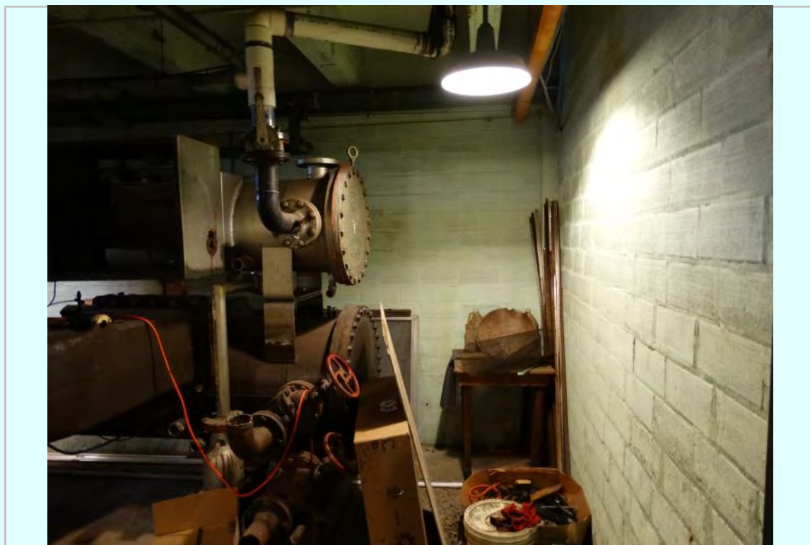
Photo: Fourth floor, mechanical space
