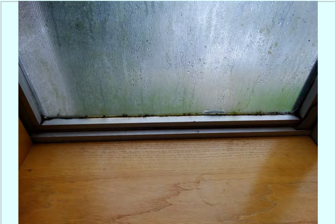
Photo: 3rd floor existing window at stool
