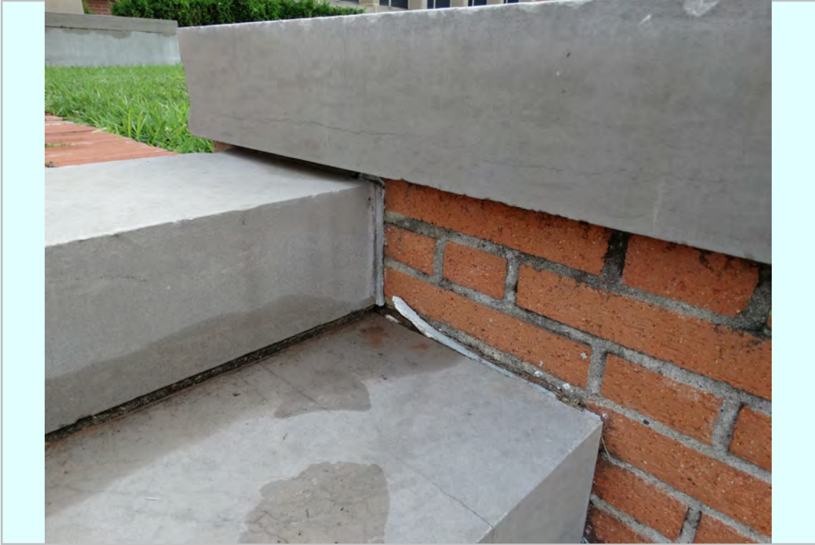
Photo: South entry retaining walls at stair juncture failing
