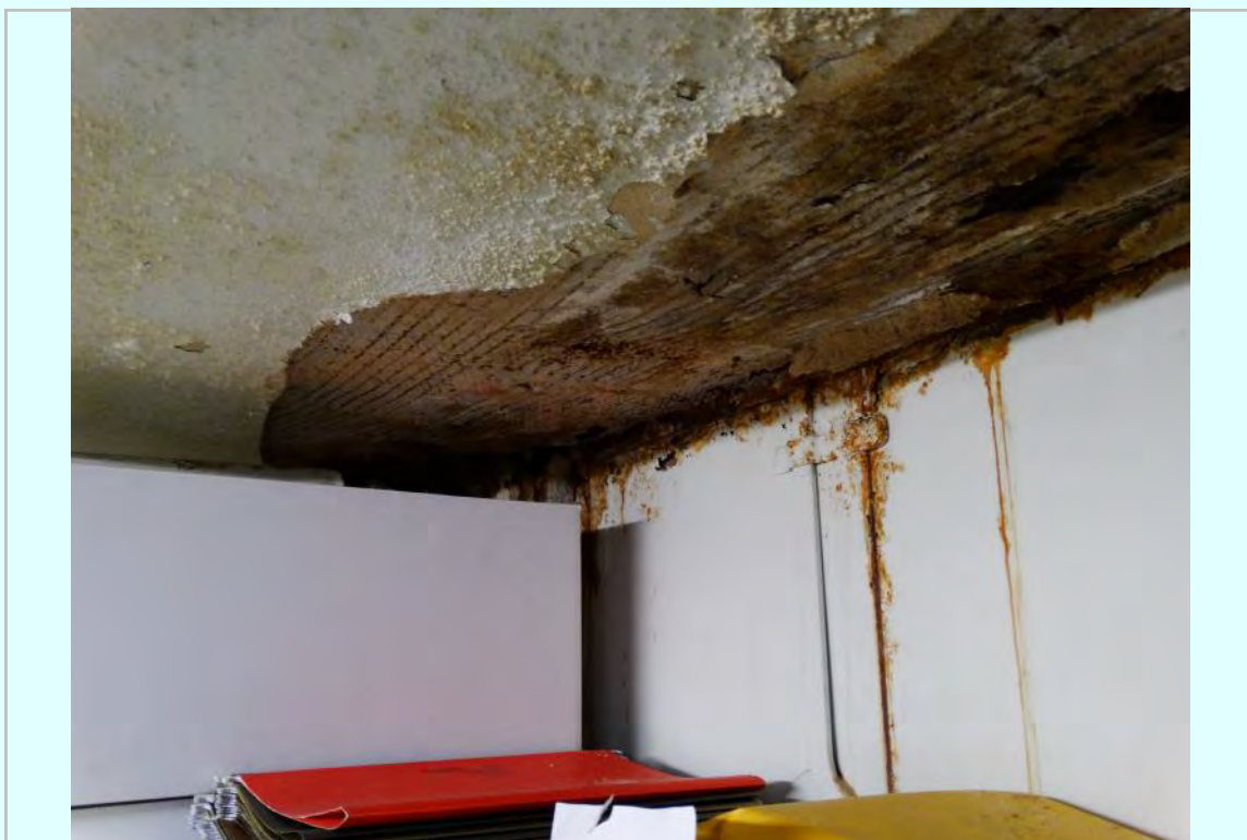
Photo: Extreme moisture damage at ceiling in storage space below County Auditor
