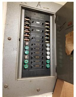
The building is served by three, overhead services at 120/240 volts, 1 phase, 3 wire. The electrical system, in most cases, consists of original panelboards, wiring and receptacles. Several panels utilize Edison base fuses and disconnect switches.
