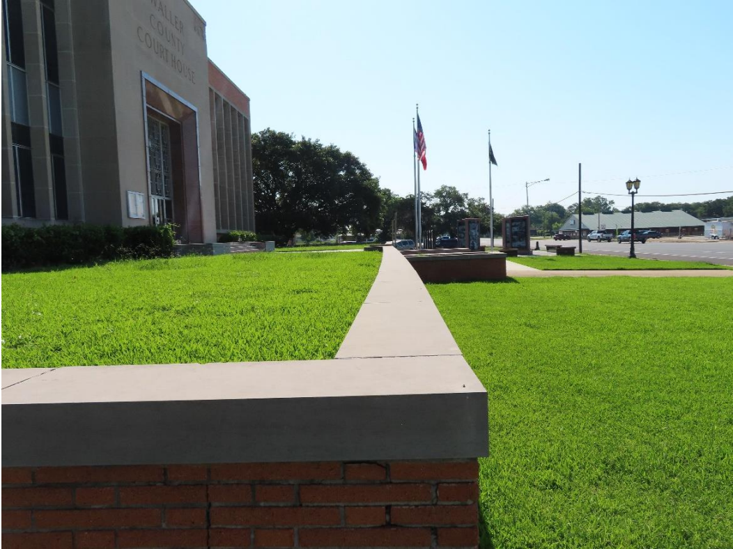
Photograph 10 – Retaining wall displacement on the south site wall.
