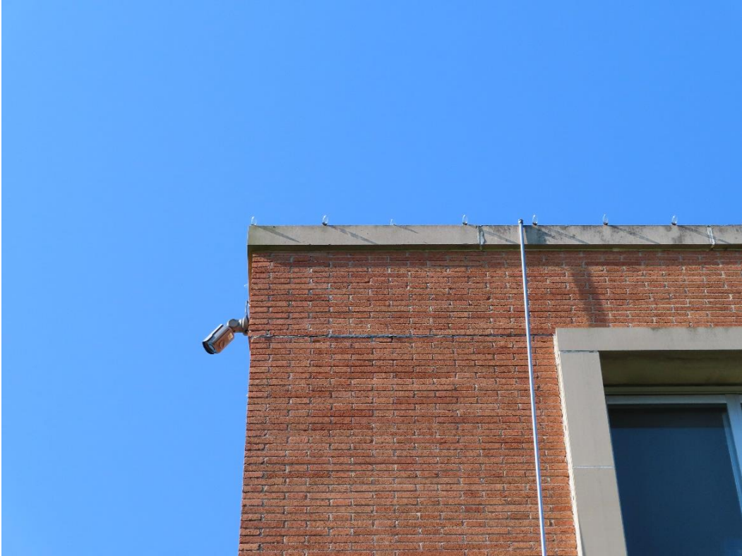
Photograph 8 – Parapet displacement in the brick veneer.
