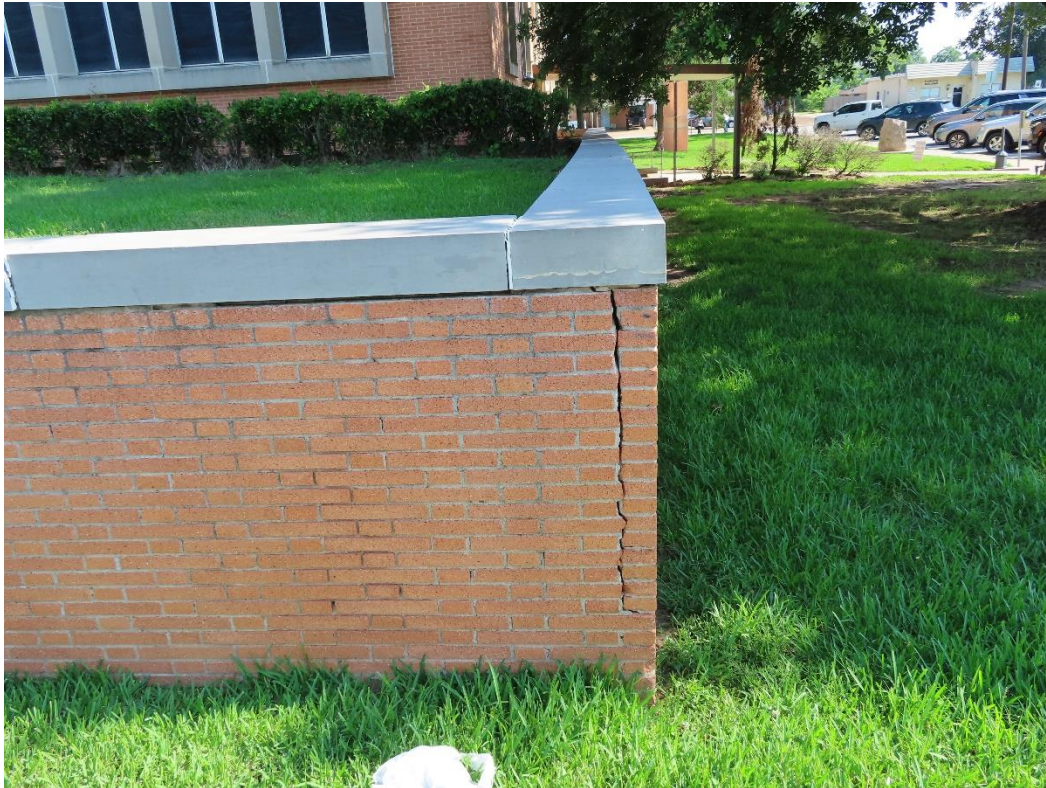
Photograph 13 – Damage retaining wall brick veneer southeast site wall corner.
