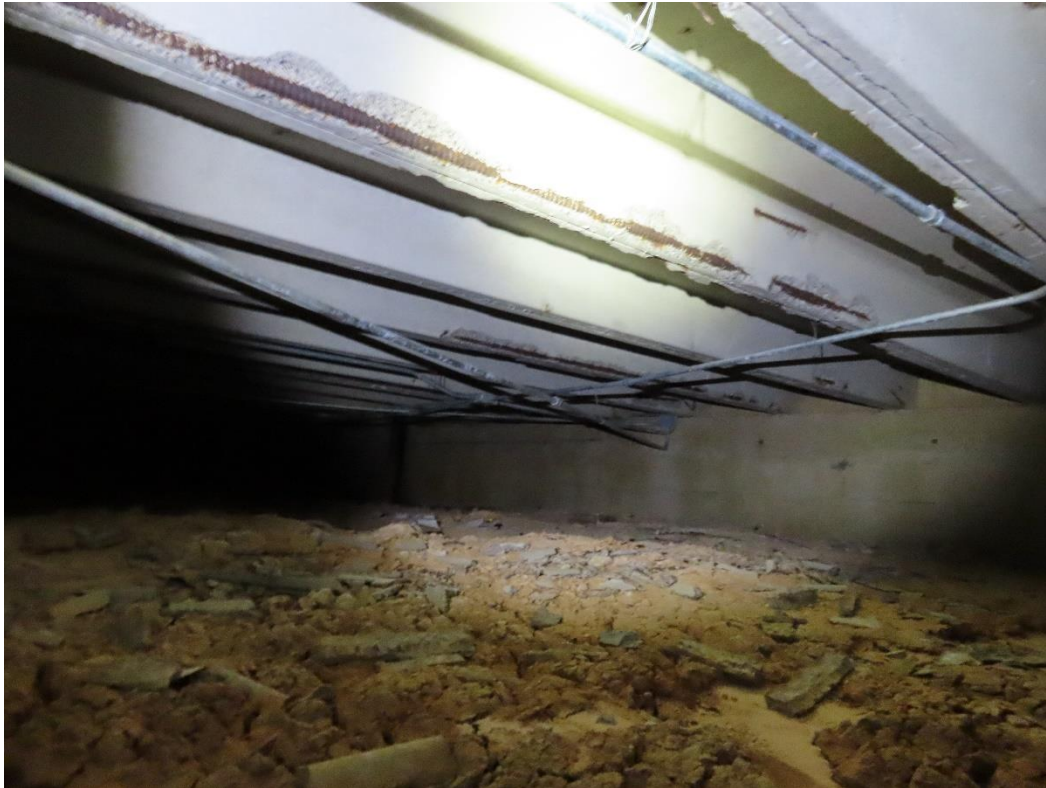
Photograph 3 – Reinforcing steel corrosion in the crawlspace.
