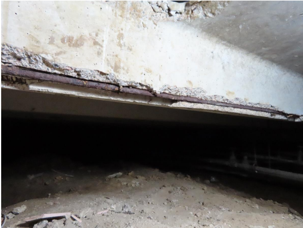
Photograph 17 – Reinforcing steel corrosion in the crawlspace.
