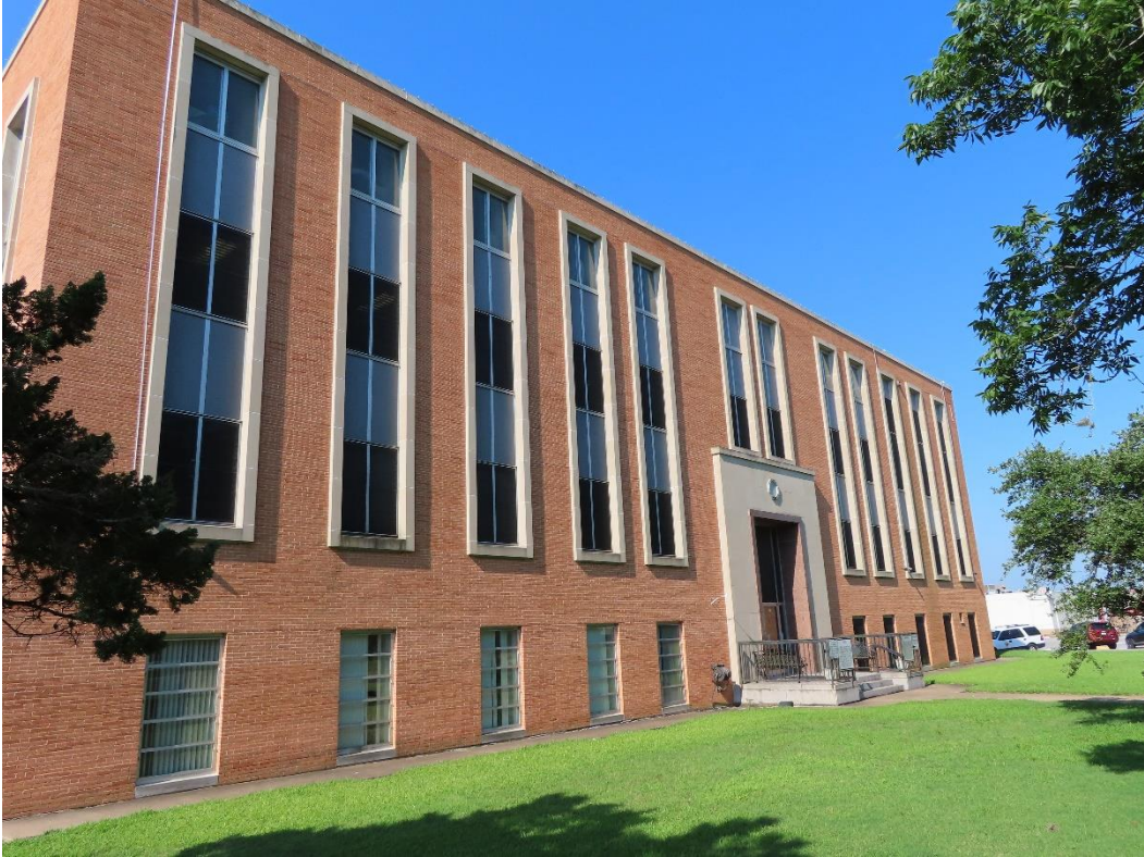
Photograph 7 – North façade elevation.
