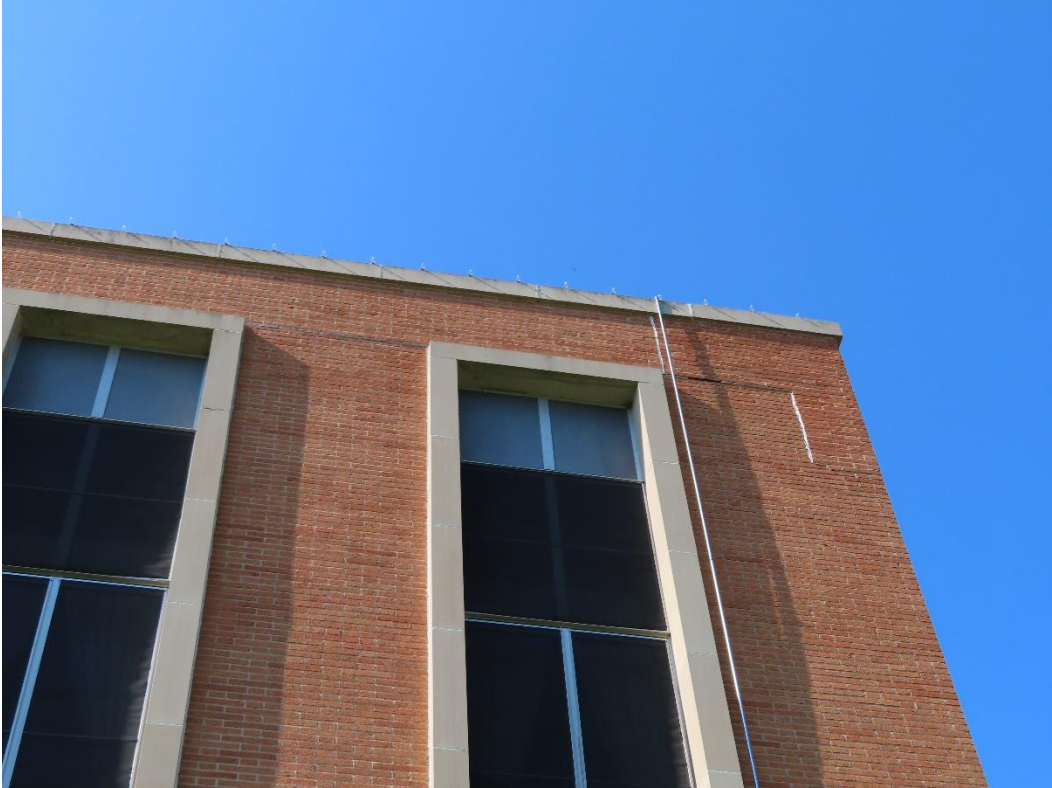
Photograph 9 – Parapet displacement in the brick veneer.
