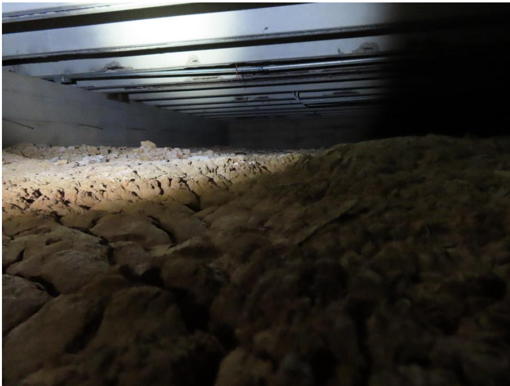
Photograph 4 – Reinforcing steel corrosion in the crawlspace.
