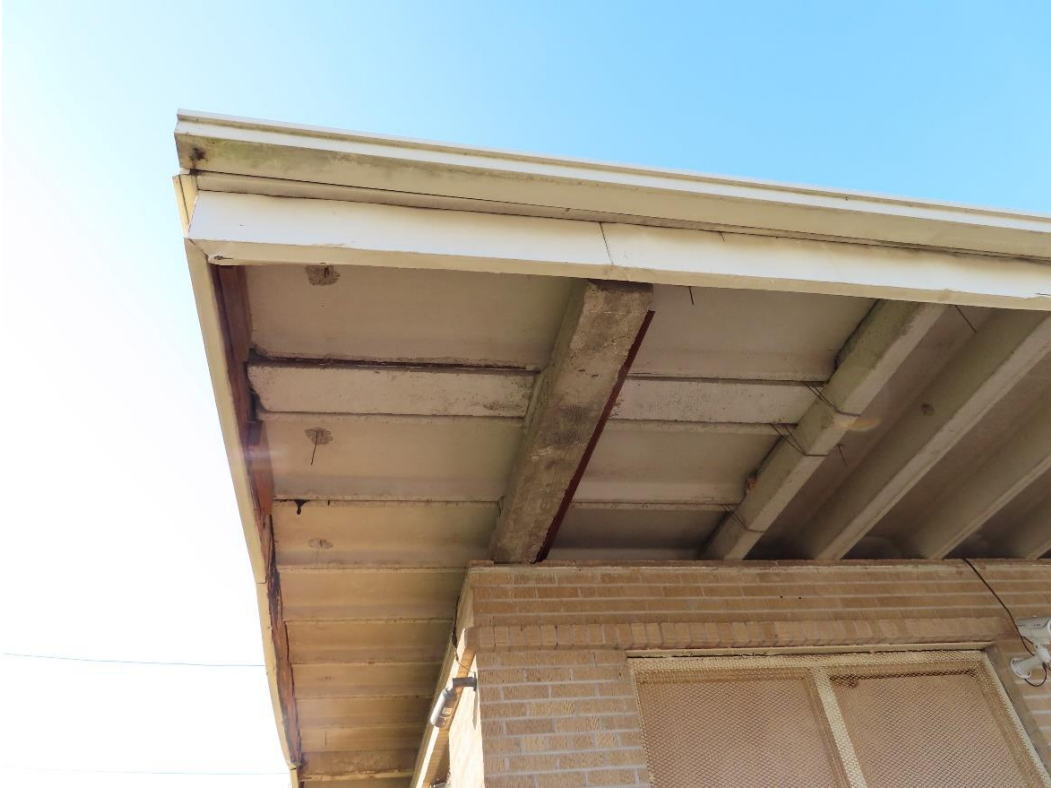
Photograph 22 – Exposed roof overhang structure and corroded reinforcing steel.
