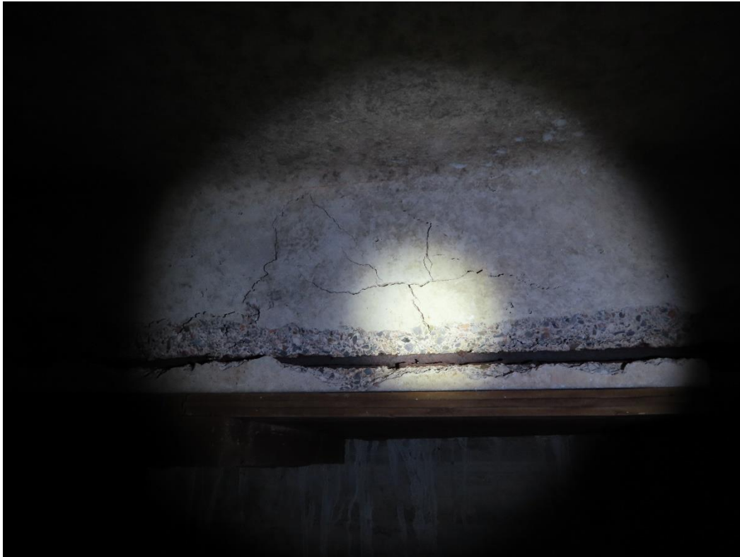
Photograph 19 – Deteriorated concrete and reinforcing steel corrosion in the crawlspace.
