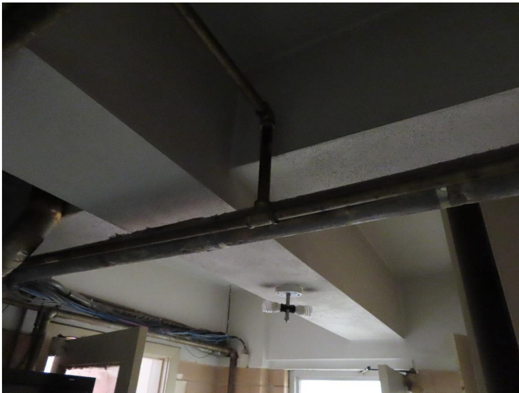
Photograph 16 – Exposed concrete structure.
