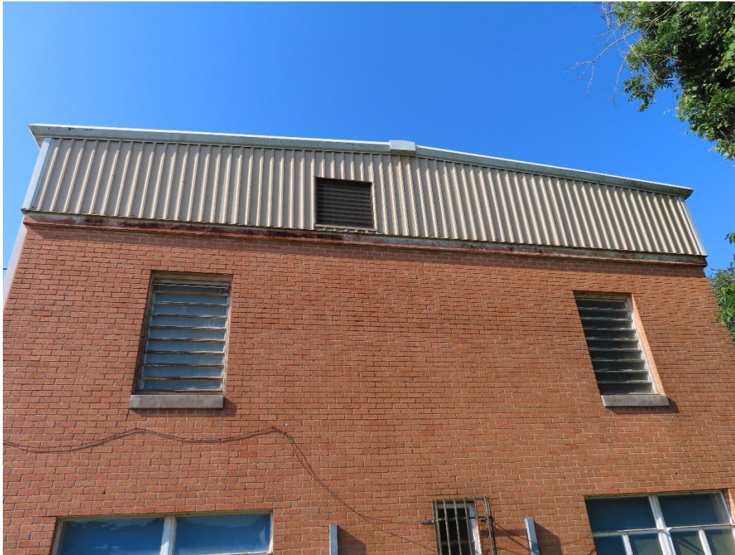
Photograph 15 – North façade of the Jail Building.
