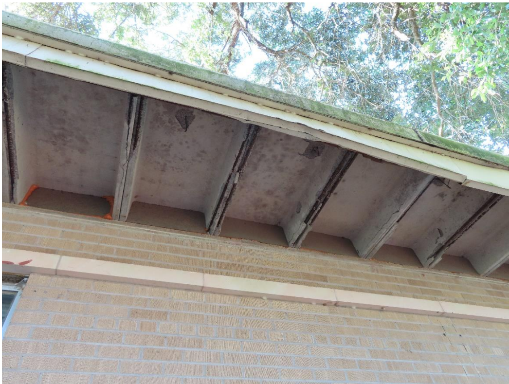
Photograph 24 – Exposed roof overhang structure and corroded reinforcing steel.
