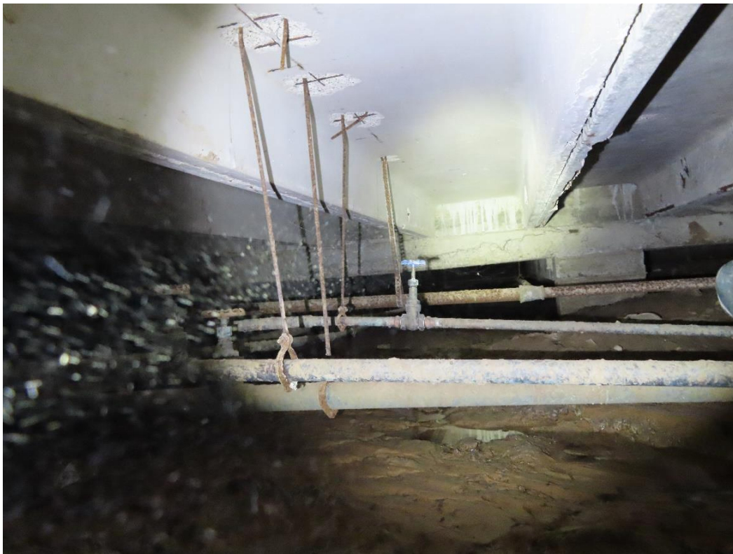
Photograph 18 – Deteriorated concrete and reinforcing steel corrosion in the crawlspace.
