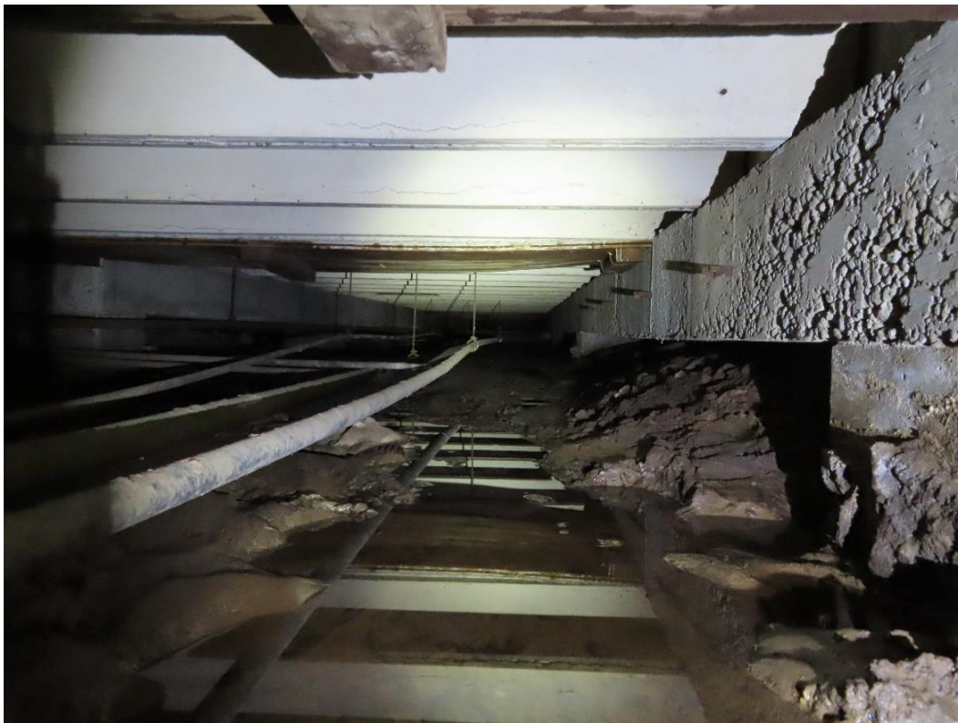
Photograph 20 – Deteriorated concrete and reinforcing steel corrosion in the crawlspace.
