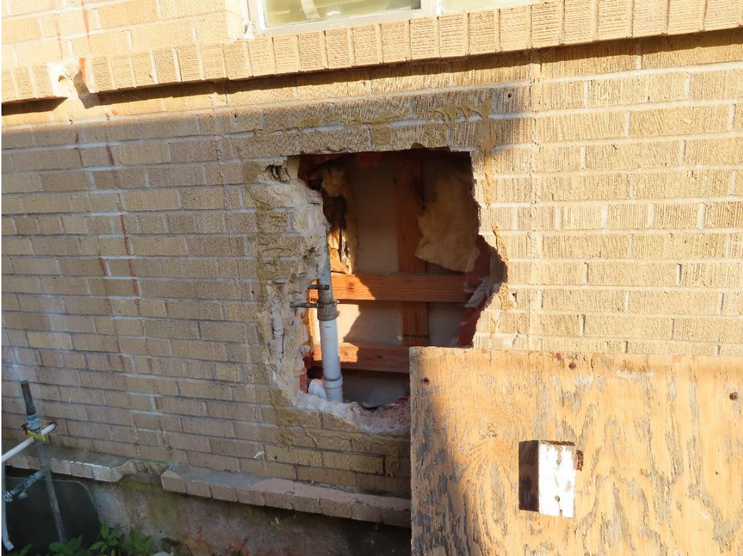
Photograph 26 – Impact damage in the exterior load-bearing wall.
