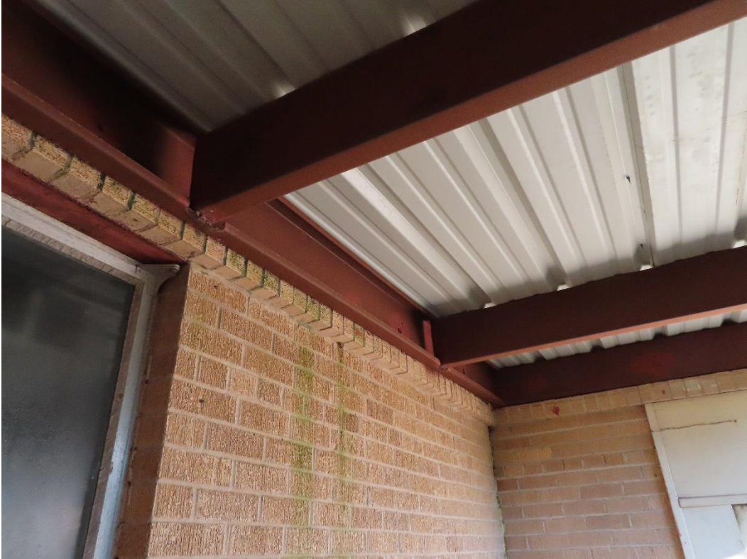
Photograph 25 – Metal canopy supported by the brick veneer.
