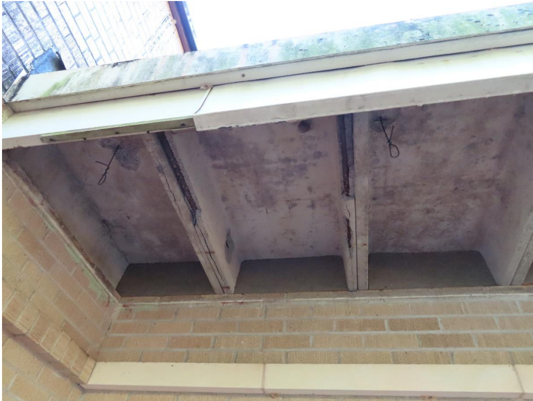
Photograph 23 – Reinforcing steel corrosion in the soffit.
