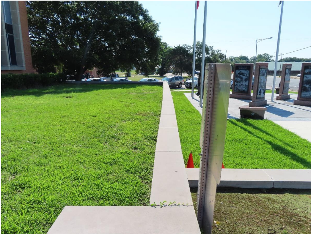
Photograph 11 – Retaining wall displacement at the south site wall.
