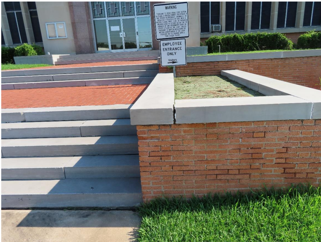
Photograph 12 – Retaining wall displacement on the south site wall.
