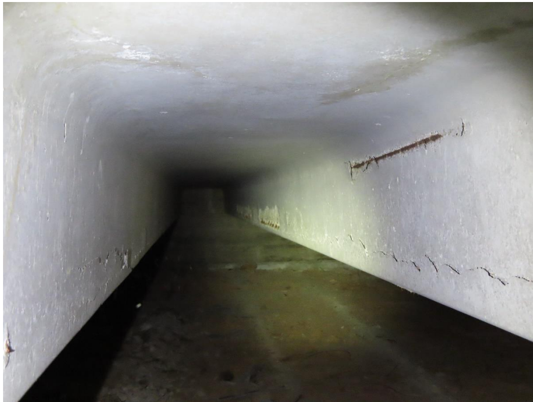
Photograph 5 – Reinforcing steel corrosion in the crawlspace.
